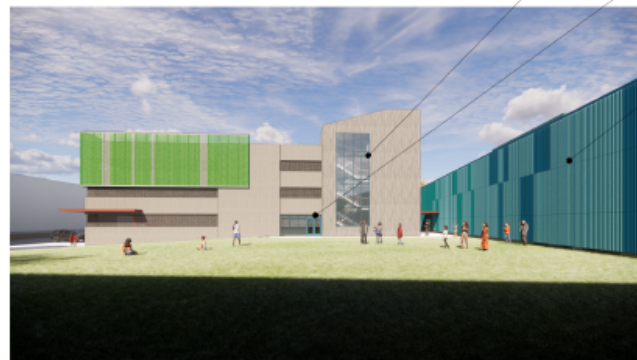
2 - EAST ELEVATION OF GARAGE
