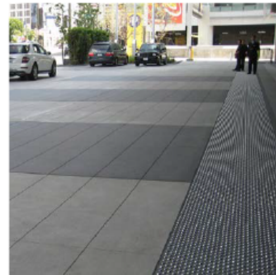
■■■■ TRUNCATED DOMES FOR ADA CROSSING
