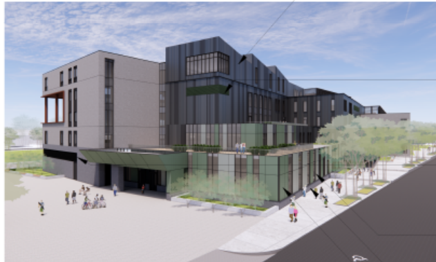
1 - VIEW TO MAIN ENTRANCE FROM SOUTHEAST CORNER
