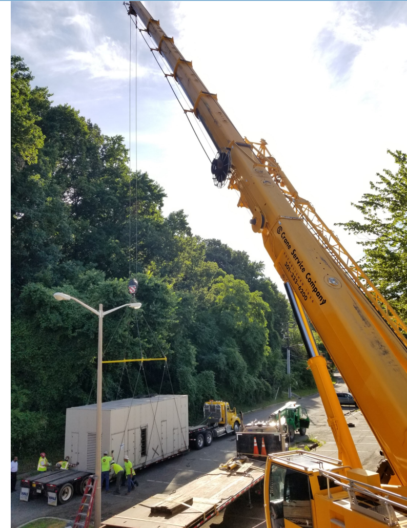
HVAC Replacement at Gunston (July 2019)
