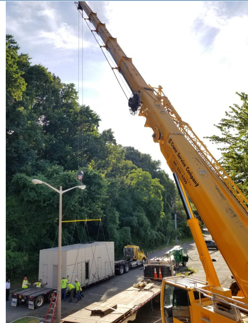
HVAC Replacement at Gunston (July 2019)
