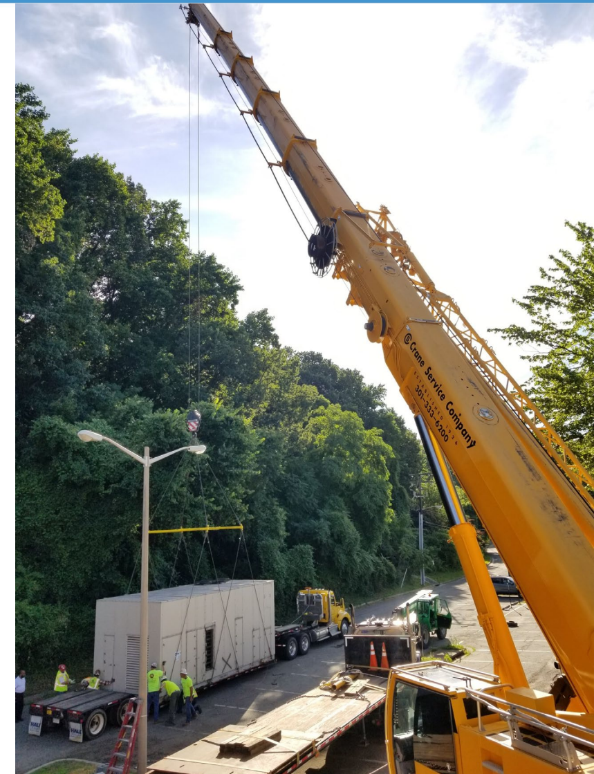
HVAC Replacement at Gunston (July 2019)
