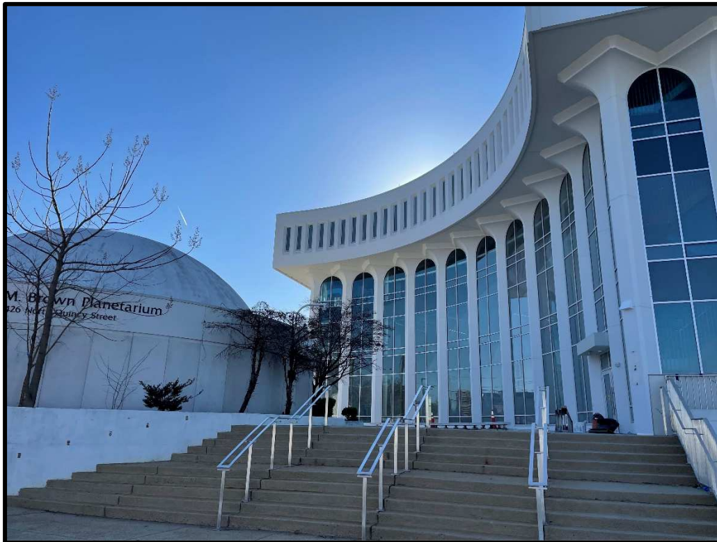
View of the Front of the Building
