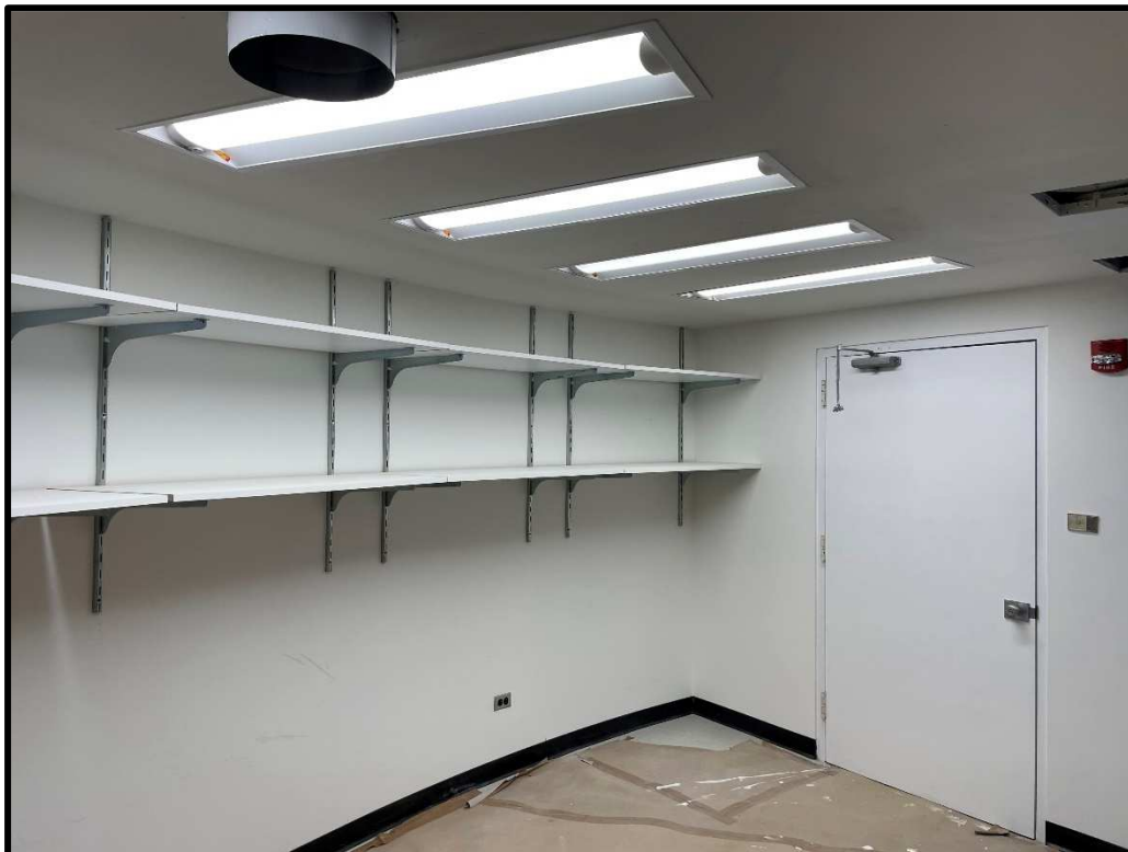
View of Work in Progress at Storage Room
