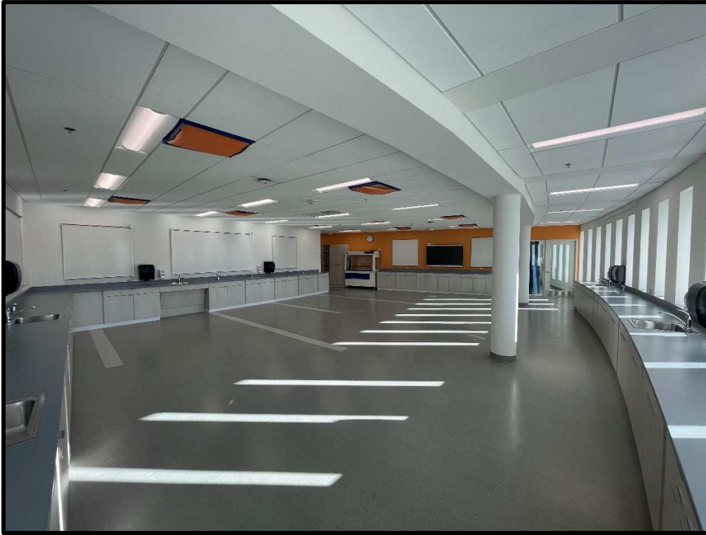
View of Work Ongoing on Level 4
