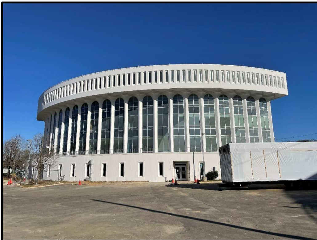
View of the Rear of the Building
