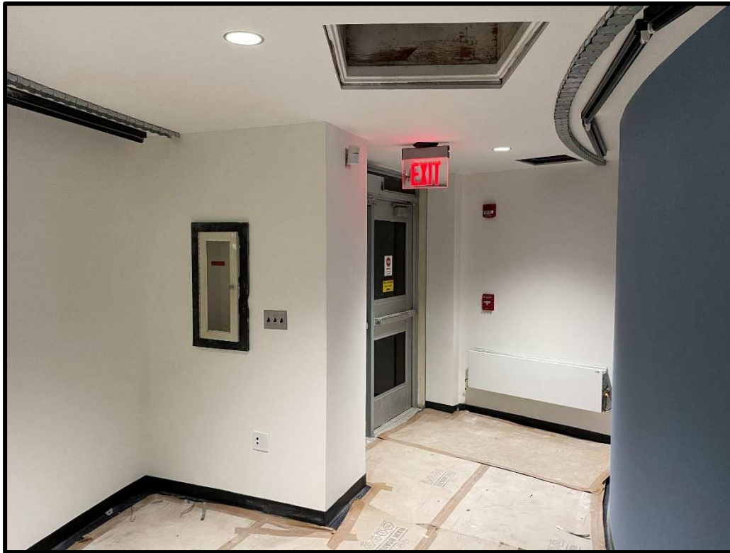
View of Work in Progress at Planetarium Corridor
