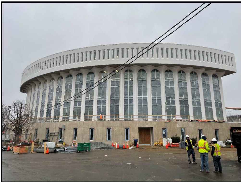
View of the Rear of the Building
