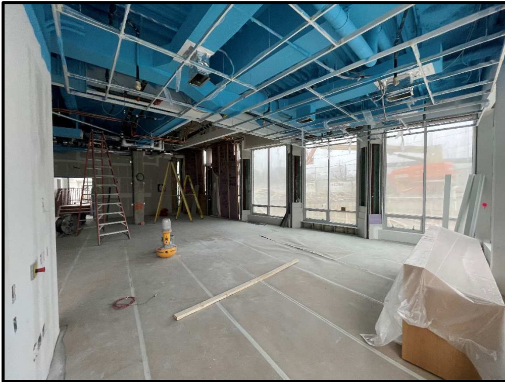
View of Work in Progress at New Front Office
