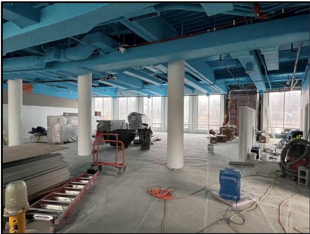
View of Work Ongoing on Level 1
