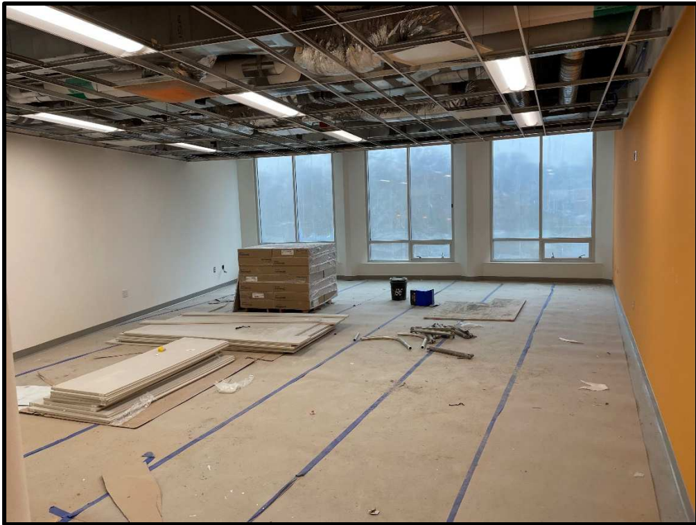
View of Work Ongoing on Level 2
