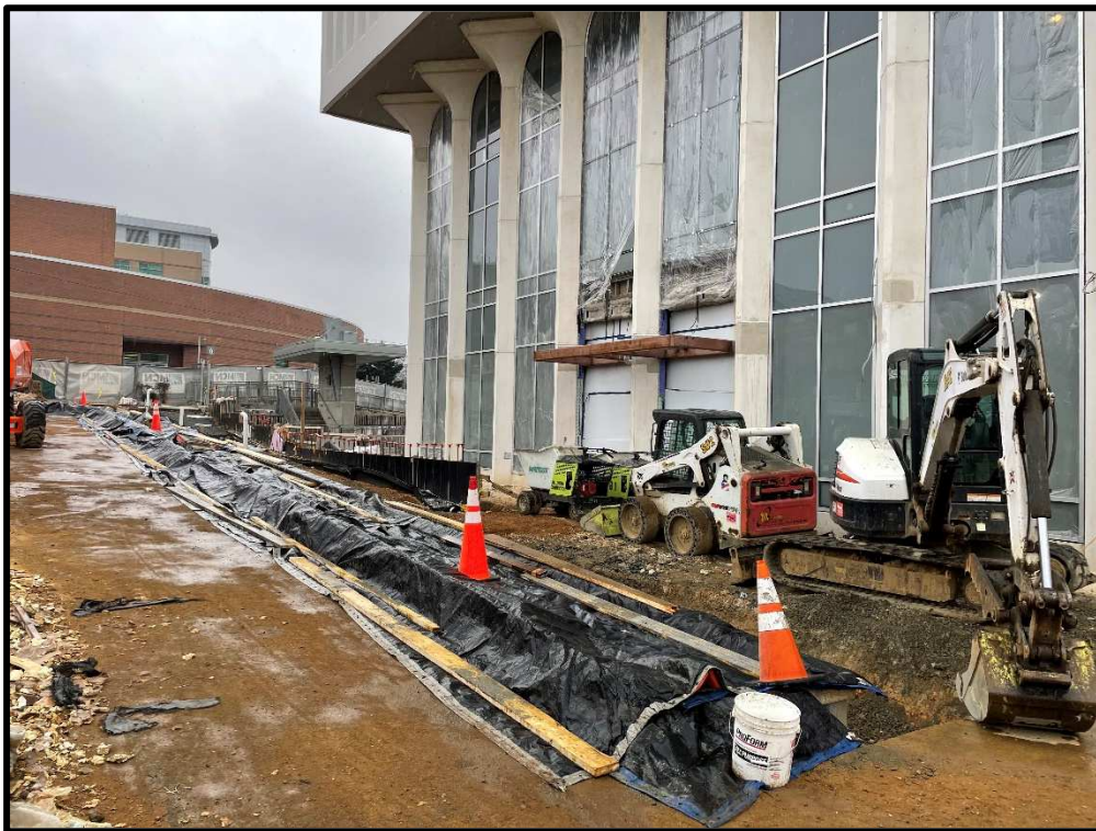
View of Work Ongoing on Main Ramp
