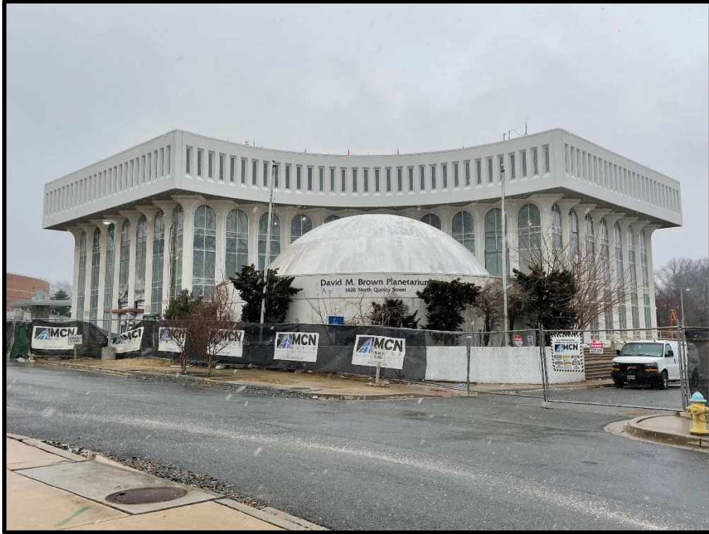
View of the Front of the Building
