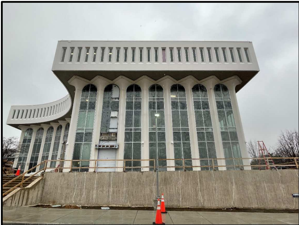
View of Exterior on East Side of Building
