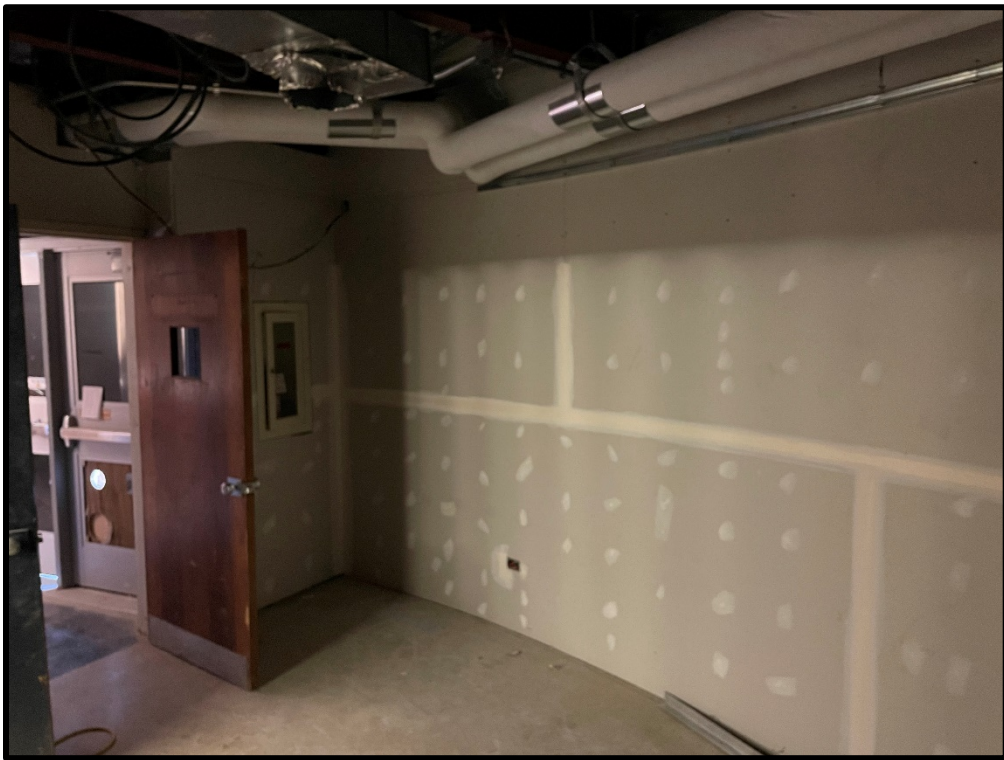
View of Work Ongoing Planetarium
