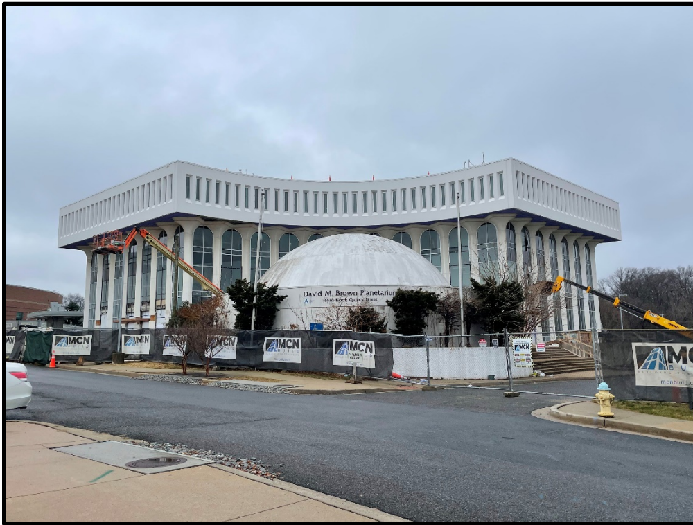
View of the Front of the Building
