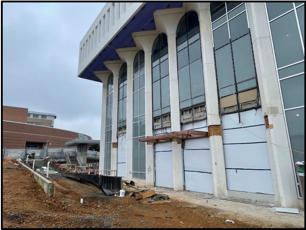
View of Work Ongoing on Main Ramp
