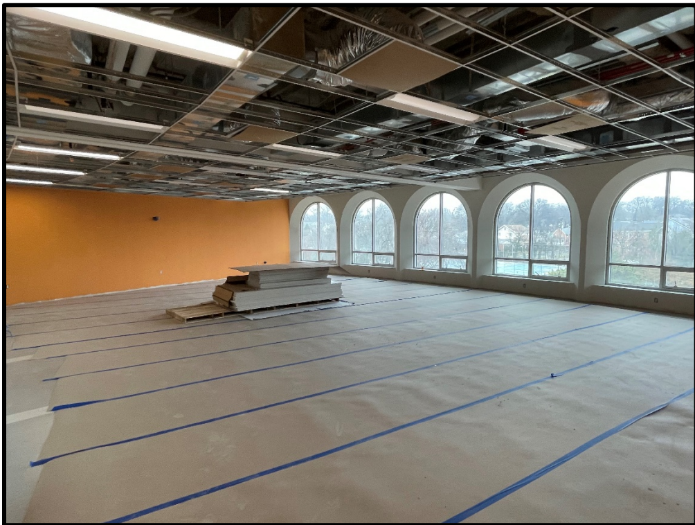
View of Work Ongoing on Level 3
