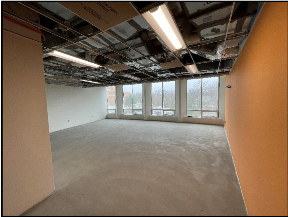
View of Work Ongoing on Level 2
