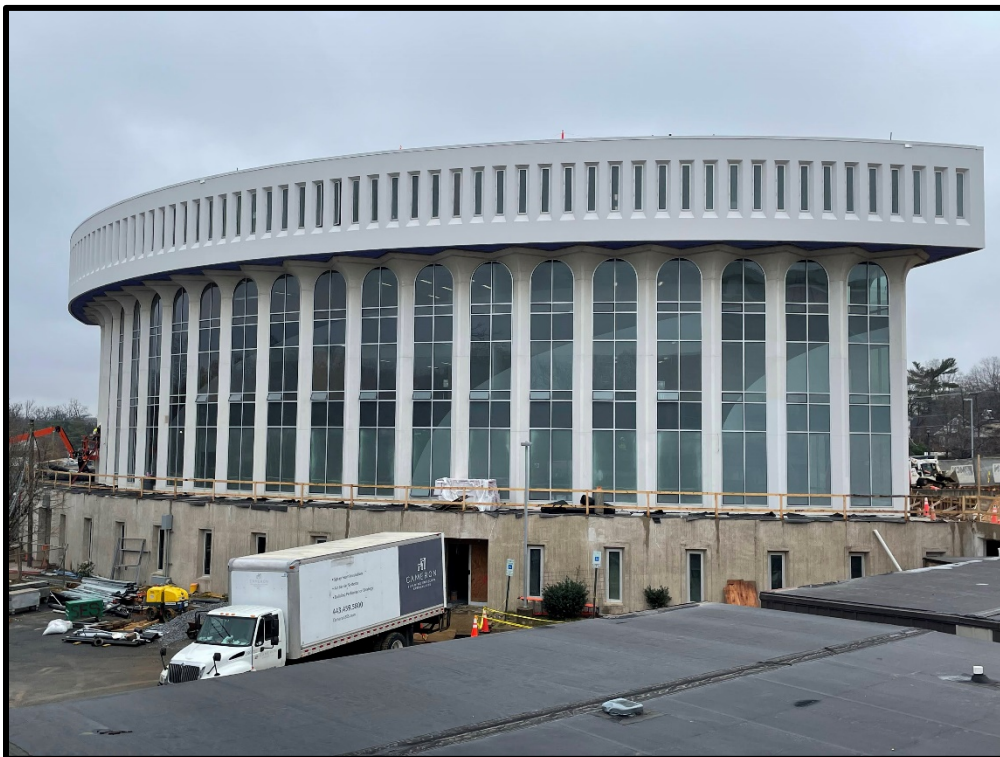
View of the Rear of the Building
