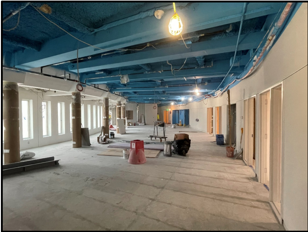
View of Work Ongoing on Level 4
