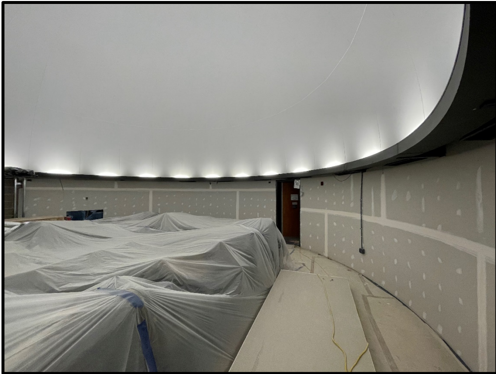
View of Work Ongoing Planetarium
