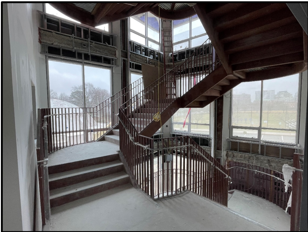
View of Stair A
