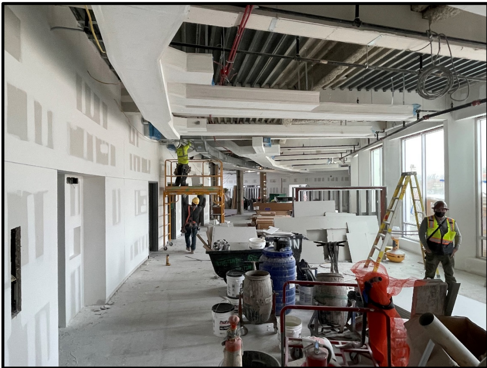
View of Work Ongoing on Level 1
