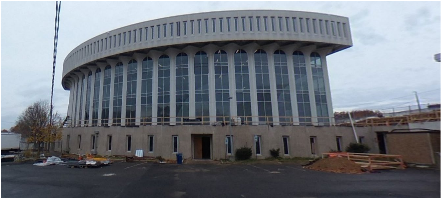
View of the Rear of the Building
