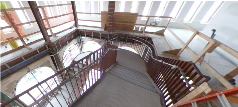
View of Stair A
