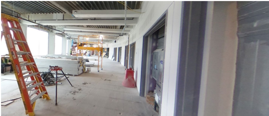
View of Work Ongoing on Level 2
