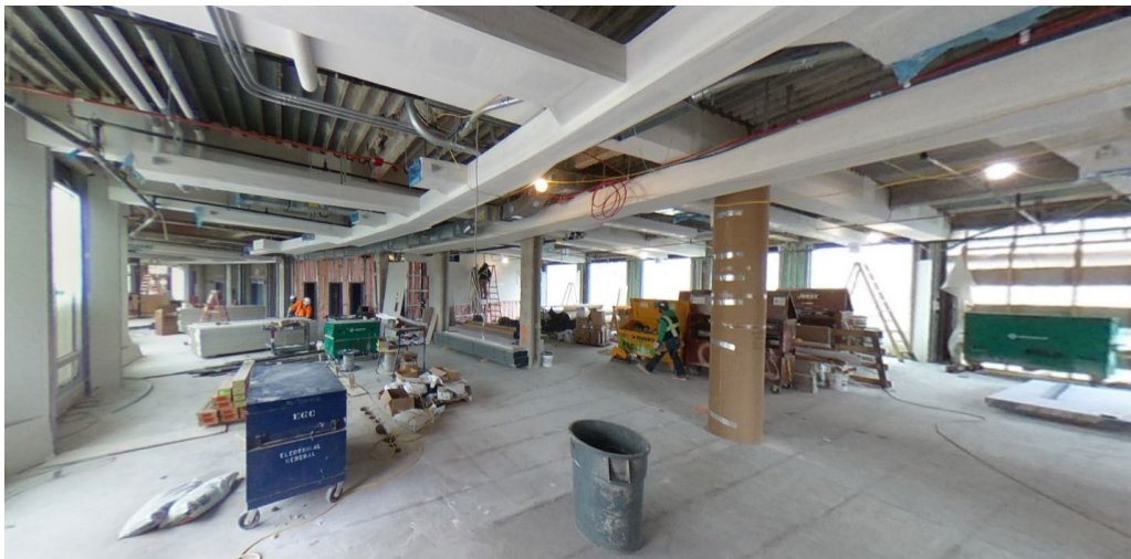
View of Work Ongoing on Level 1
