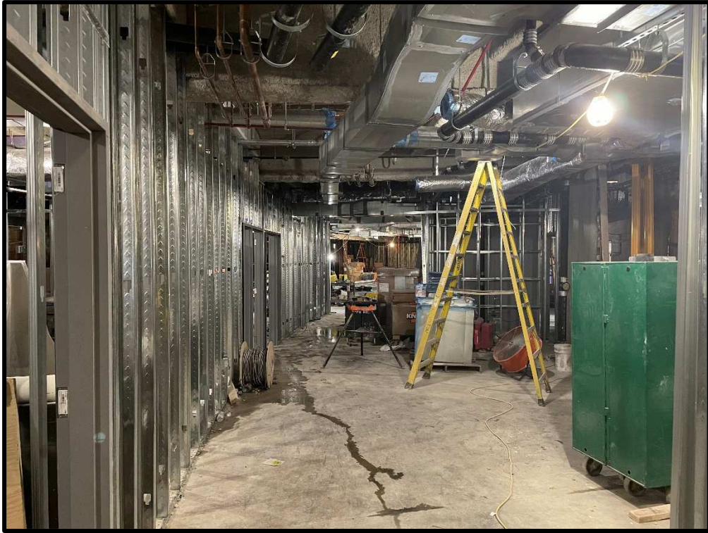
View of Work Ongoing on the Ground Floor
