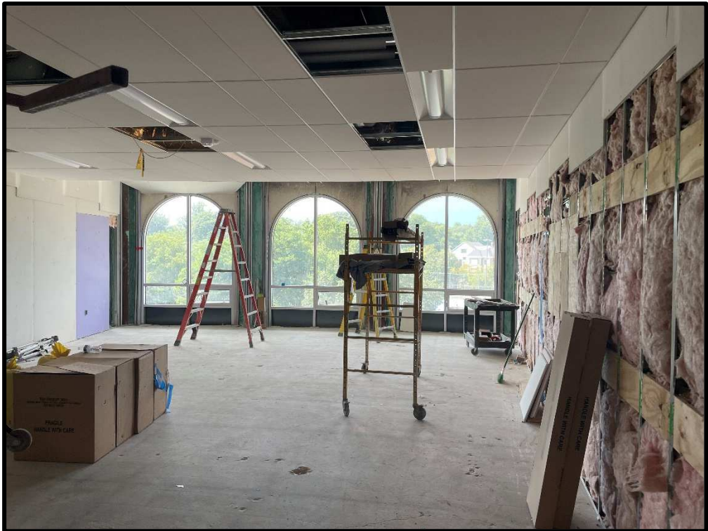
View of Work Ongoing on Level 3
