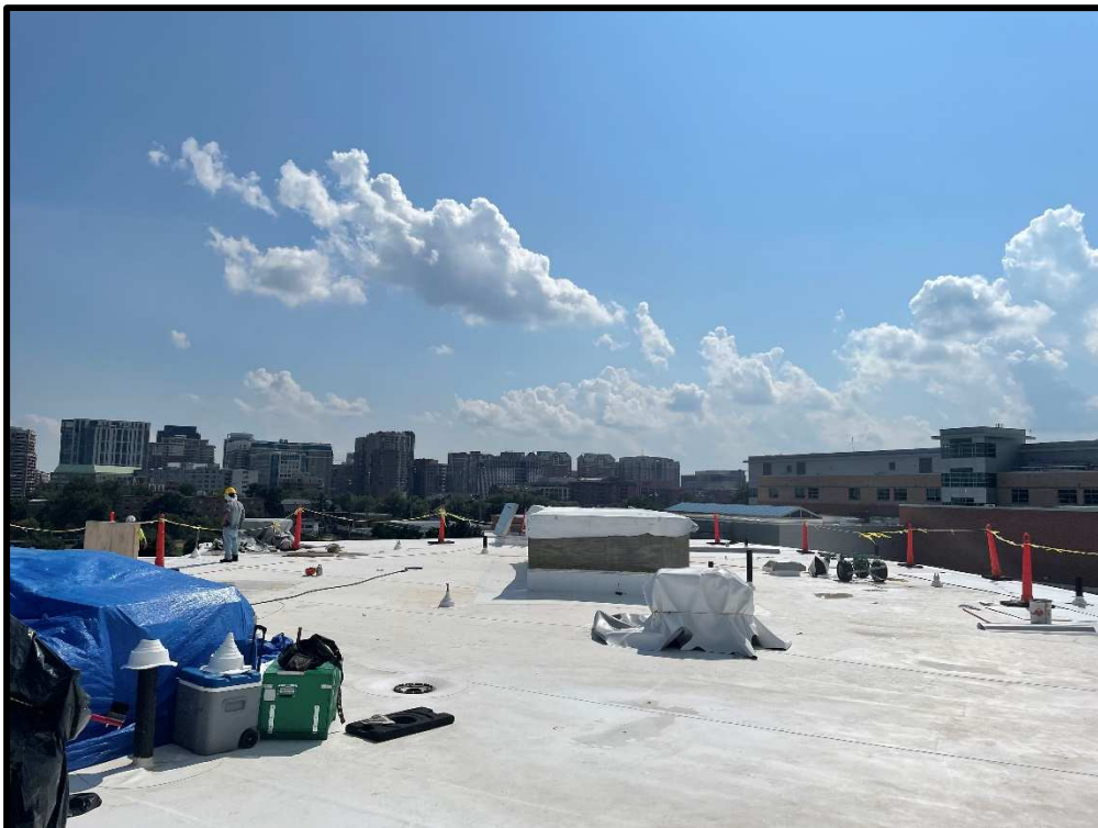
View of Working Ongoing on Roof
