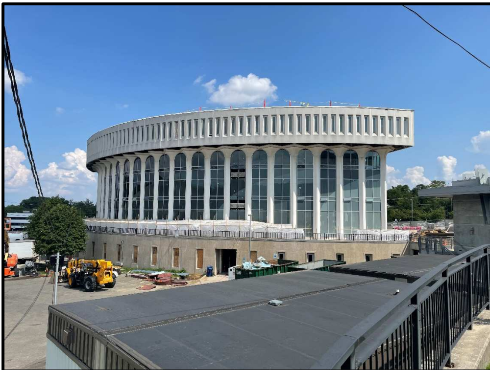
View of the Rear of the Building
