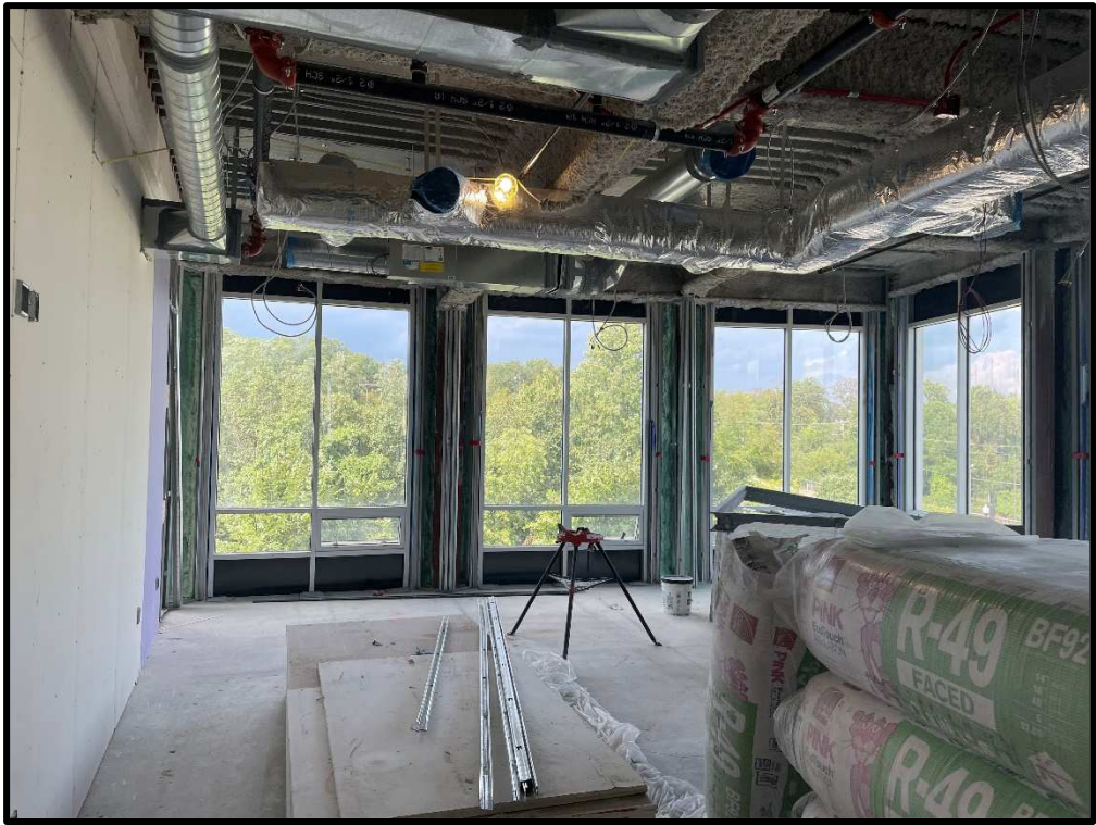
View of Work Ongoing on Level 2
