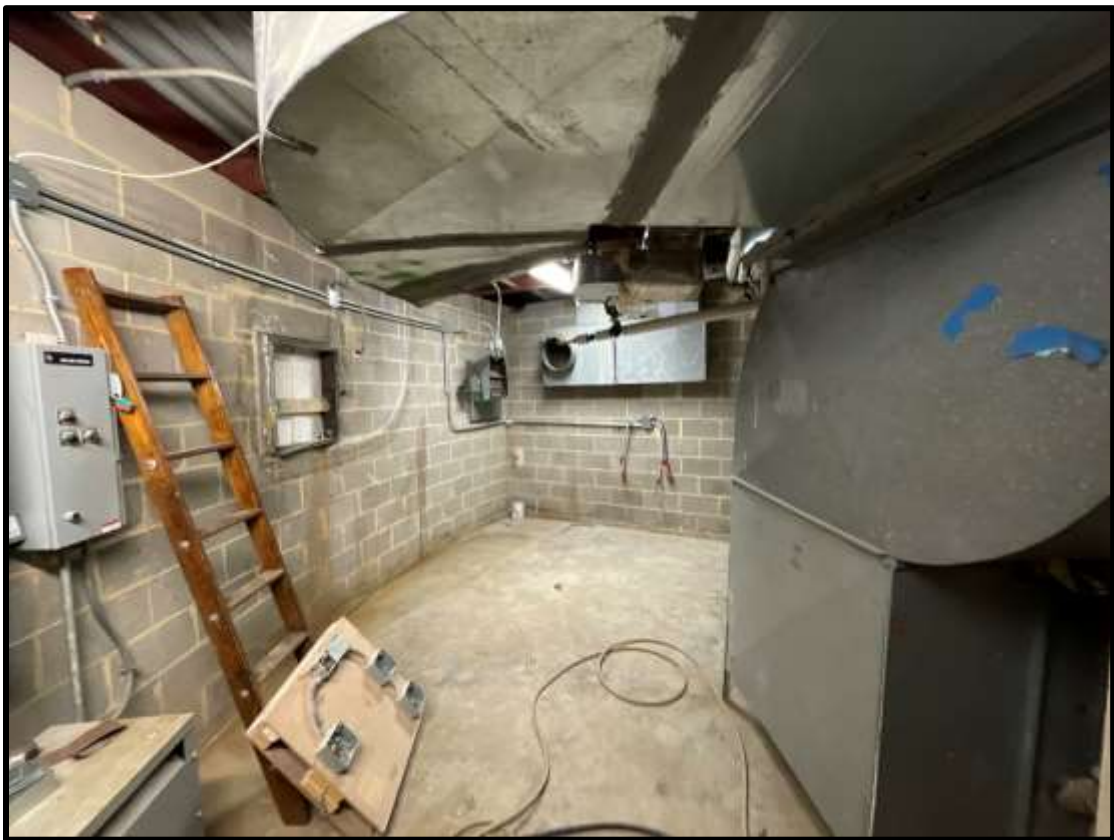
View of Working Ongoing in Planetarium
