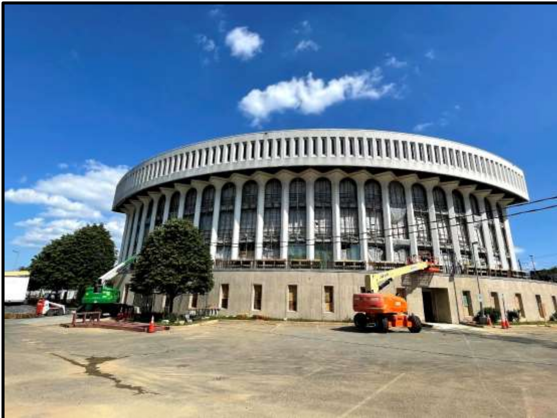
View of the Rear of the Building
