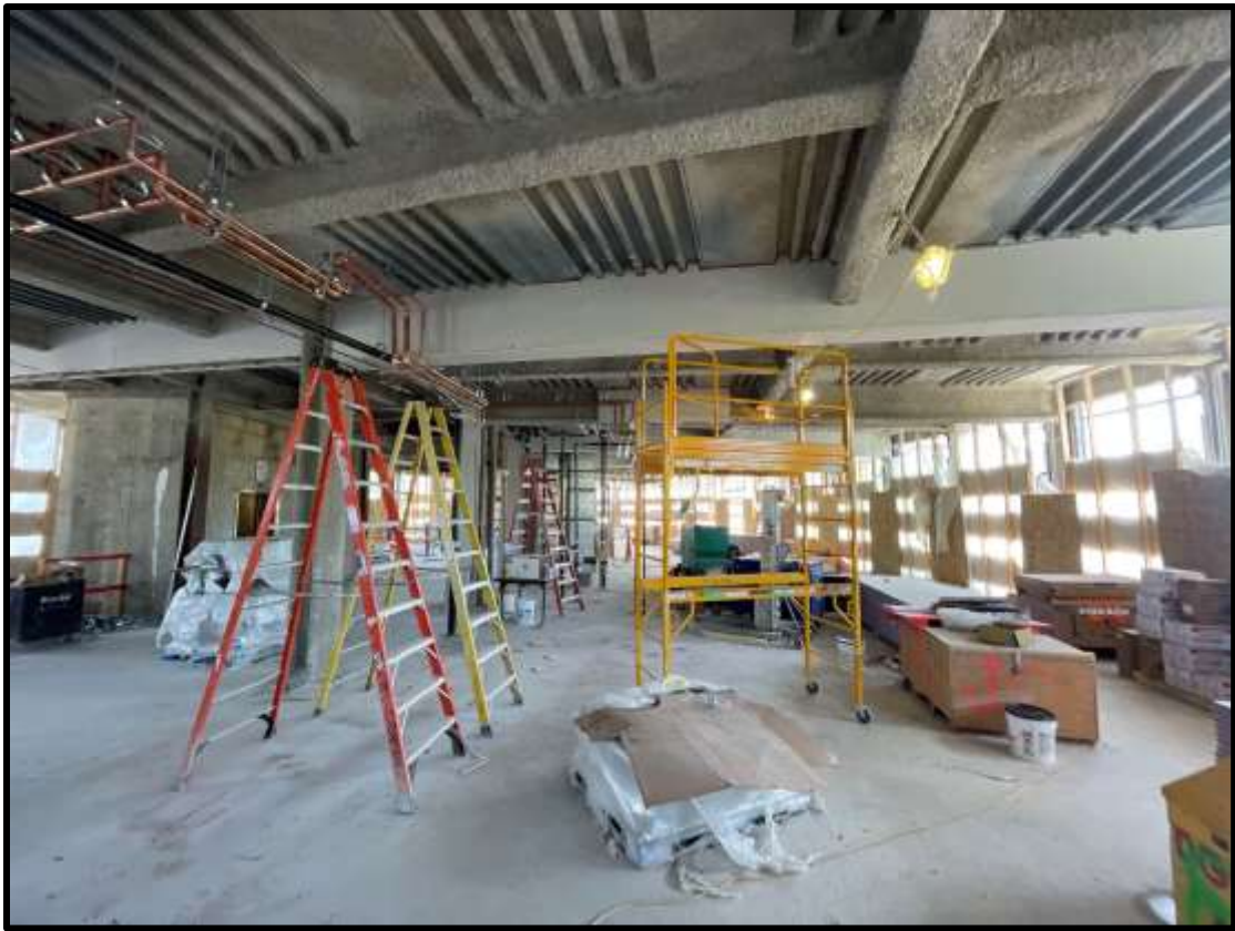
View of Work Ongoing on Level 1
