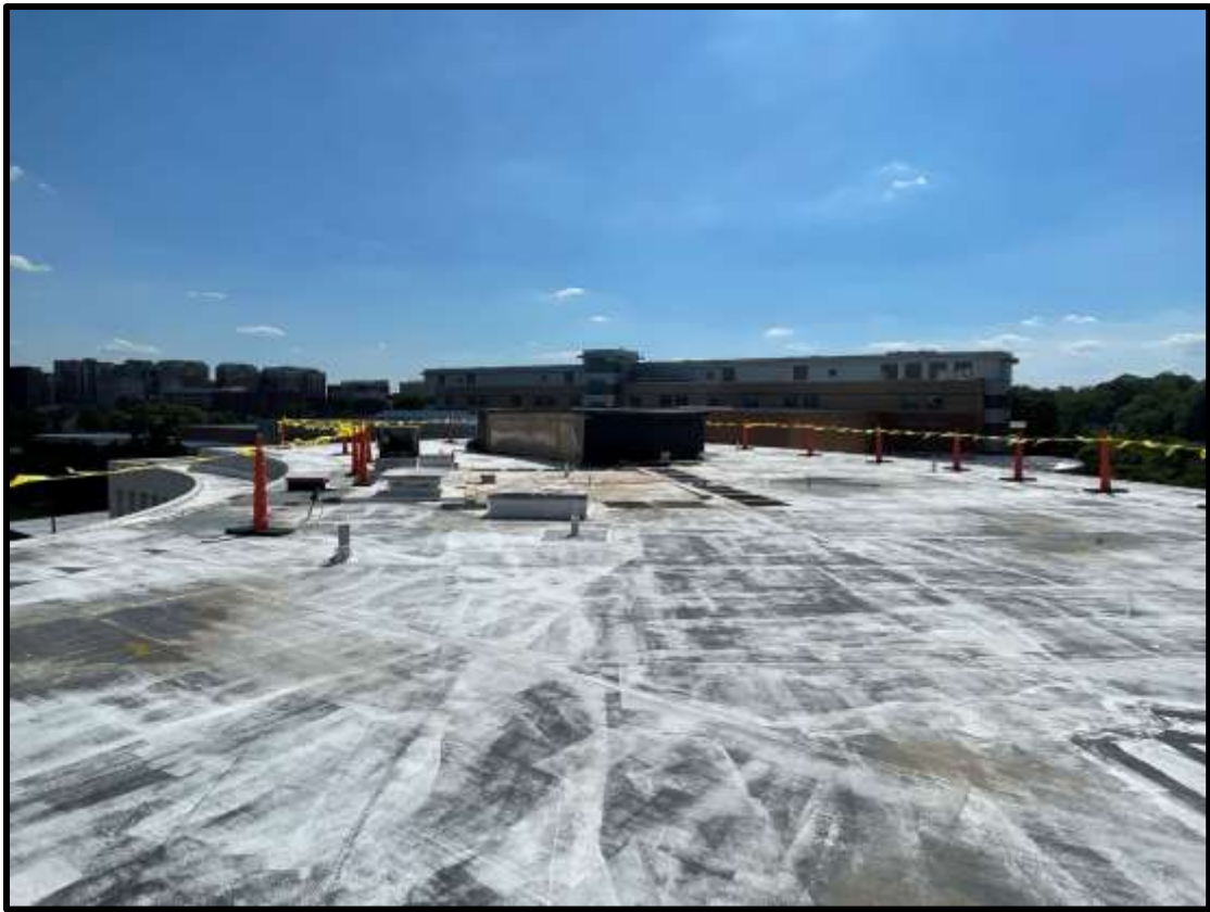
View of Working Ongoing on Roof
