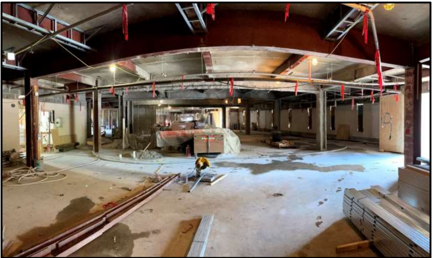
View of Work Ongoing on the Ground Floor
