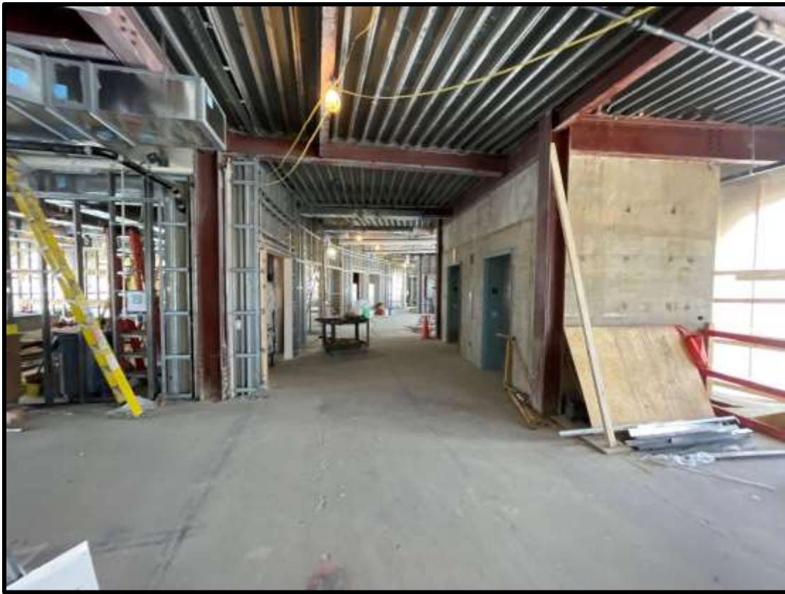
View of Work Ongoing on Level 3
