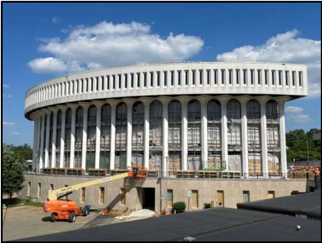
View of Rear of Building from Washington Liberty High School
