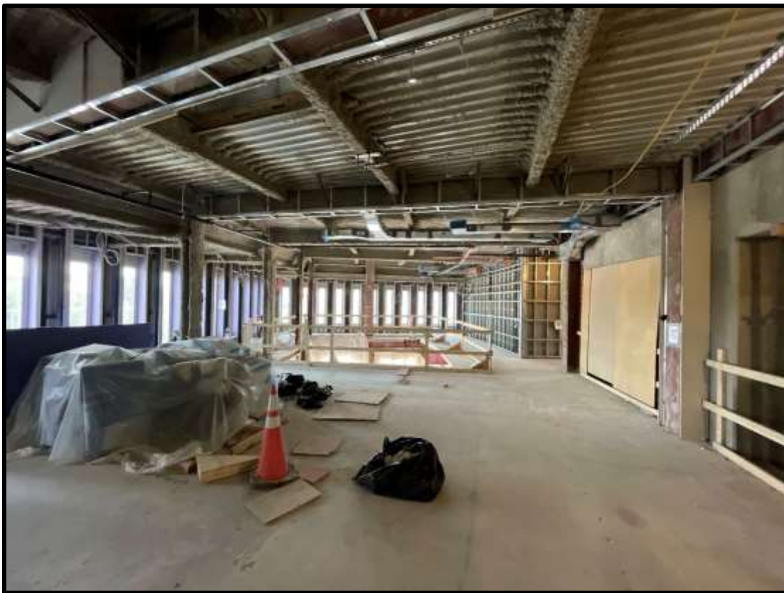
View of Work Ongoing on Level 4
