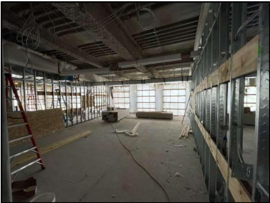
View of Work Ongoing on Level 2
