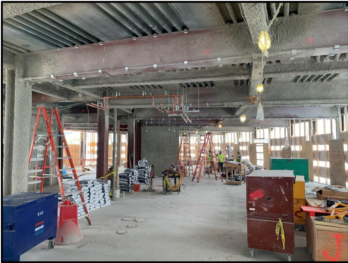
View of Work Ongoing on Level 1
