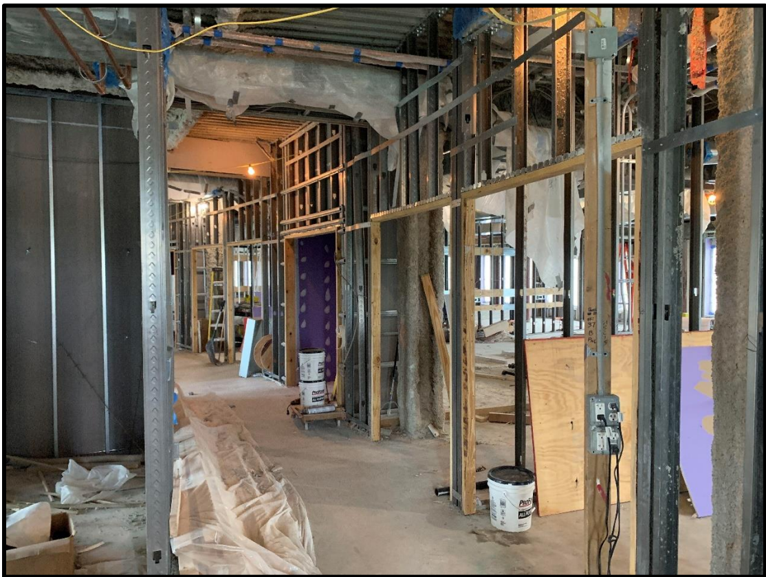
View of Work Ongoing on Level 4
