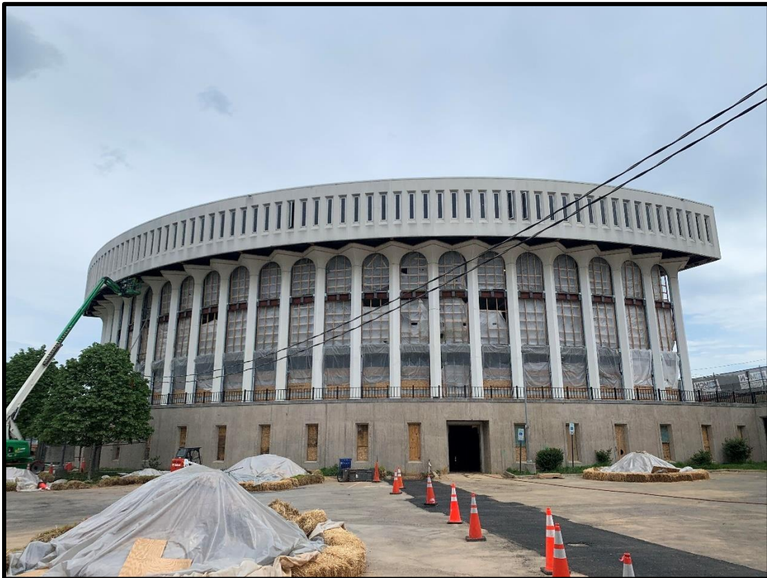
View of the Rear of the Building
