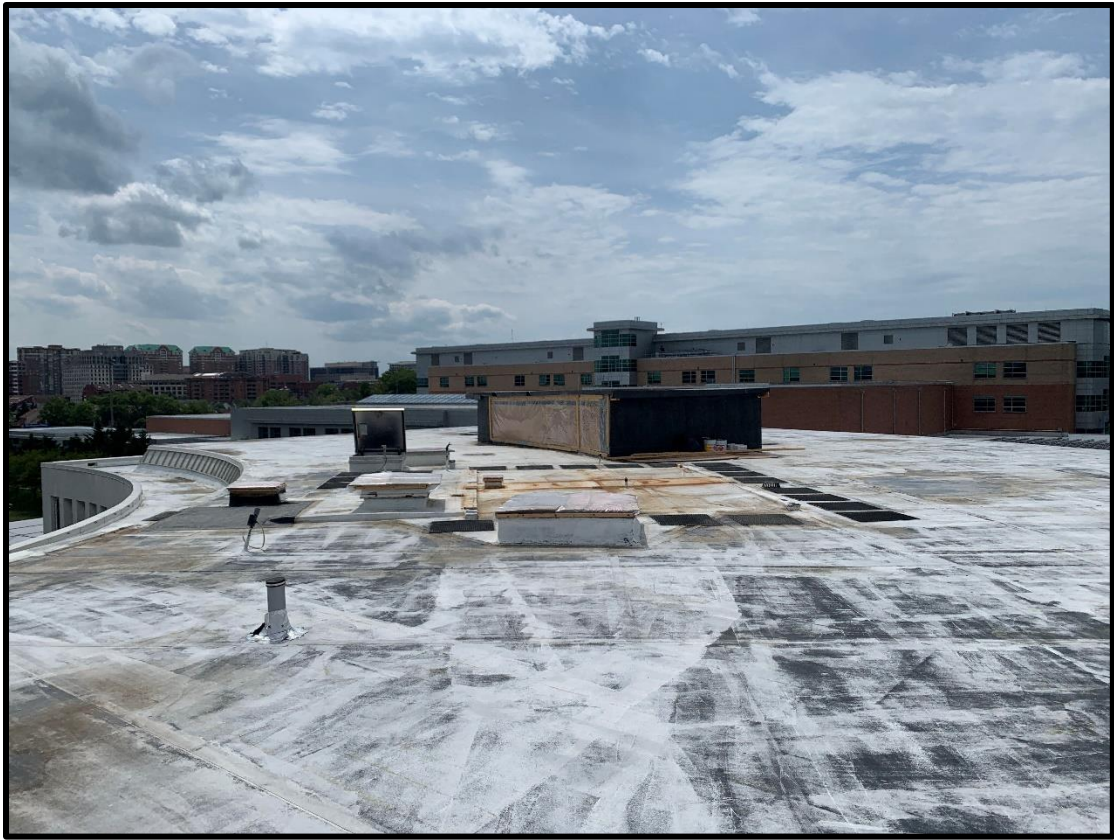
View of Working Ongoing on Roof
