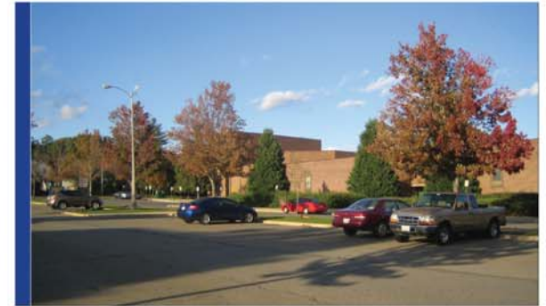
View towards Middle School main entrance from parking lot
