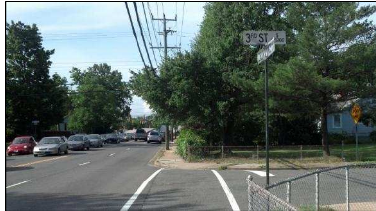
Narrow sidewalks with obstructions and without buffer along Carlin Springs Rd
