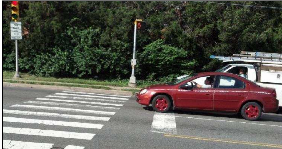
Crosswalk without curb ramp
