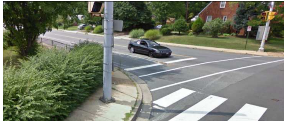
Limited curb space for queuing (for pedestrians waiting for a 'walk' signal)
