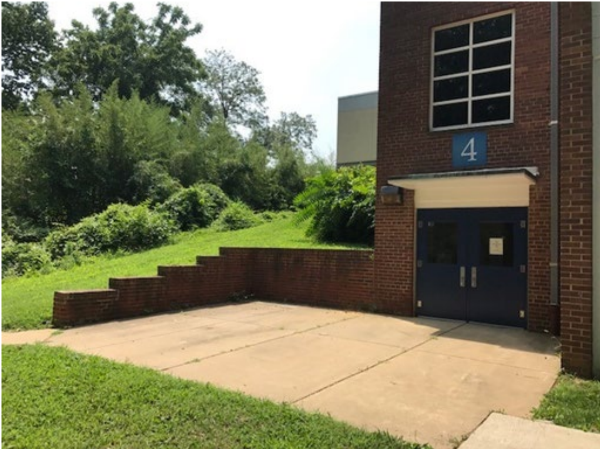
Photo 1.3 Exterior door that would provide access to the construction area
