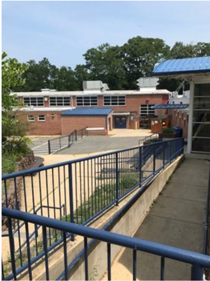
Photo 2.3 Existing exterior ramp
