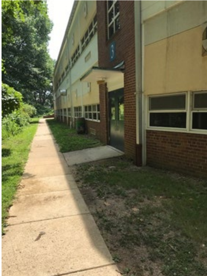
Photo 4.4 West side access
