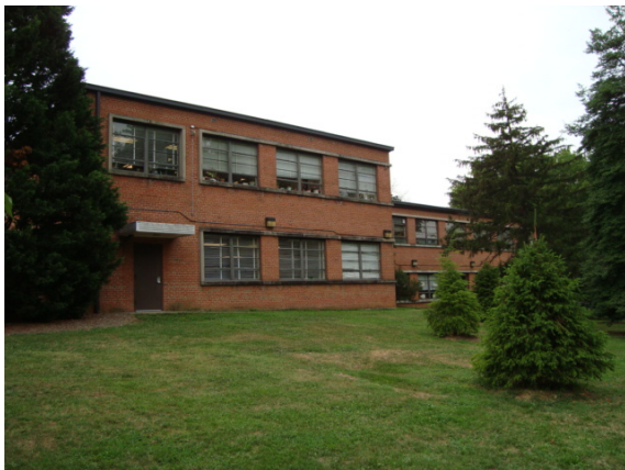
Photo #5: Building rear elevation
