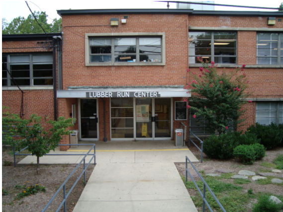
Photo #1: Building entrance
