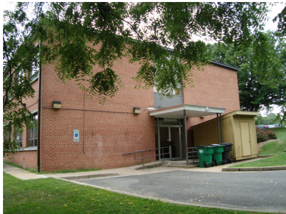
Photo #4: Building left side elevation
