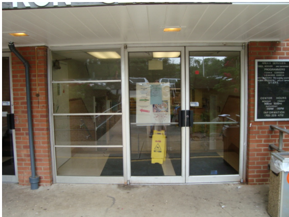
Photo #11: Entrance doors
