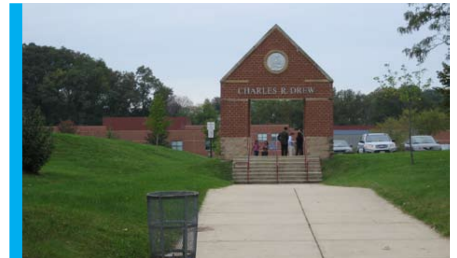
Entrance gate at pedestrian access
