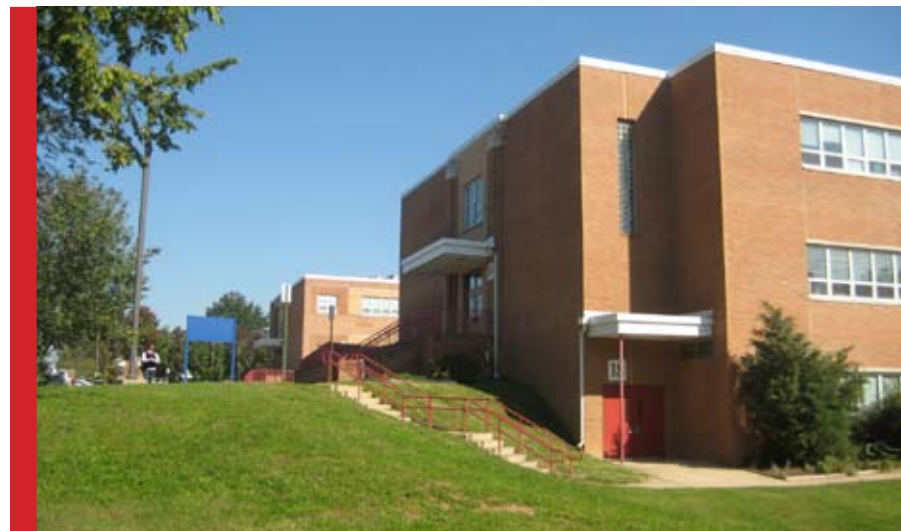
Access to fields from Queen St.
