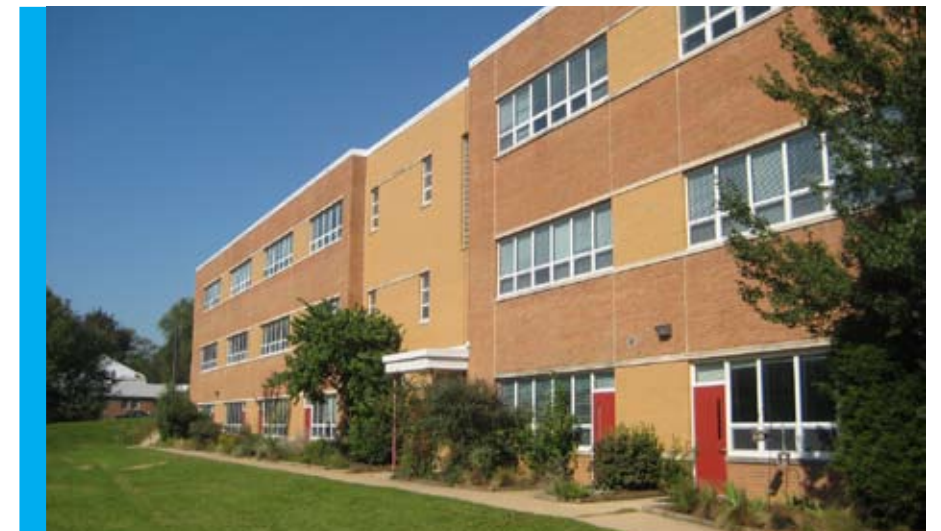
1999-2000 Addition to school
