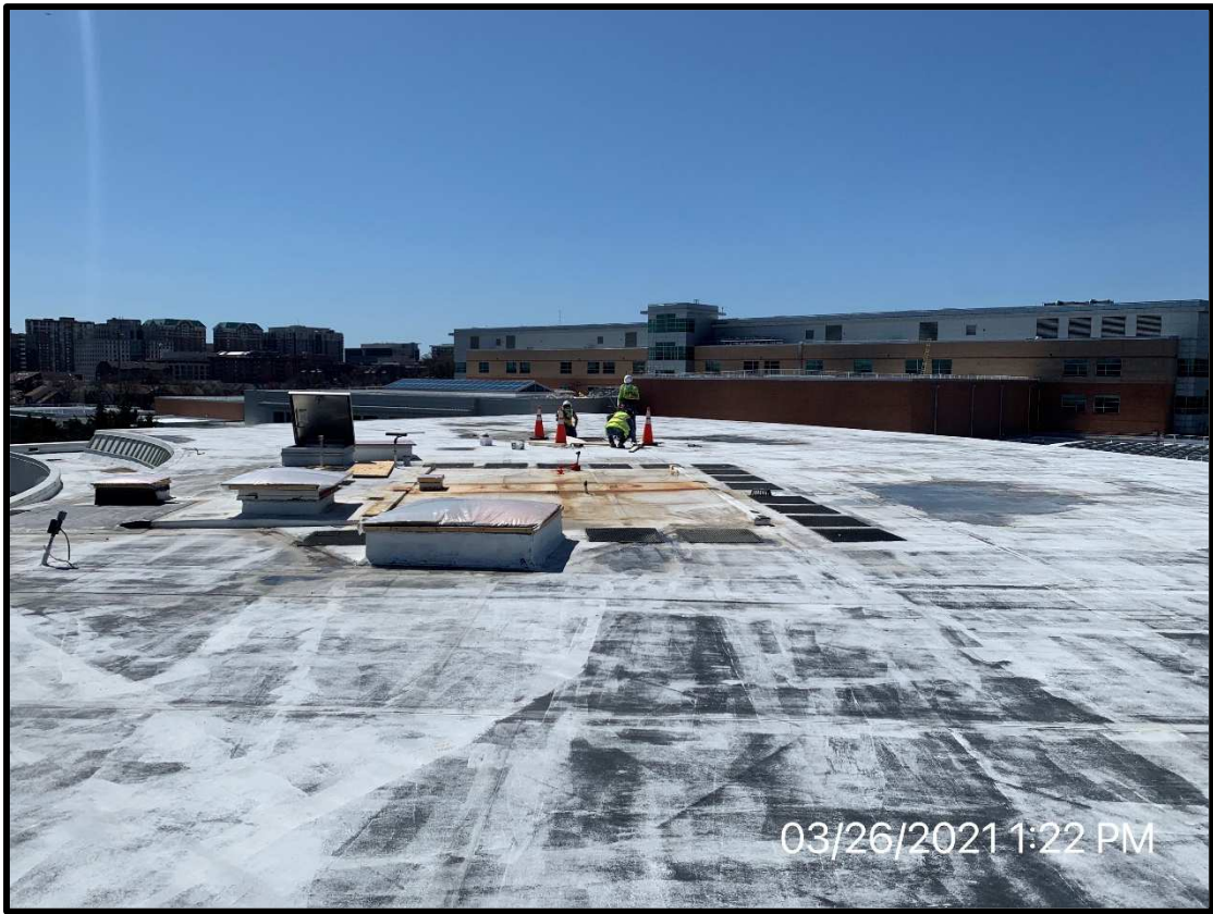
View of Working Ongoing on Roof
