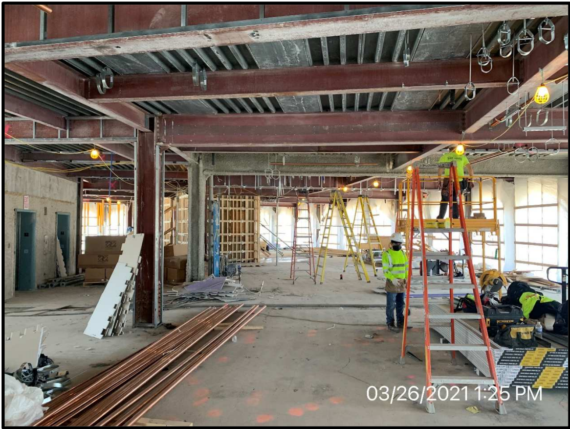
View of Work Ongoing on Level 3
