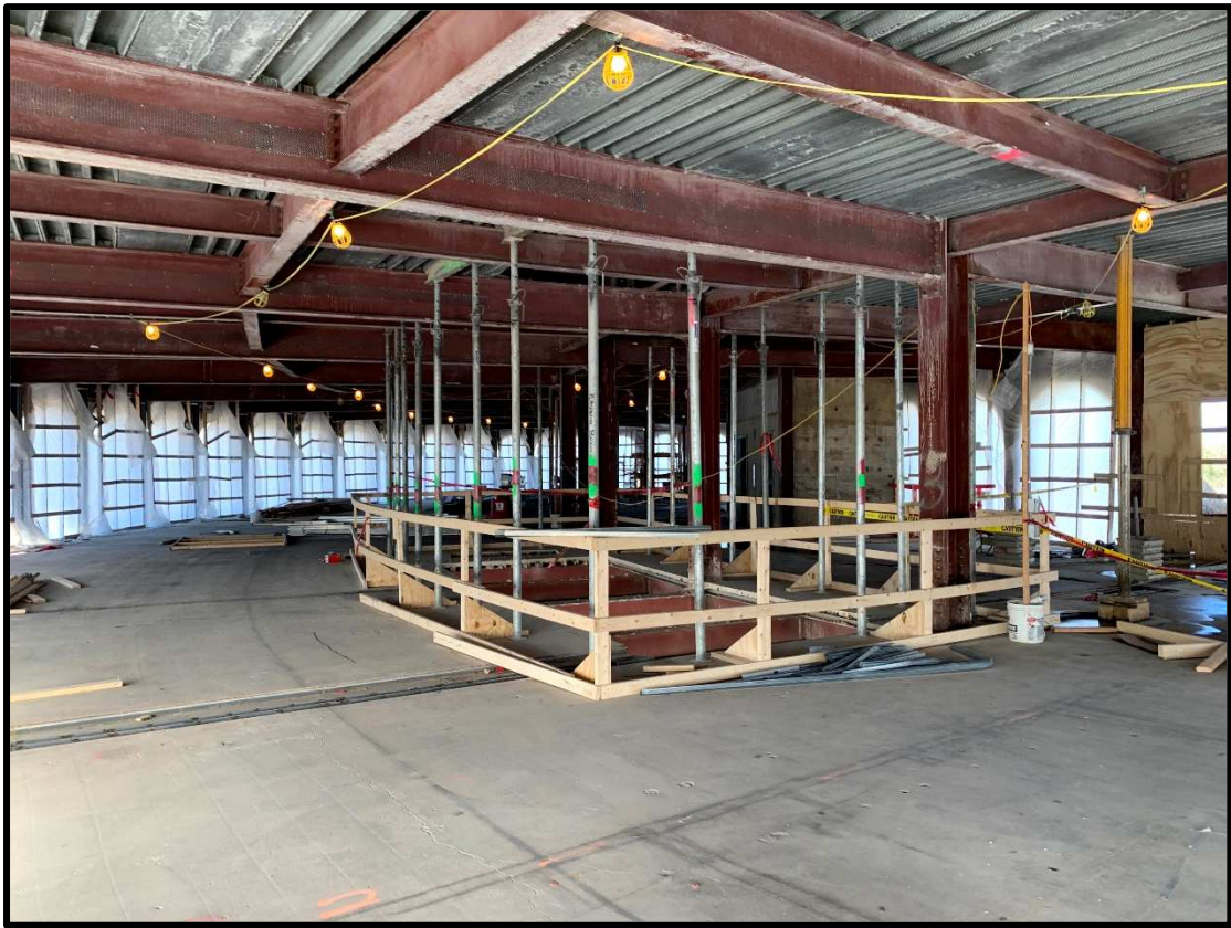
View of Work Ongoing on Level 3
