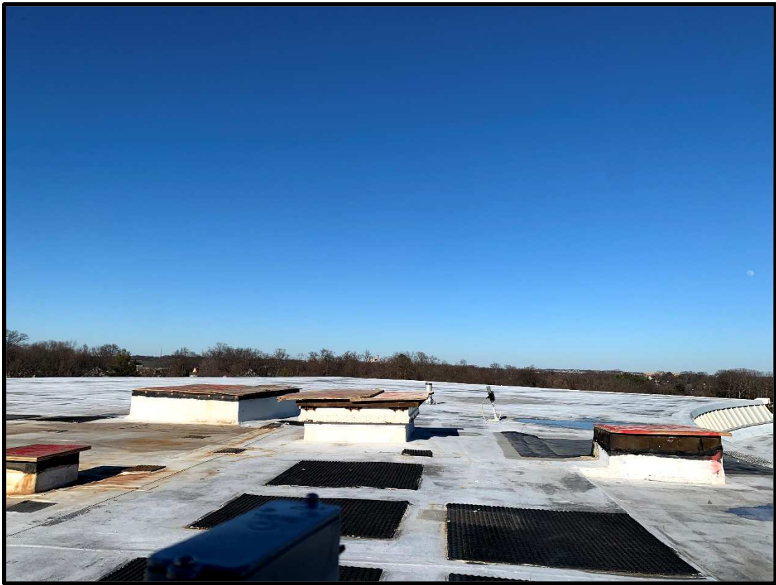
View of Working Ongoing on Roof
