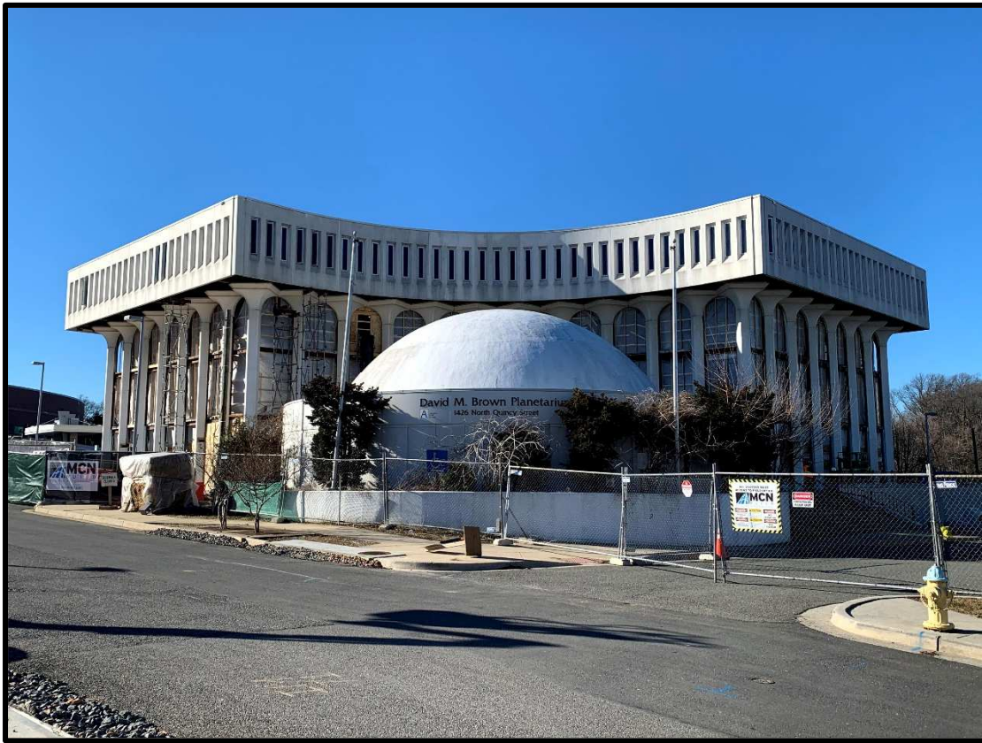
View of the Front of the Building
