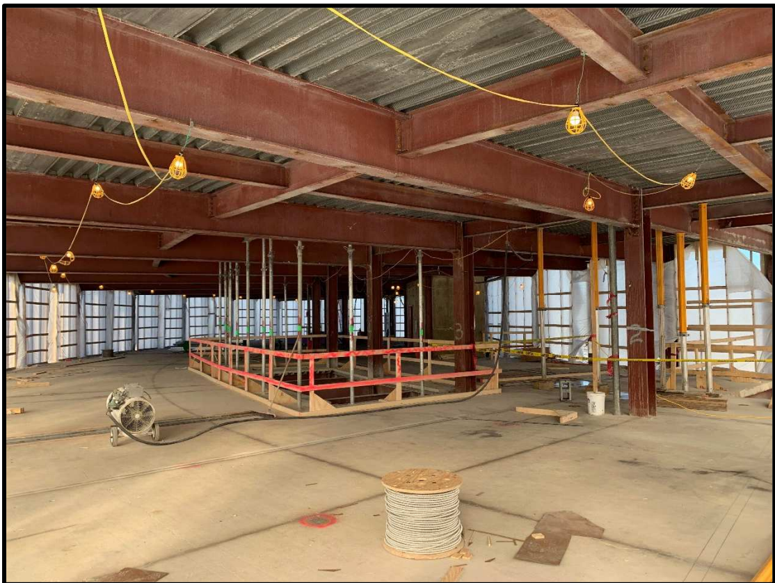
View of Work Ongoing on Level 2
