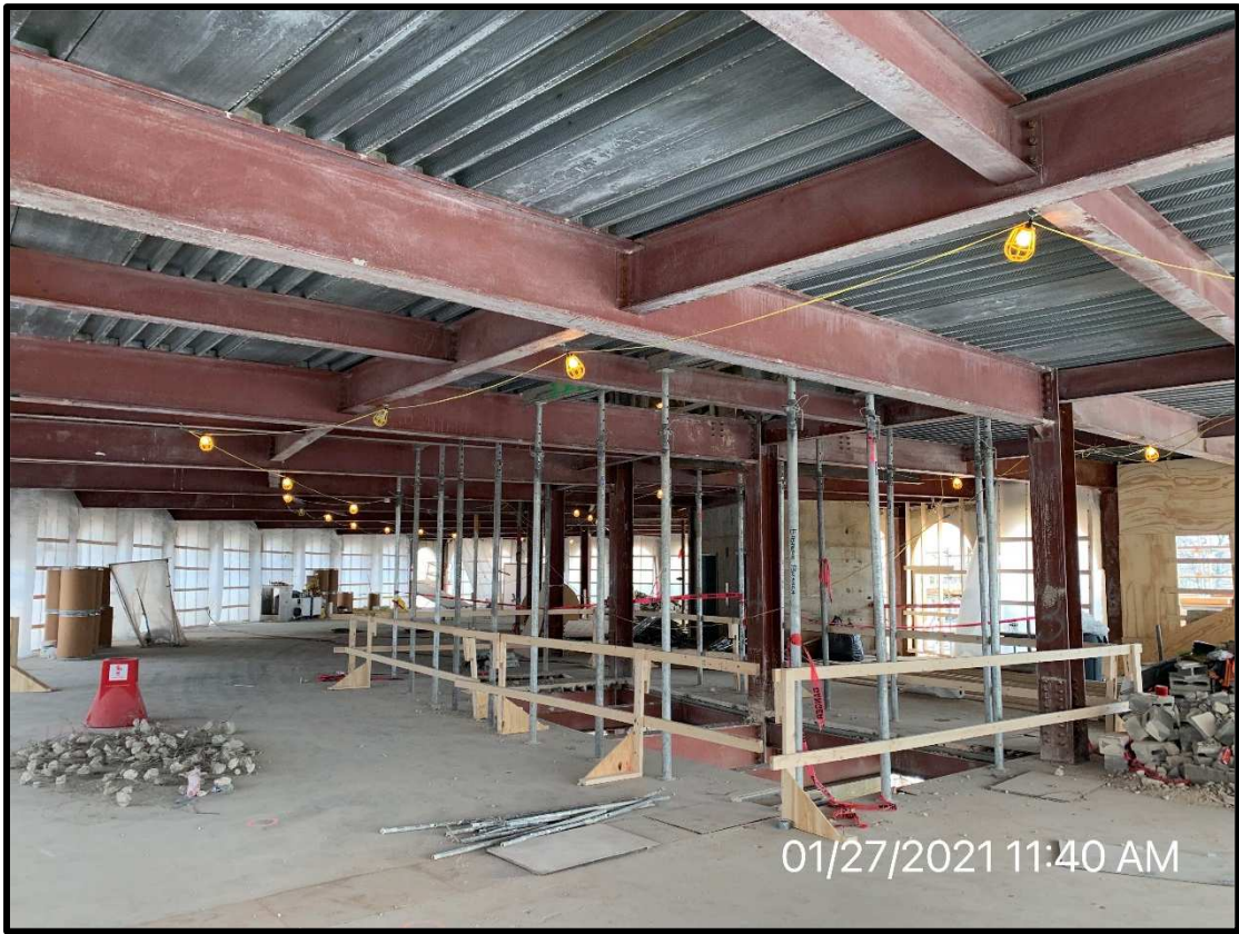
View of Work Ongoing on Level 3
