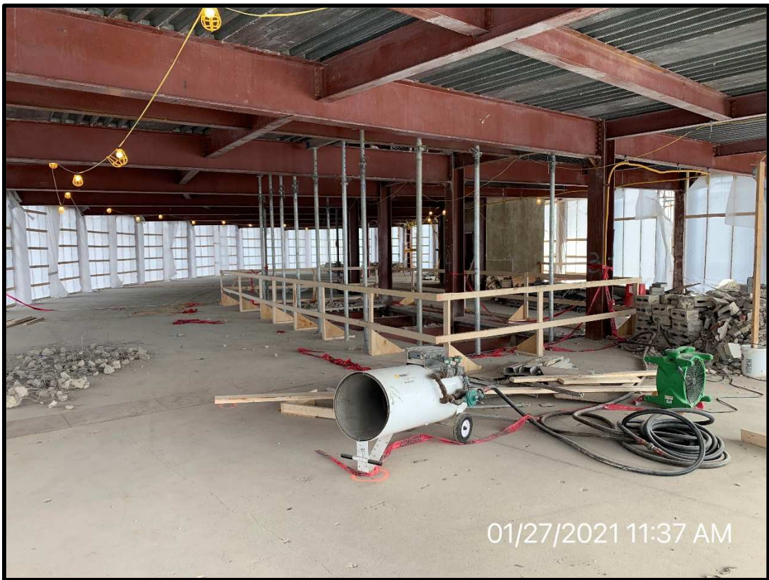
View of Work Ongoing on Level 2
