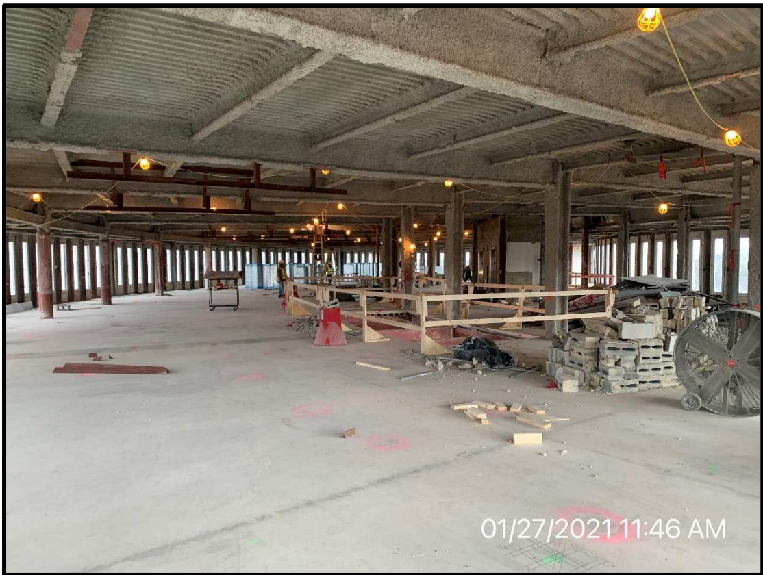
View of Work Ongoing on Level 4
