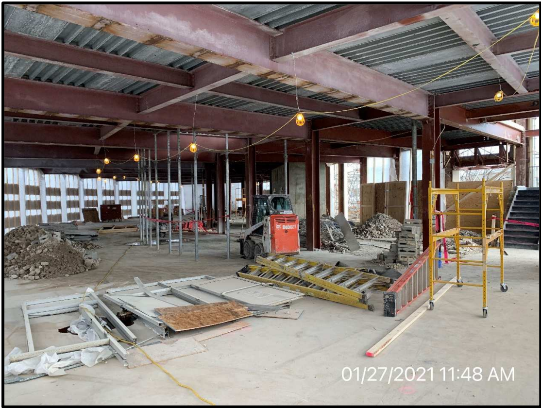
View of Work Ongoing on Level 1
