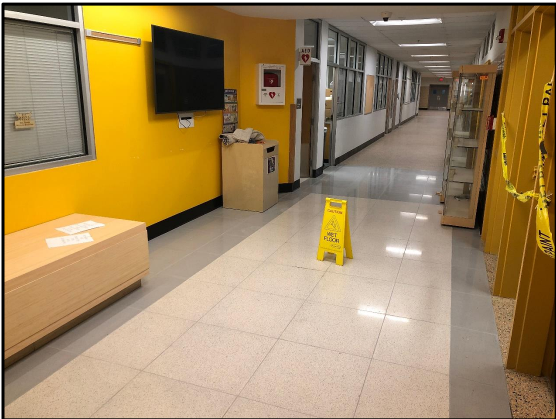
Installation of new terrazzo tile in renovation
