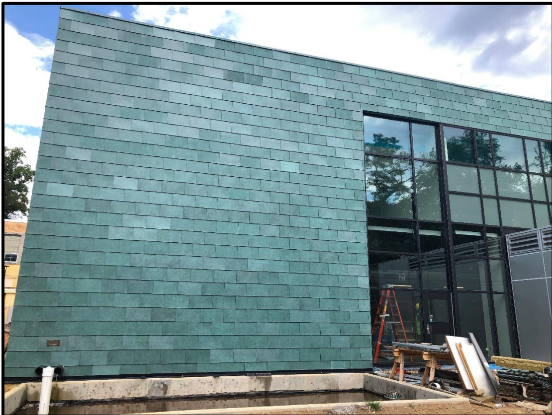
View of the west elevation of the addition
