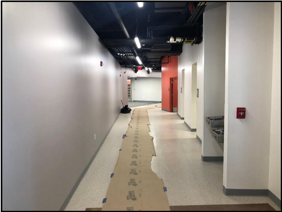
View of second floor corridor looking North
