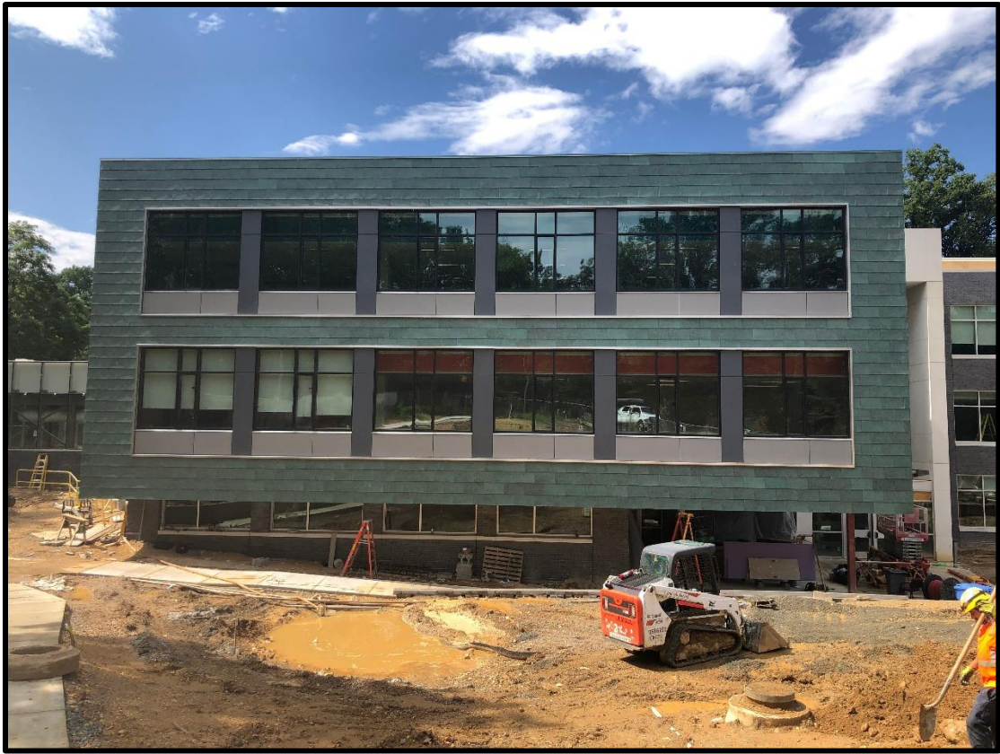
View of the south elevation of the addition
