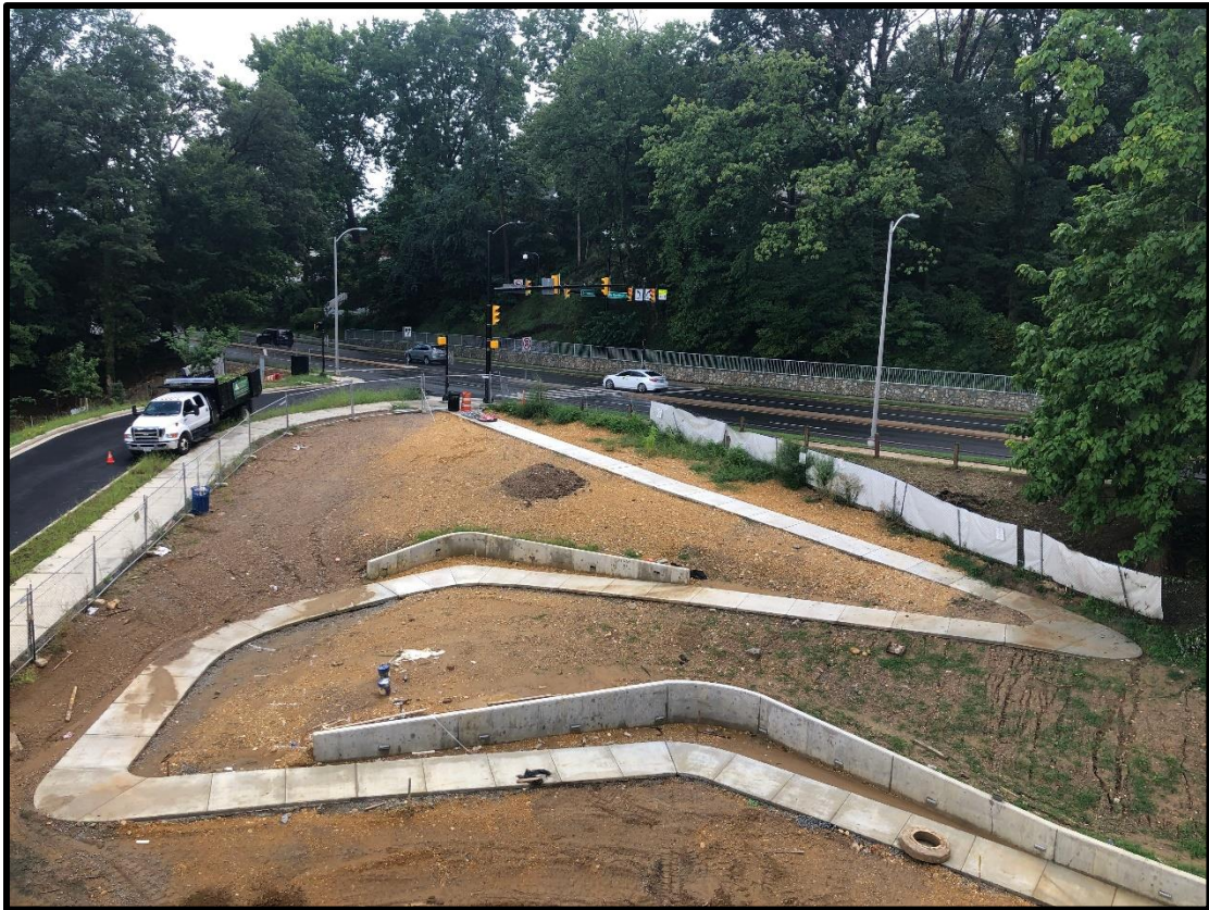
View of historical trail sidewalk installation
