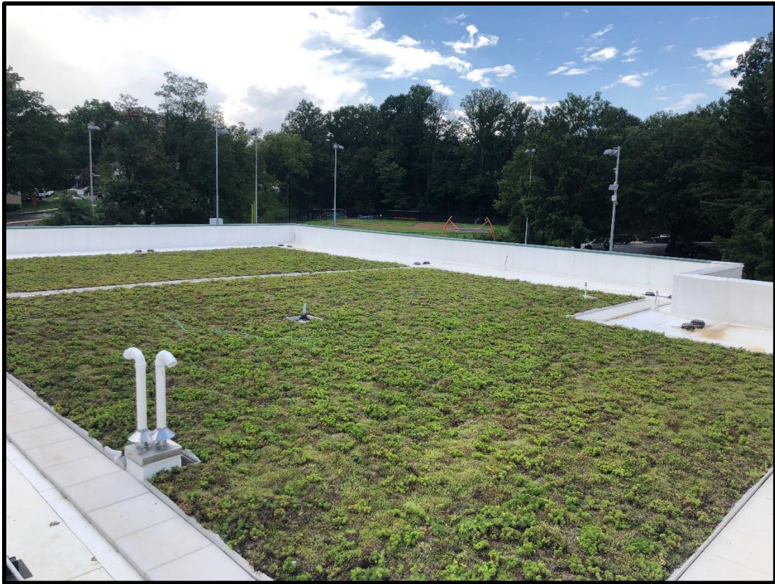
View of new roof and rainscreen installation
