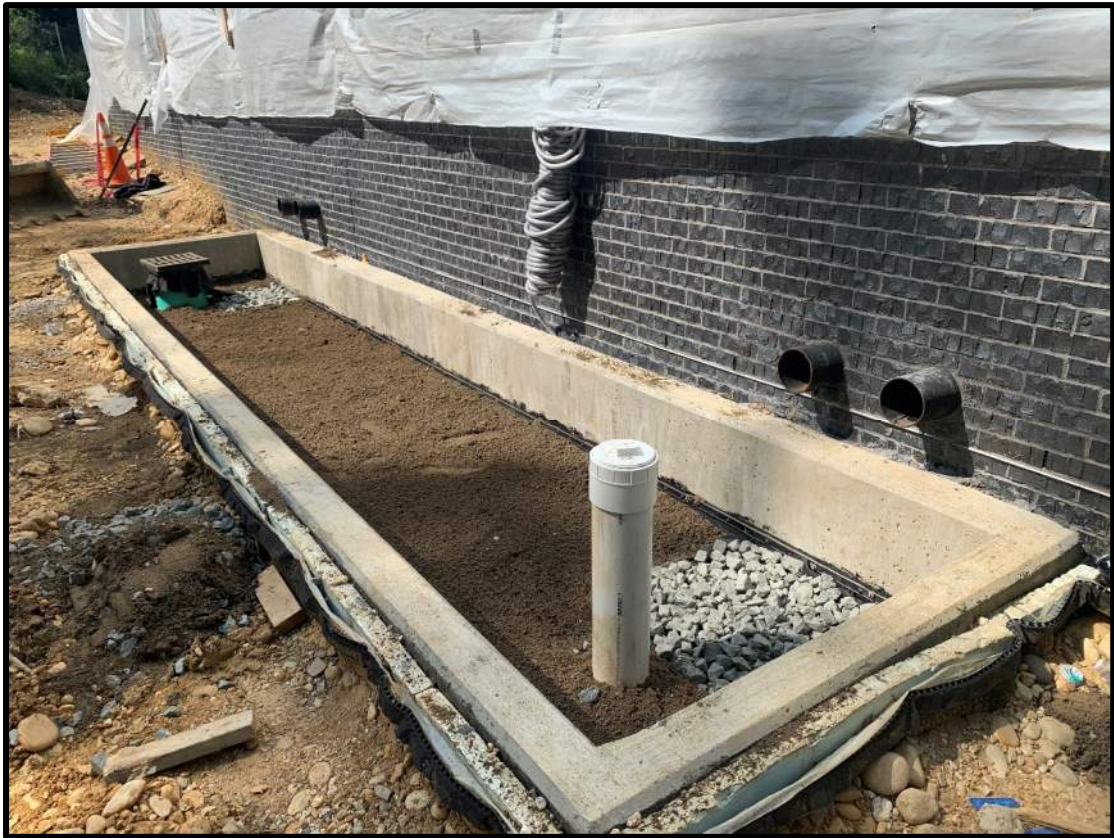
Bio pond installation ongoing
