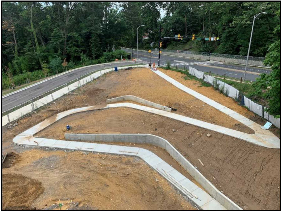
View of historical trail sidewalk installation
