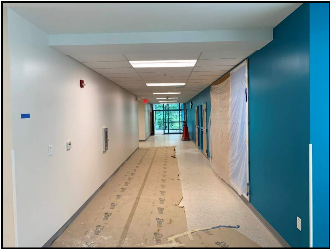
View of third floor corridor
