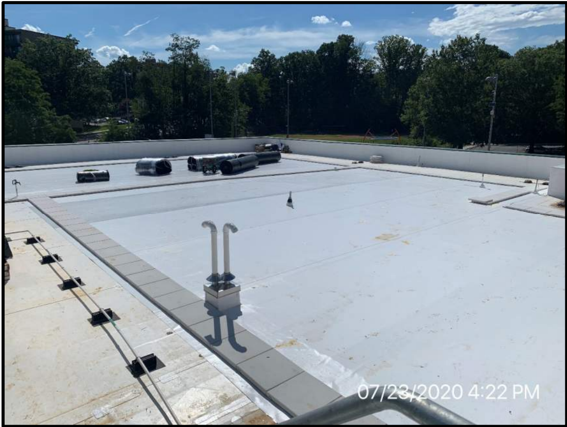
View of new roof and rainscreen installation
