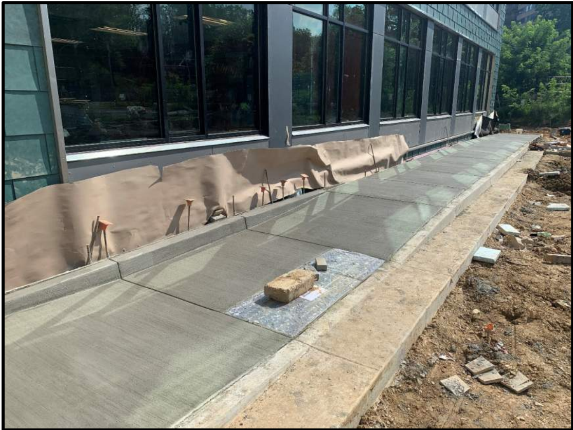
Front entrance sidewalk installation.
