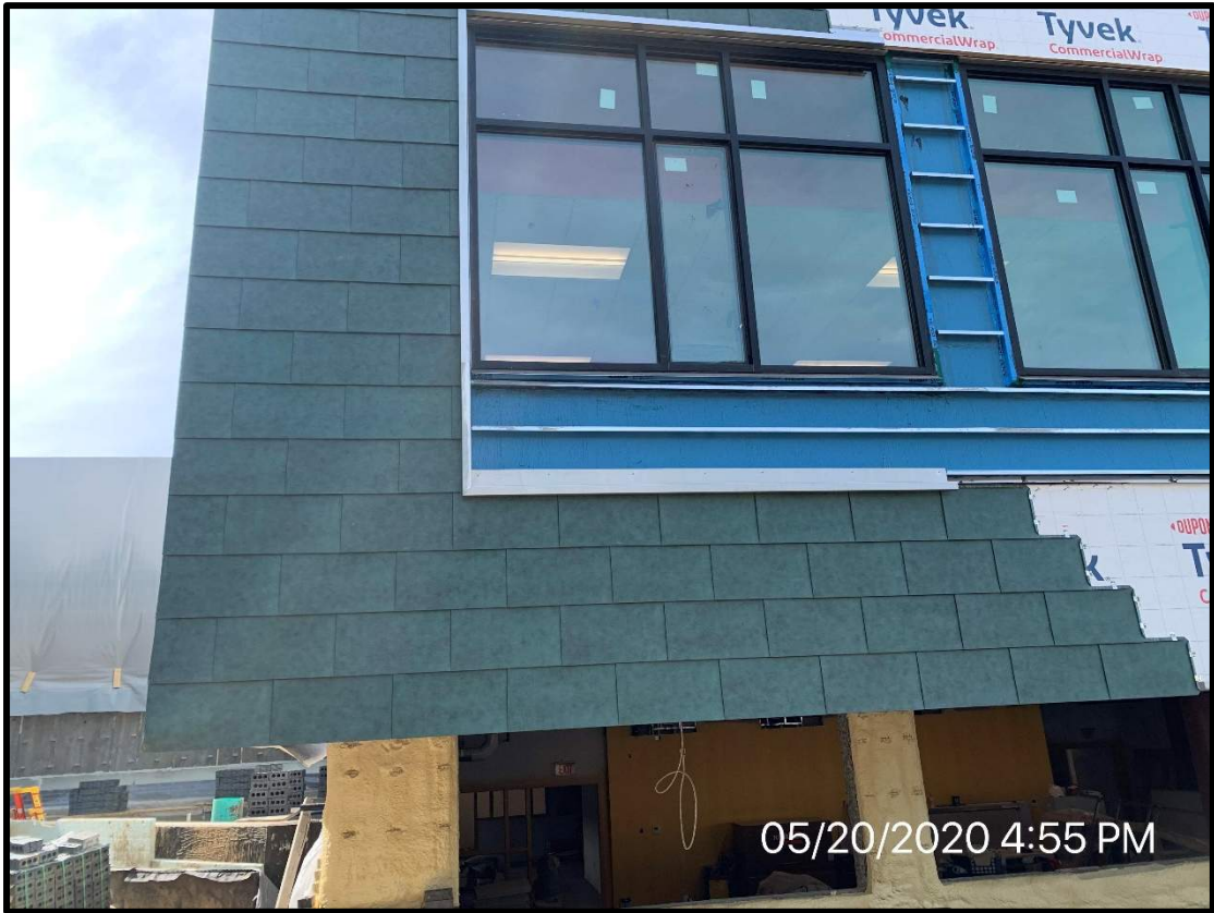
View of copper panel mockup for the addition
