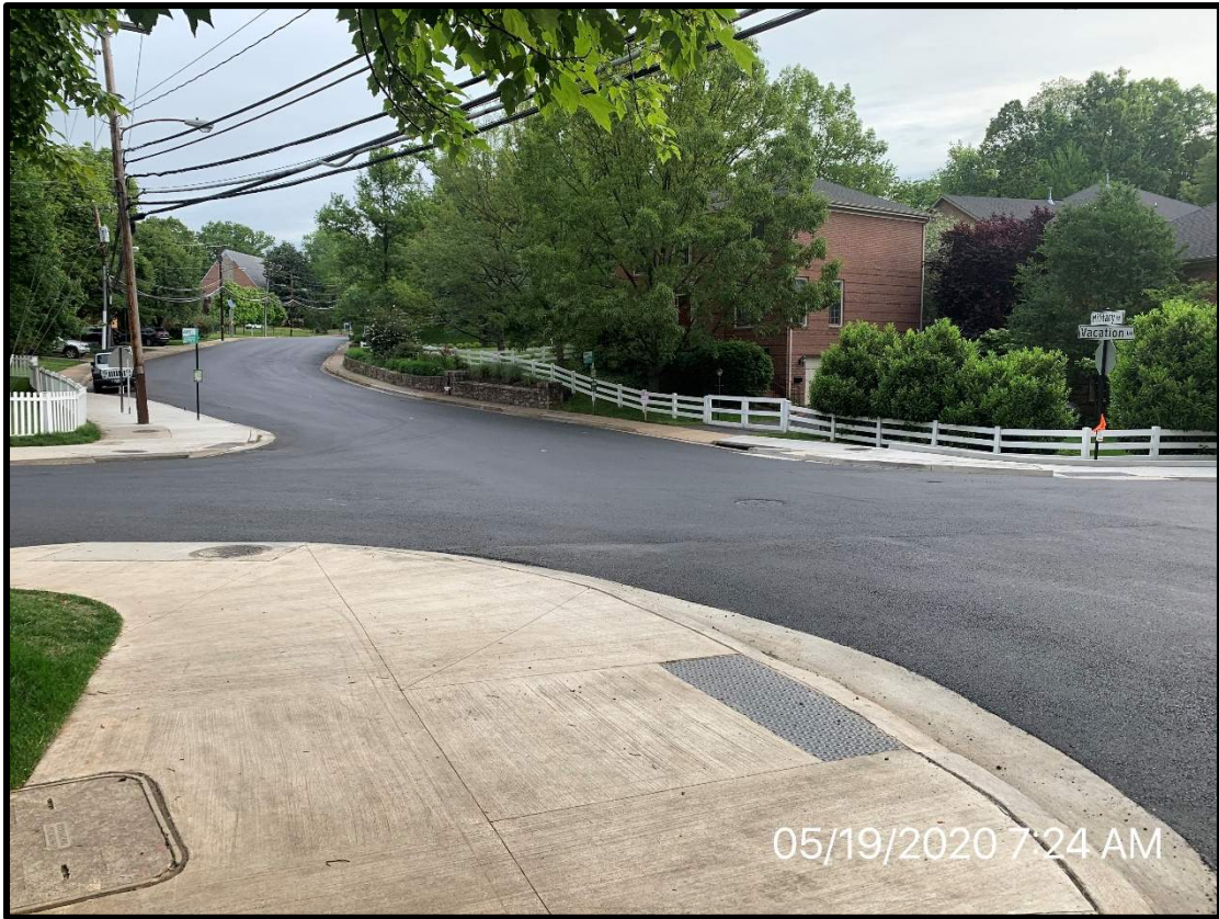
Exterior work along vacation lane ongoing
