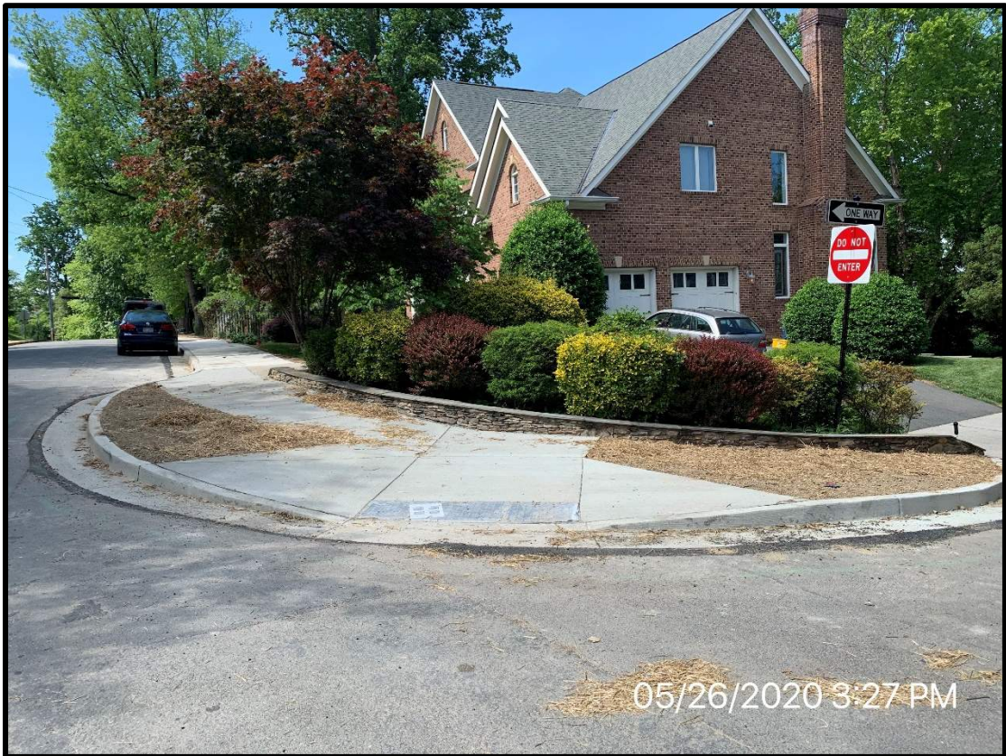
Exterior work along vacation lane ongoing
