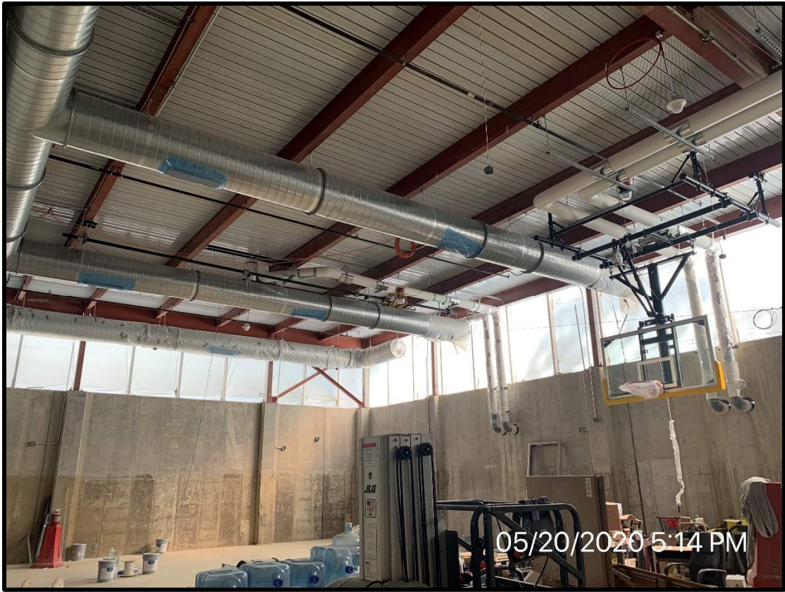
View of new auxiliary gym area
