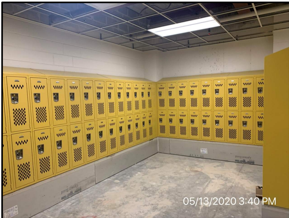
View of new locker rooms (typical)
