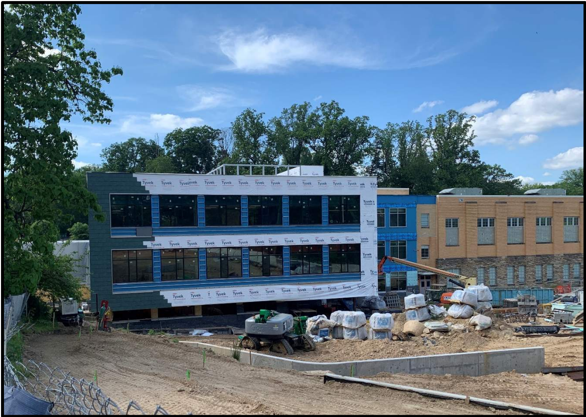
View of the south elevation of the addition
