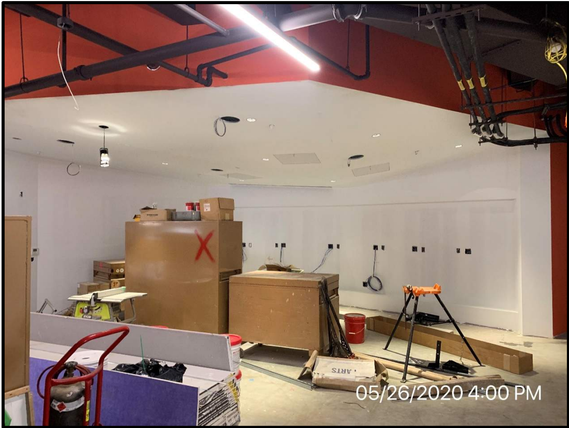
View of new student commons area
