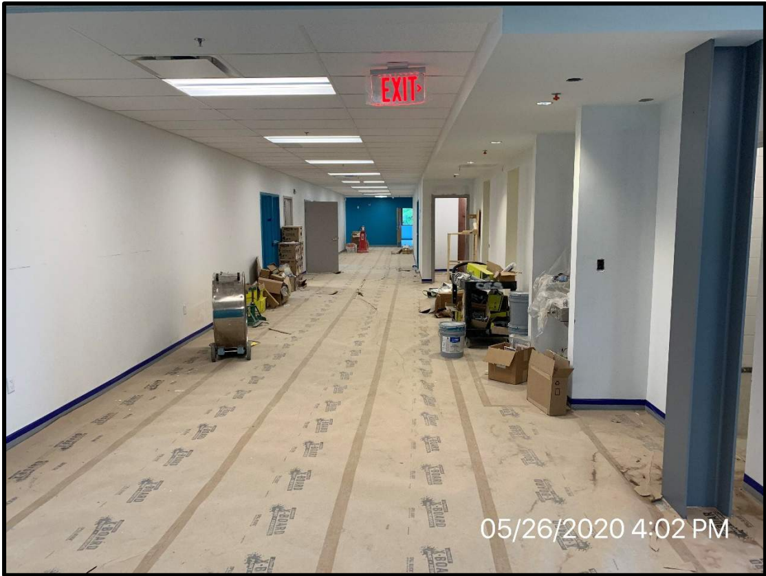
View of third floor corridor looking North
