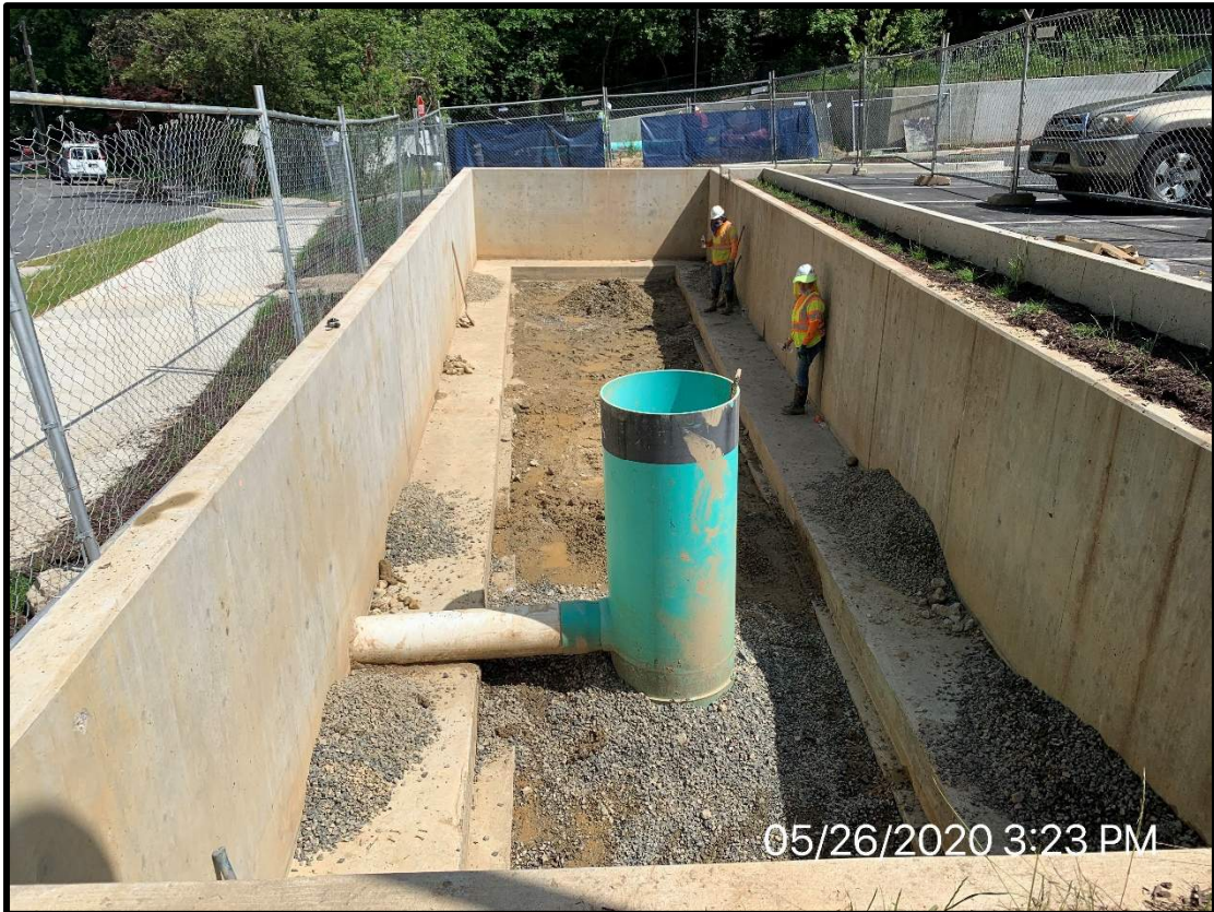
Bio pond installation ongoing
