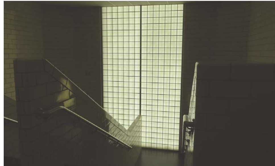
SOUTHEAST VIEW OF THE MAIN CENTRAL STAIR
