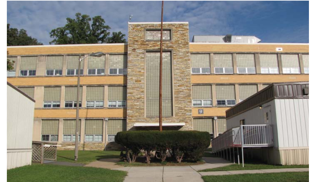
CENTRAL STAIR TOWER AND CENTRAL CLASSROOM BLOCK FACADE
