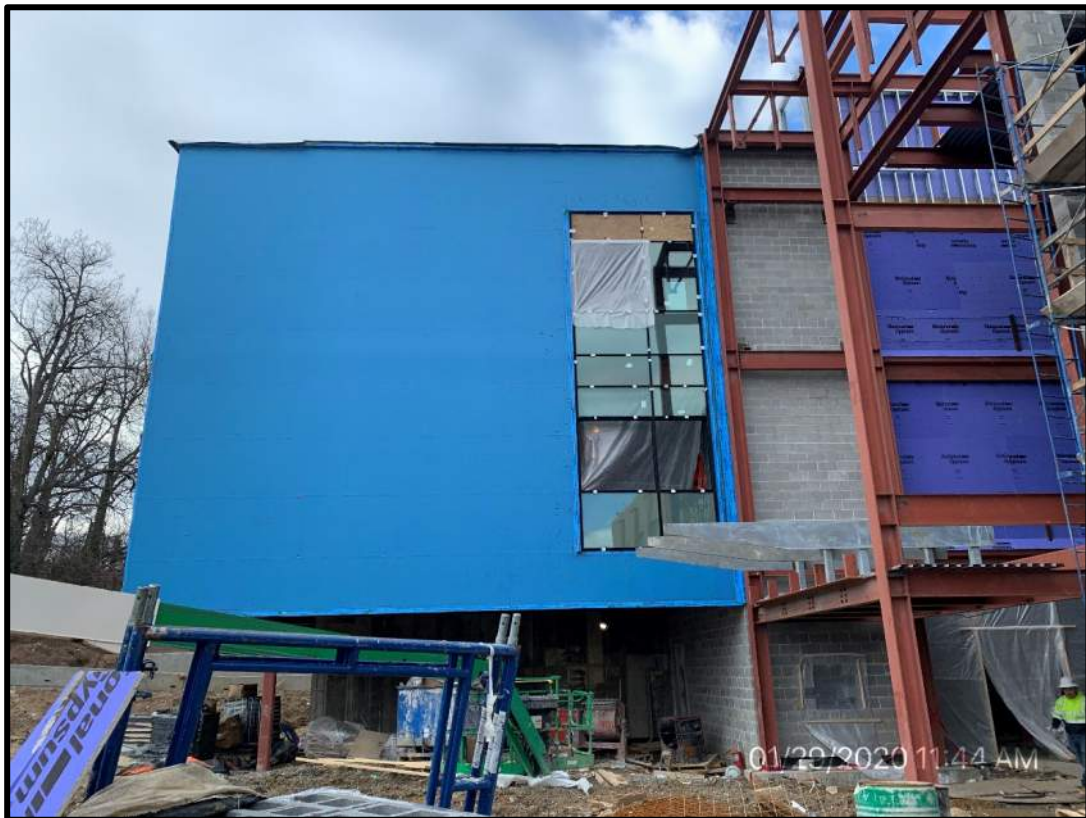
East elevation including new curtain wall
