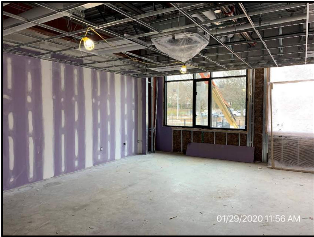
Current status of mock up classroom
