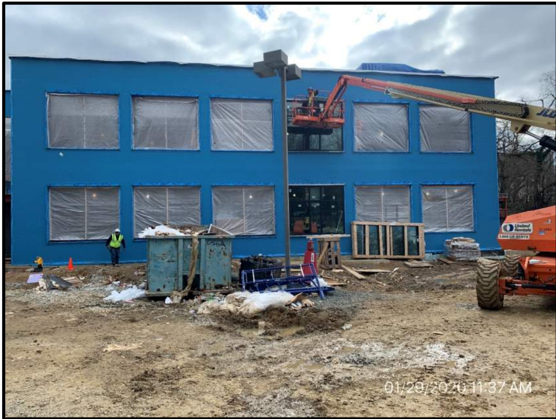
North face of the building current status with mock-up windows installed
