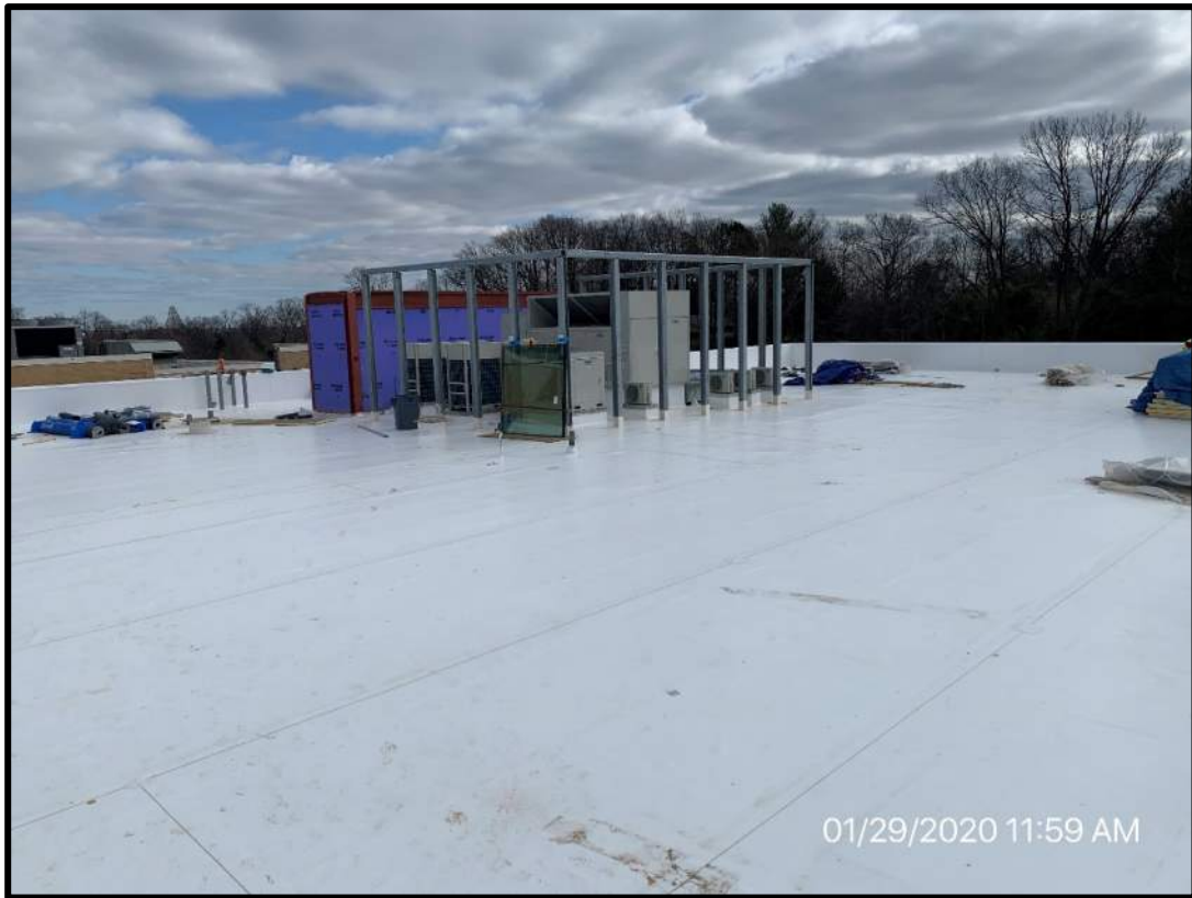
PVC roof installation current status (Main Roof)
