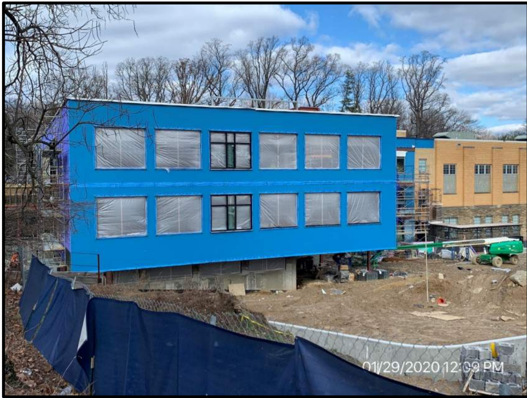
South elevation of building with mock-up windows installed
