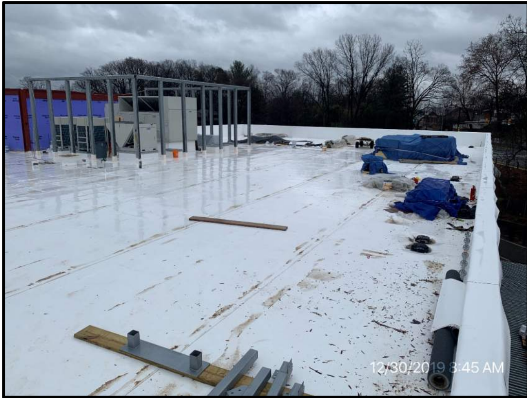
PVC roof installation current status
