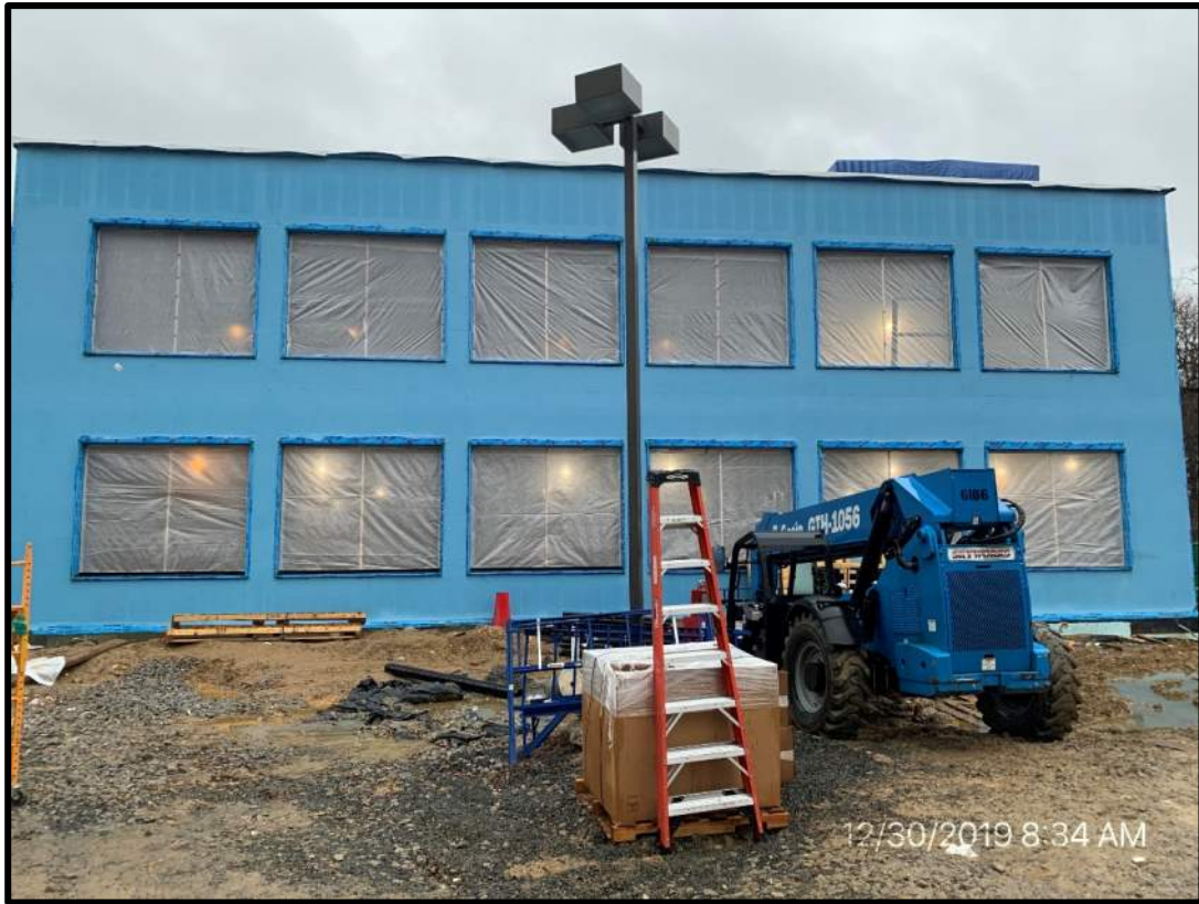
North face of the building current status
