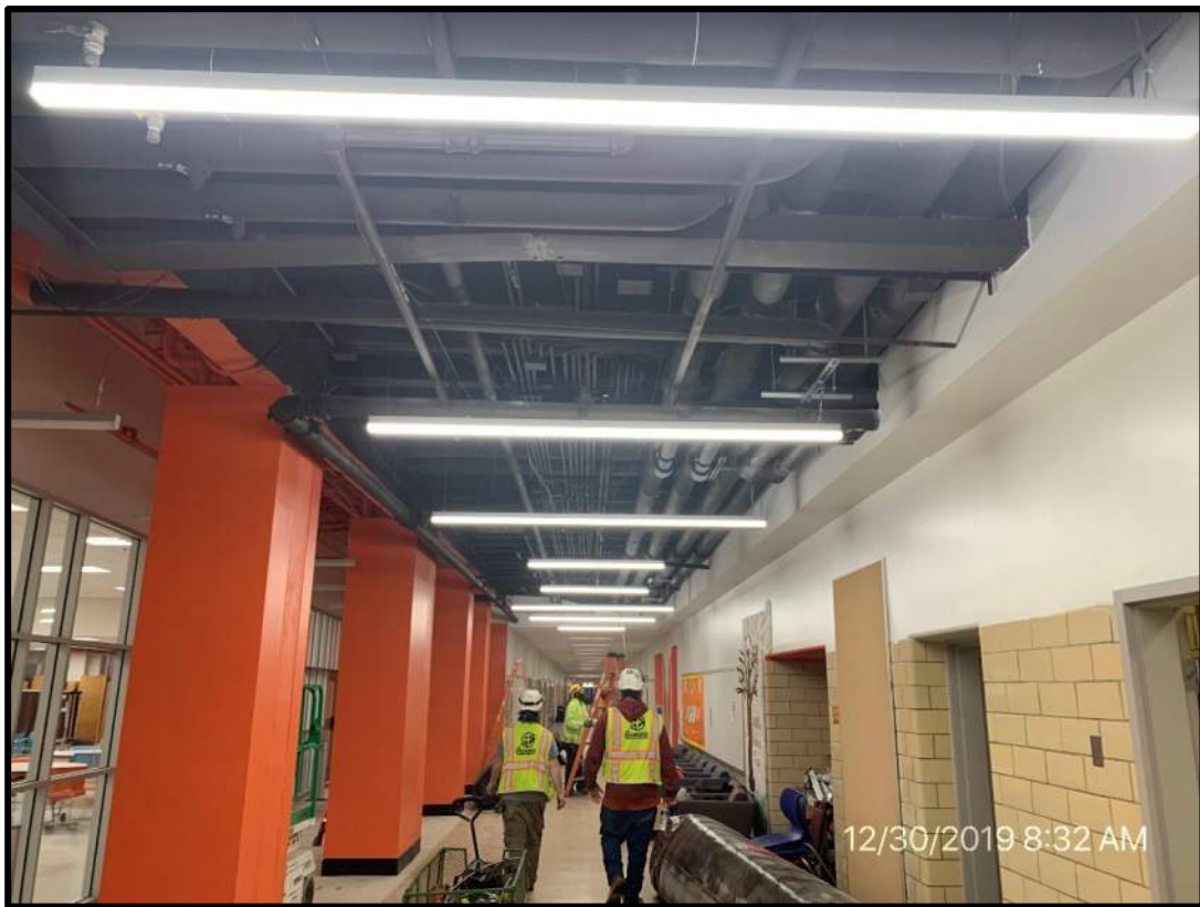
New permanent lighting in renovation cafeteria corridor
