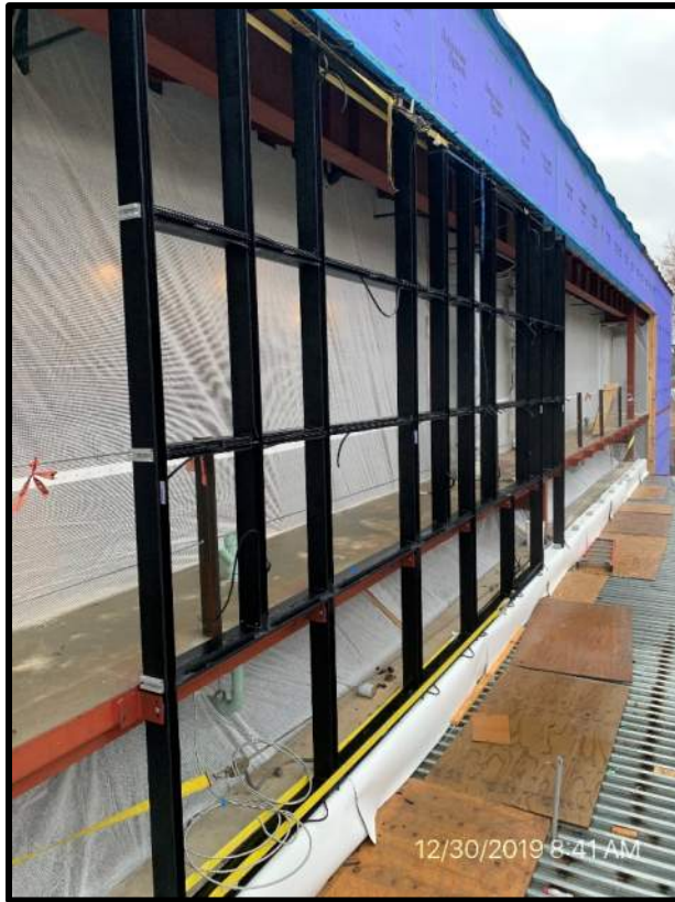
Exterior curtain wall erection status on West elevation
