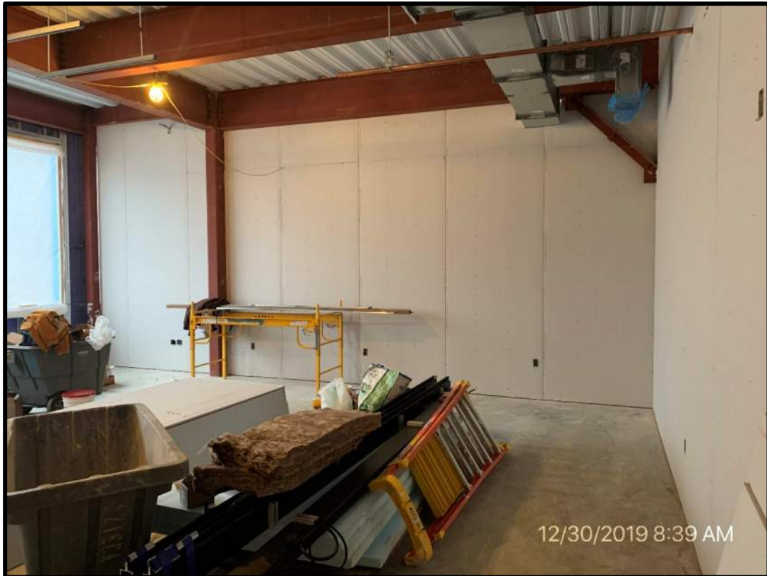
Current status of mockup classroom in the Addition
