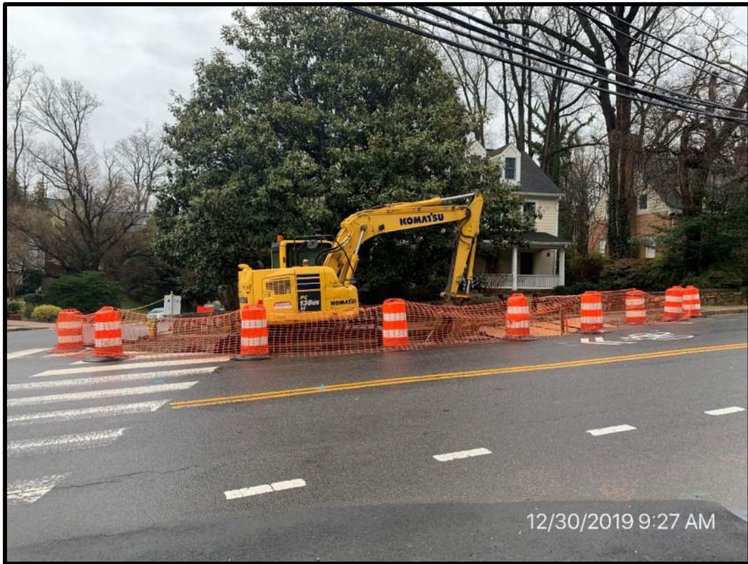
Current status of work at Military Road and Vacation Lane
