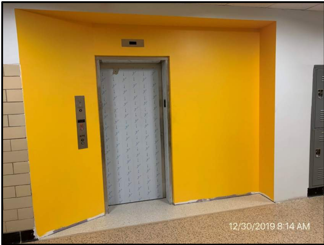
New elevator lobby at first floor in renovation.
