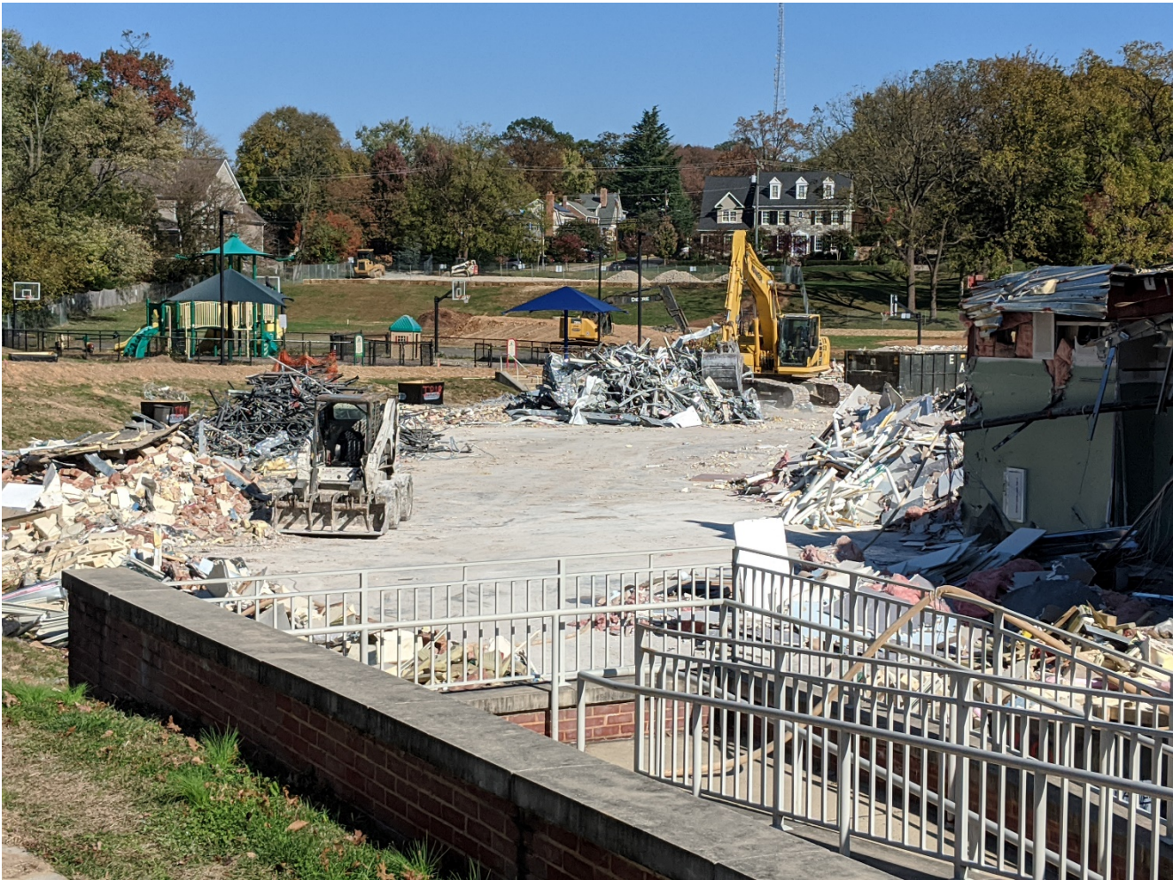
Exterior Building Demolition
