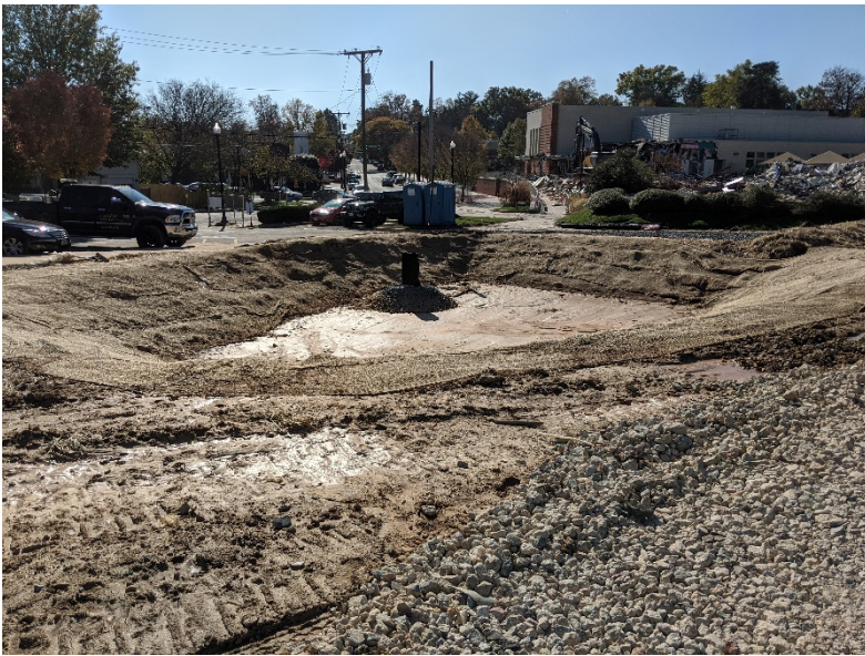
Installation of Erosion and Sediment control facilities
