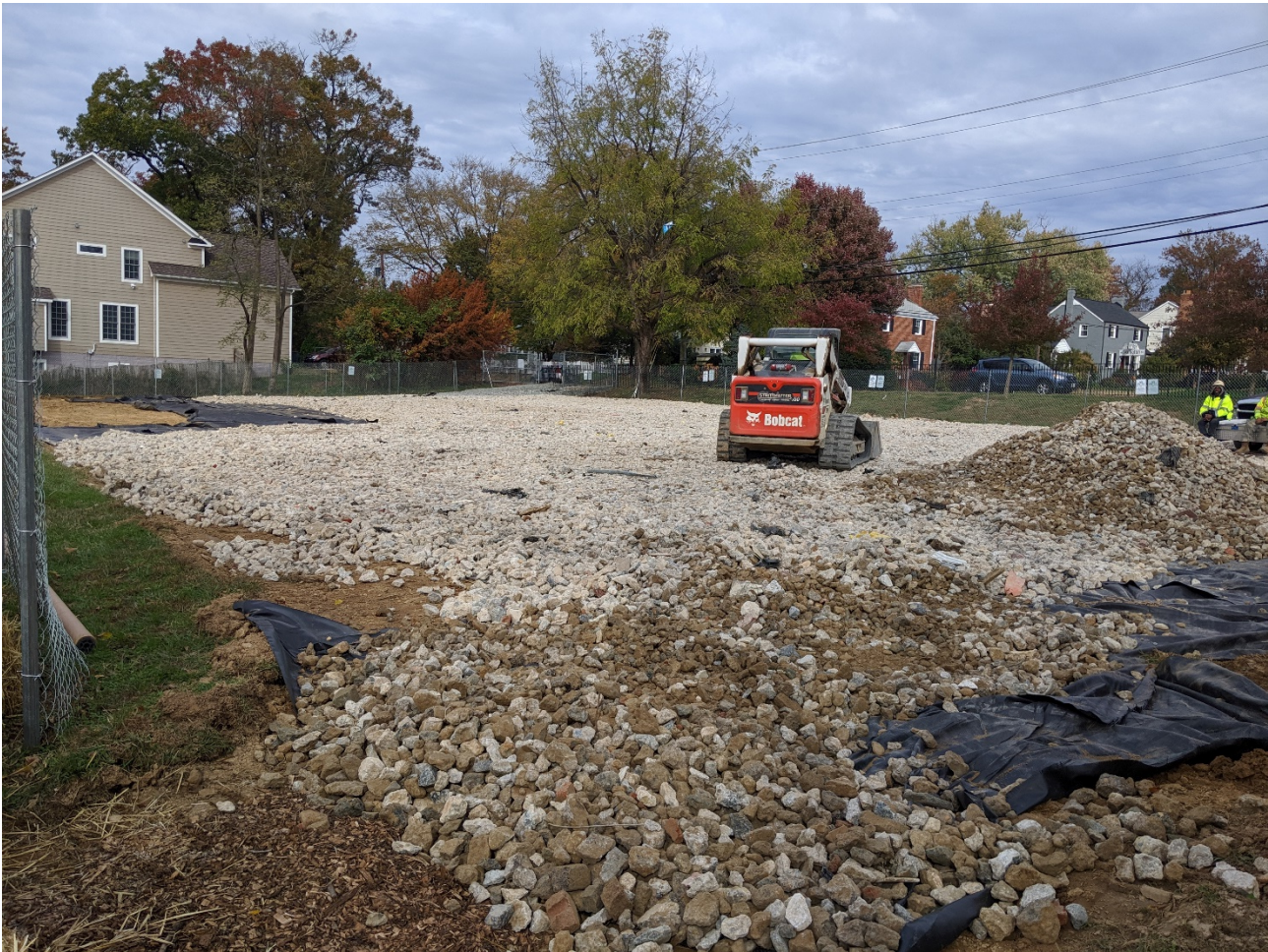
Temporary Construction Worker Parking Lot
