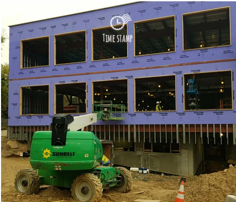
North and South side exterior framing and sheathing installation
