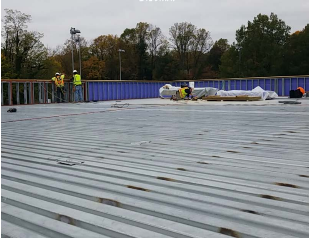
Metal deck roofing and parapet
