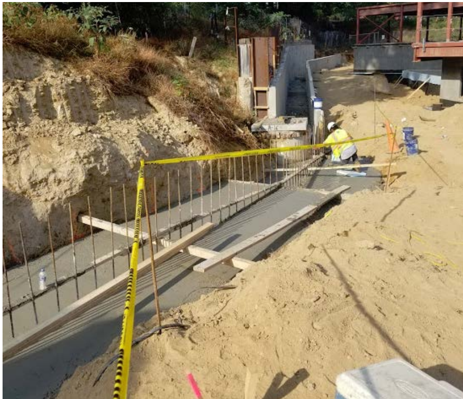
Concrete Footings for Site Walls
