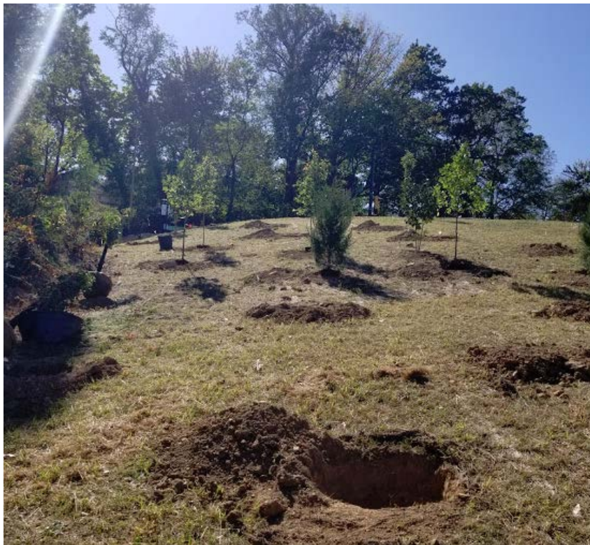
New trees and shrubs were planted throughout site
