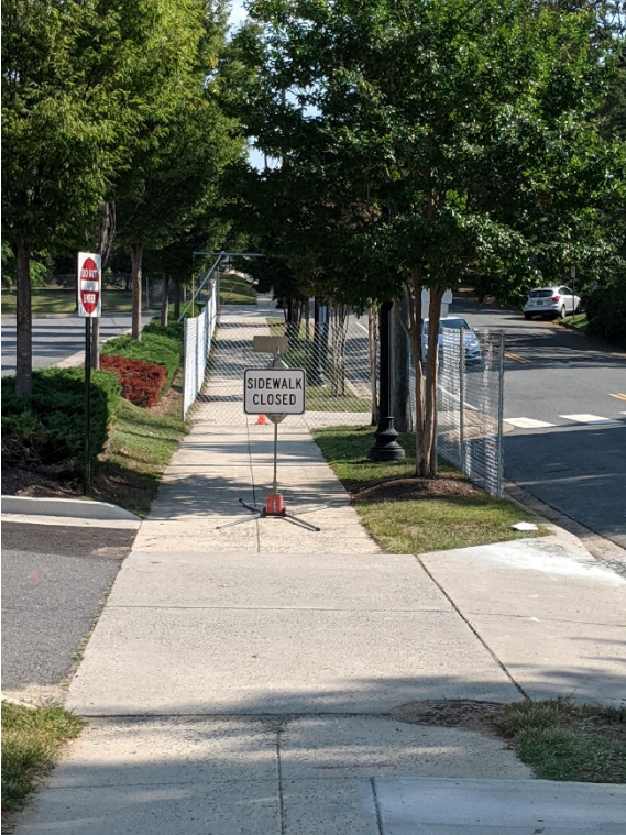
Installation of site perimeter fencing
