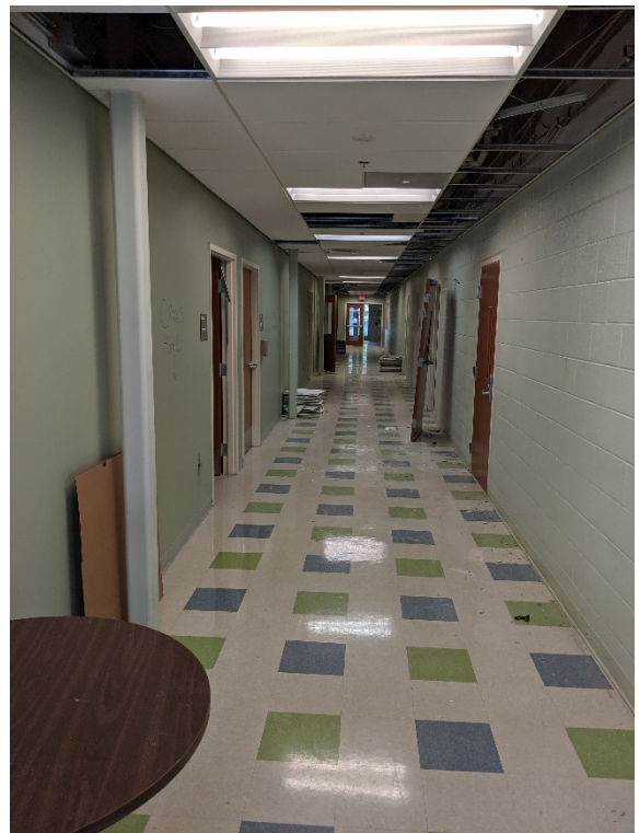
Interior building demolition investigations
