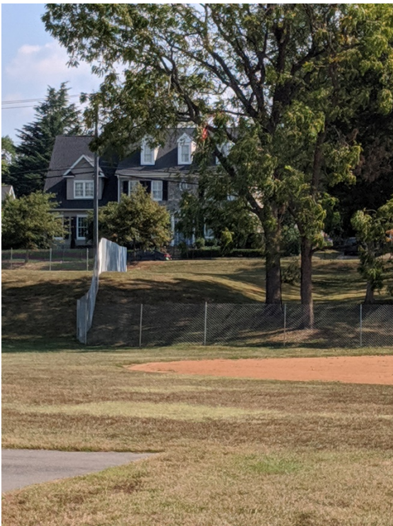
Installation of site perimeter fencing
