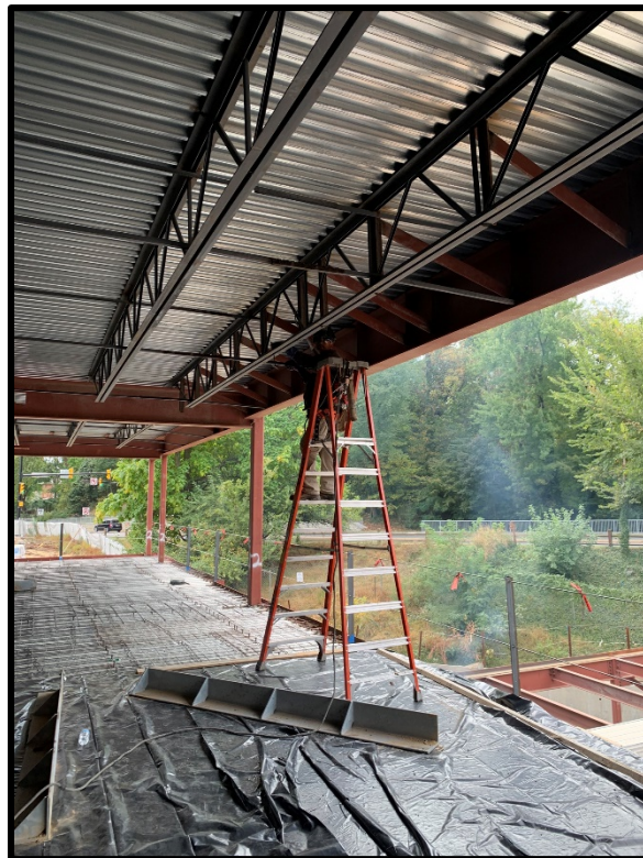
Final Steel Outriggers Being Welded In Place
