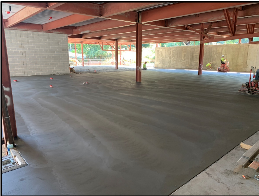
View of Structural Concrete Slab Finishing on Level 2
