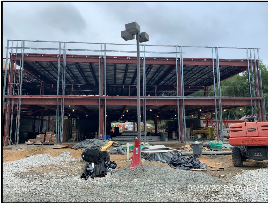
North Side of Addition Showing the Newly Installed Exterior Framing
