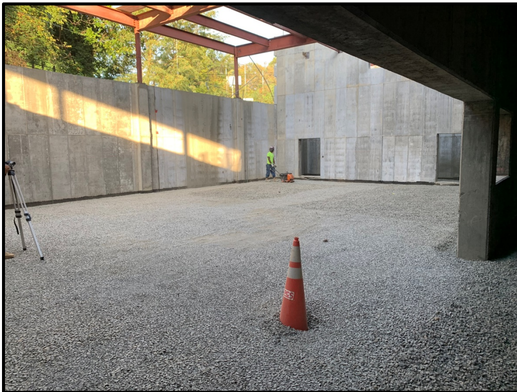
First Floor Subgrade Compaction Activity
