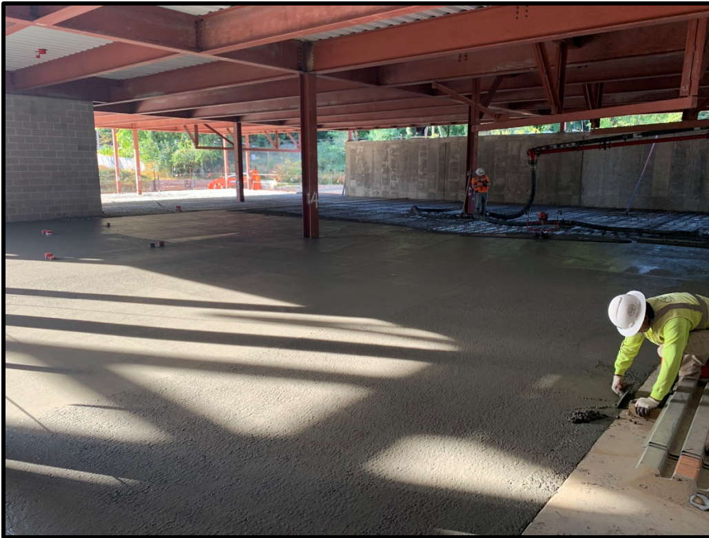
View of Structural Concrete Slab Installation on Level 2
