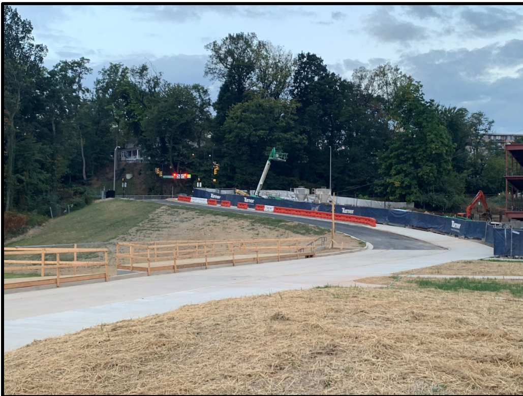
View of New Drop-Off and Pick-Up Traffic Lane
