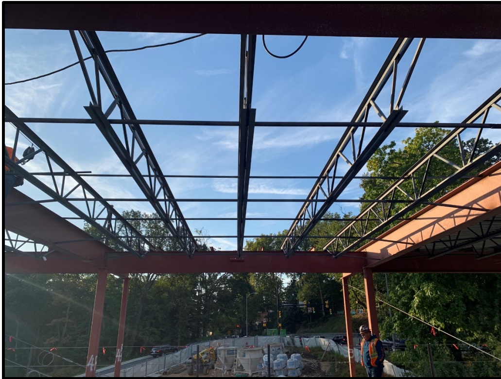
View of Completed Road Framing
