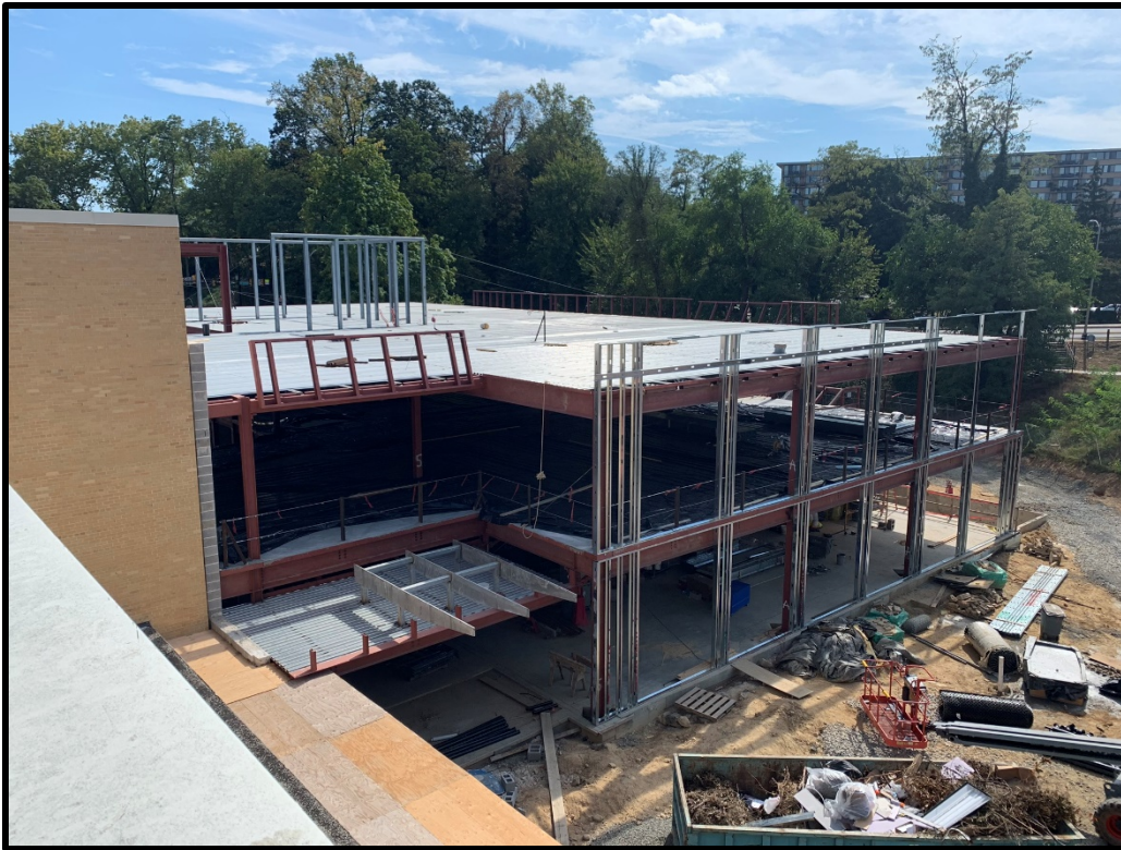
View of North Side of Addition Including Roof Metal Decking
