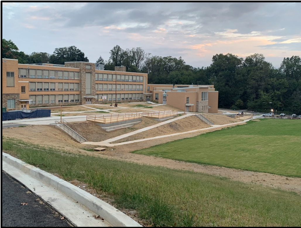
View of Rear of School With New Walkways, Turf, and Ramps
