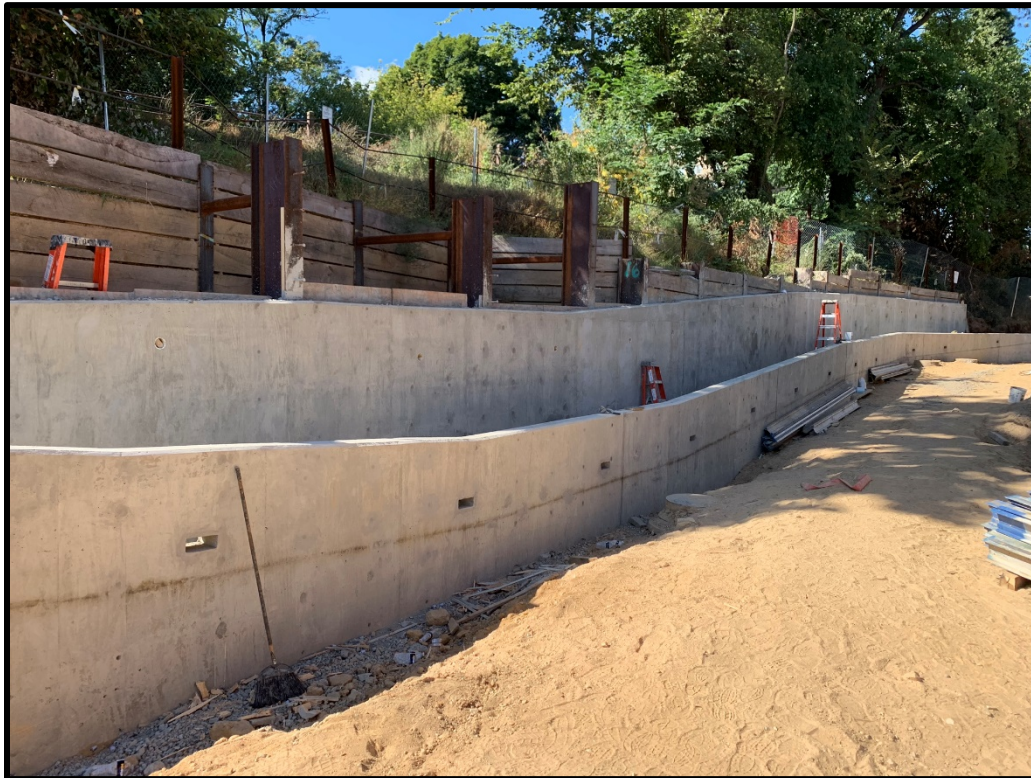
View of Site Walls on West Side of Project Site
