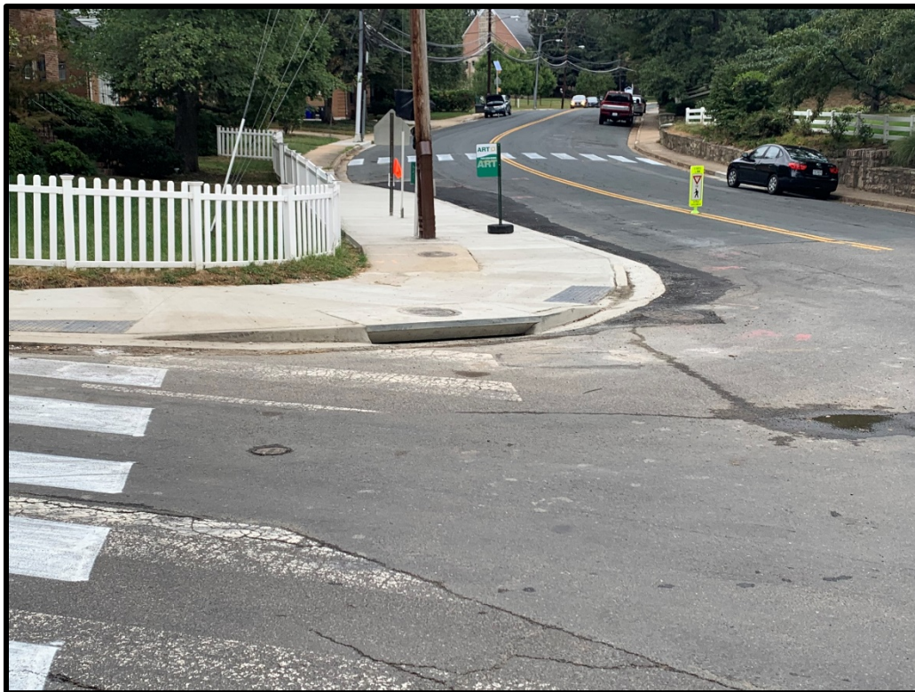
View of New Curb Bump Out and ADA Access
