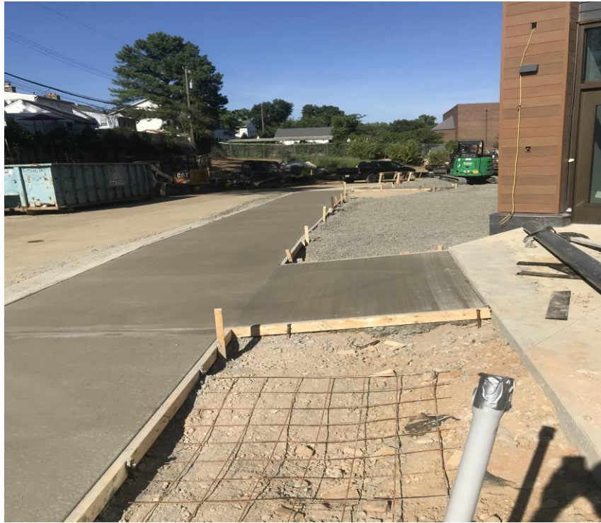
INSTALLATION OF BUS LOOP PEDESTRIAN SIDEWALK
