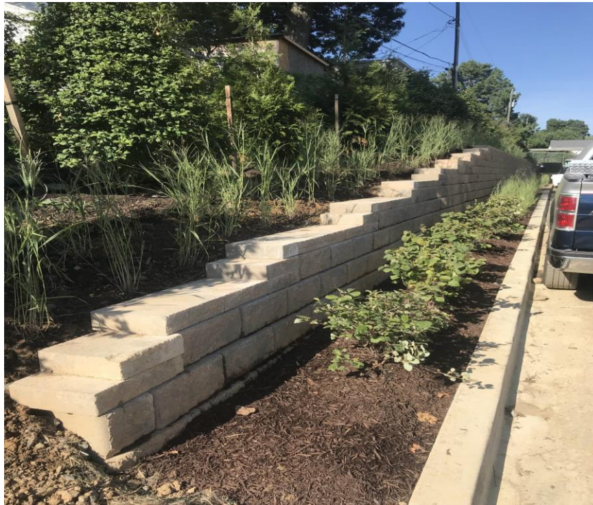
LANDSCAPING AND RETAINING WALL ALONG NORTH PROPERTY LINE
