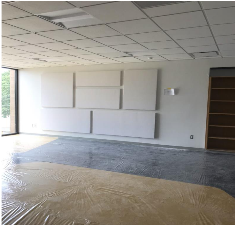
MUSIC ROOMS COMPLETE AND CARPET PROTECTION IN PLACE
