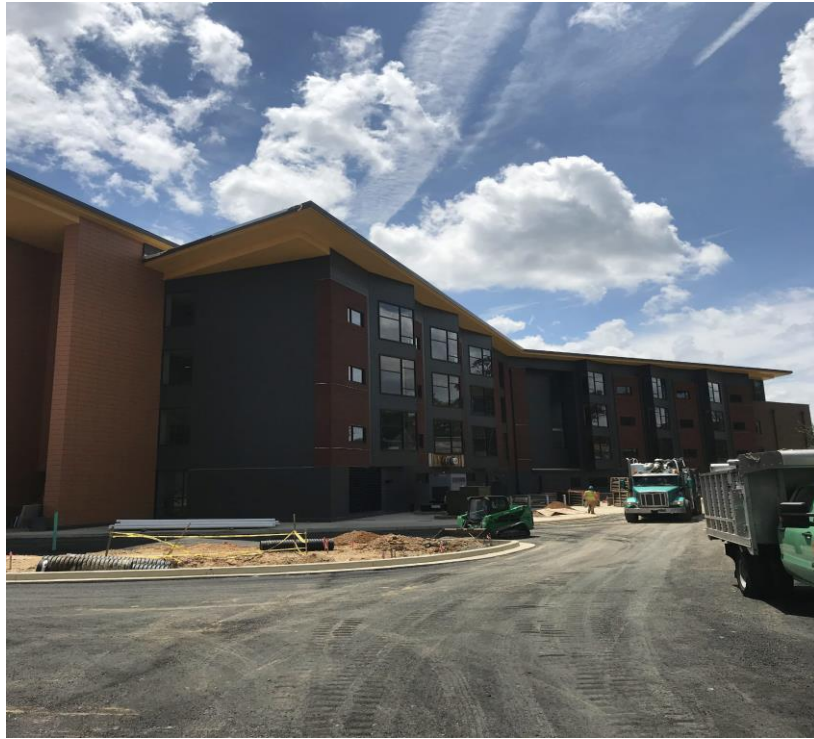
NORTH FAÇADE COMPLETION AND BUS LOOP COMPACTED STONE SUBGRADE
