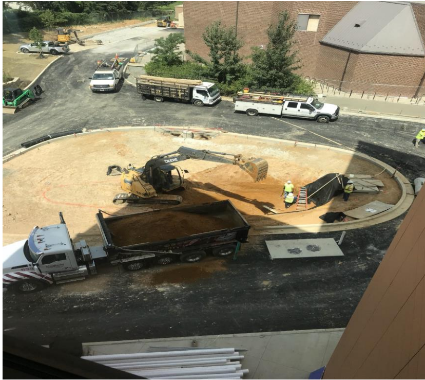
BUS LOOP BIO-RETENTION AREA EXCAVATION
