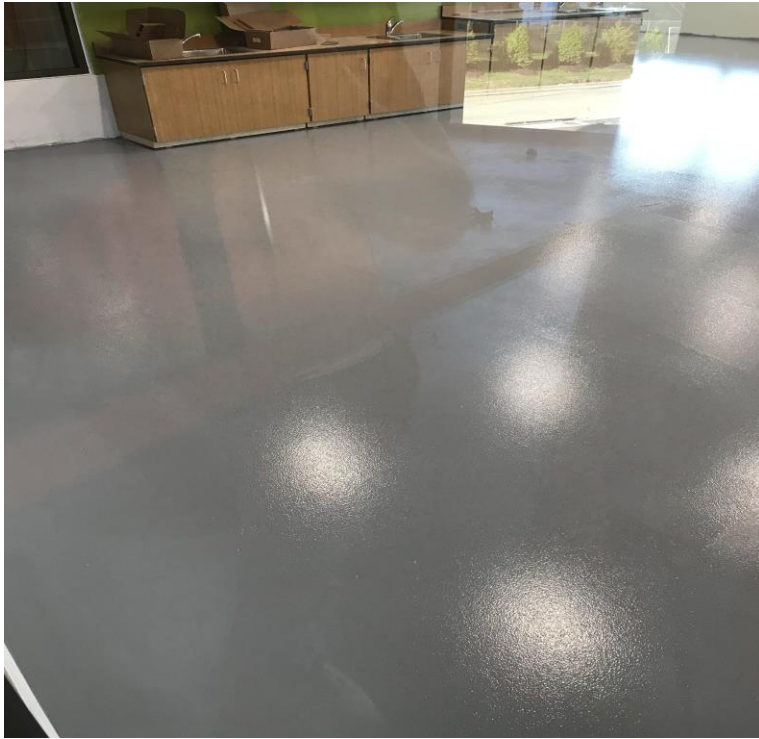
ART ROOM EPOXY COATED FLOORING IN PLACE
