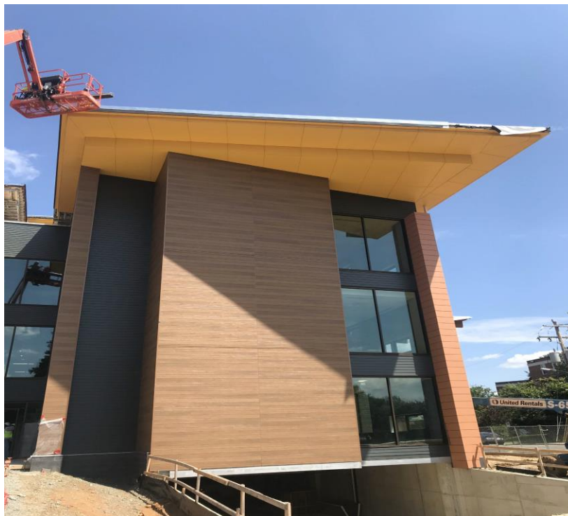
SOFFIT AND FASCIA INSTALLATION AT FAÇADE OVER GARAGE ENTRY RAMP
