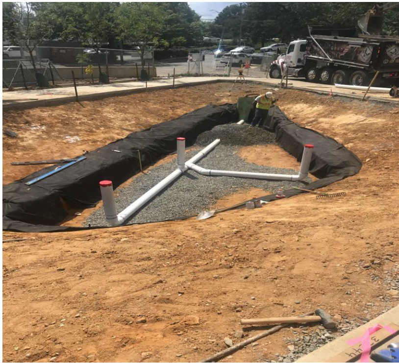
BIO-RETENTION AREA IN PROGRESS AT BUS LOOP ENTRY
