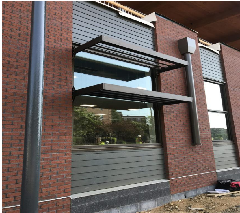
SUNSHADES INSTALLED ON WEST FACADE
