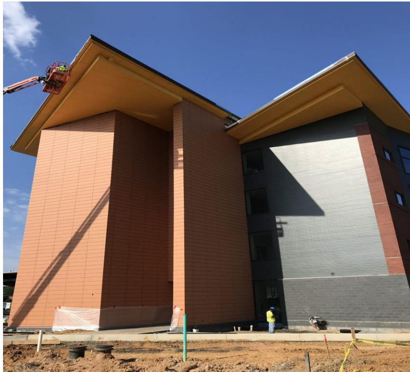
EAST FAÇADE COMPLETION
