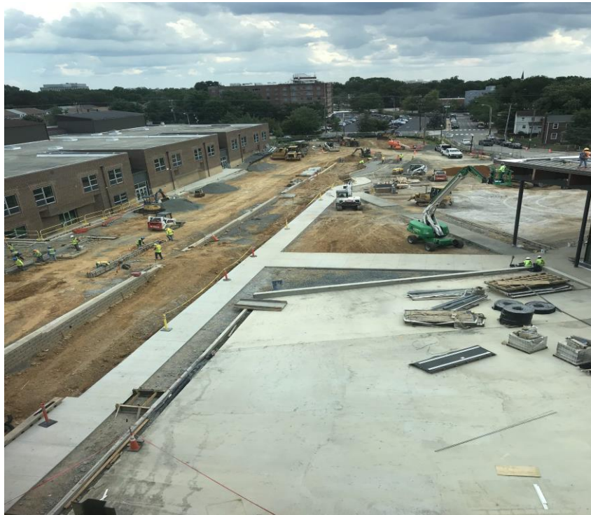
CONSTRUCTION OF GRADE 1 – 5 PLAY AREAS
