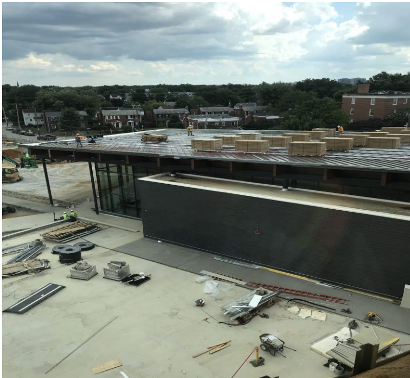
SOLAR PANEL INSTALLATION OVER GYM STANDING SEAM METAL ROOFING
