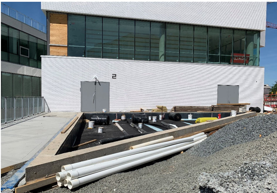
Starting Wilson Blvd hardscape
