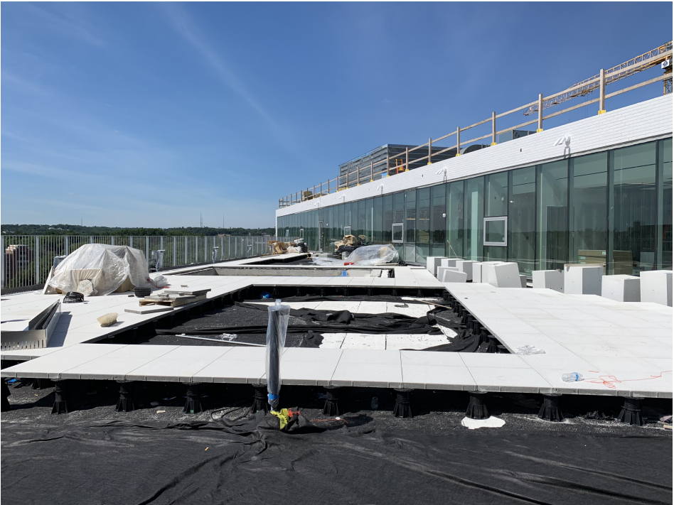
Terraces with pavers and planting soil
