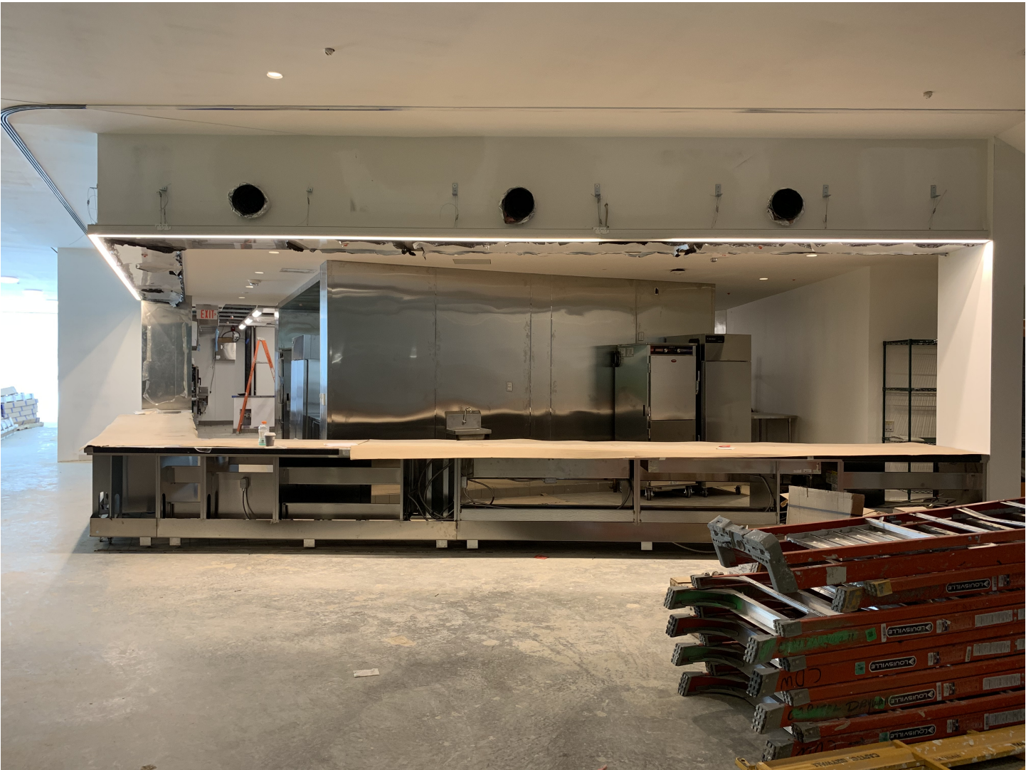
Cafeteria counter installed
