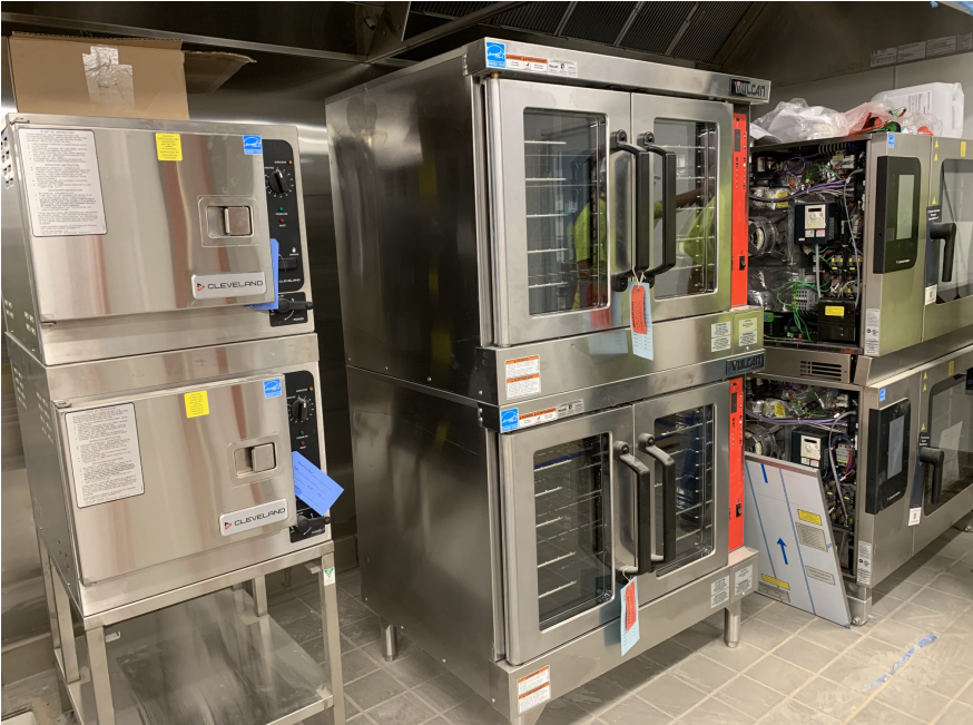
Kitchen equipment delivered
