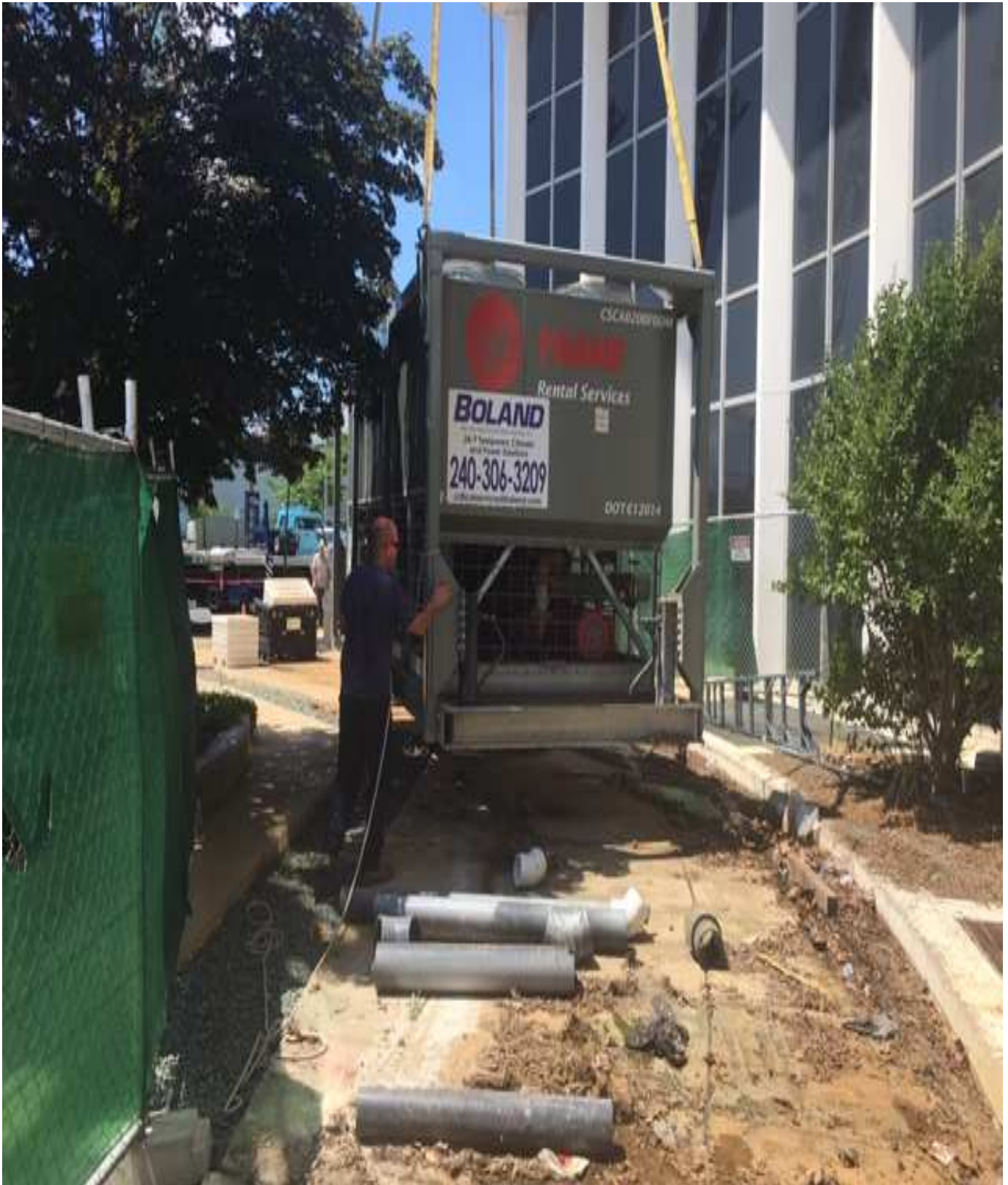
Planetarium Temporary existing chiller removal
