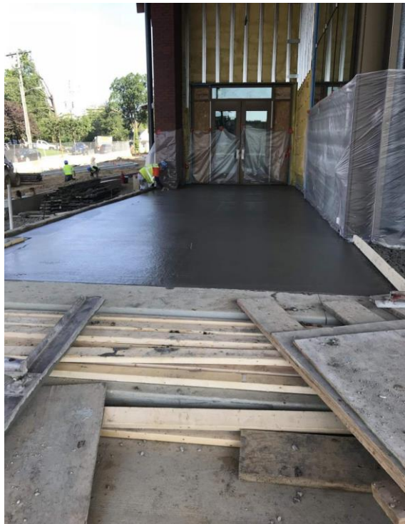
SITE SIDEWALK OUTSIDE OF THE GYM IN PROGRESS
