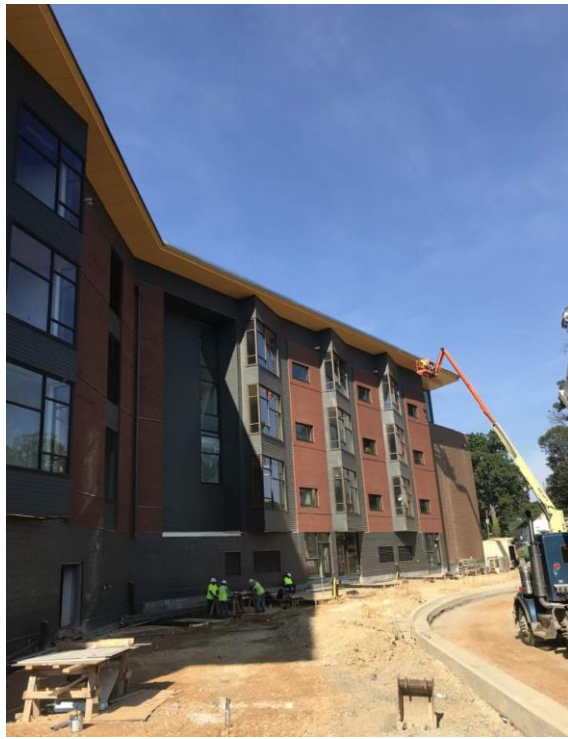
NORTH FAÇADE NEARING COMPLETION
