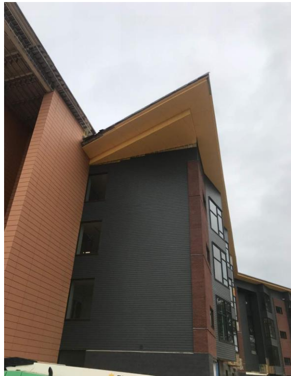
SOFFIT AND FASCIA INSTALLATION AT NORTH FACADE
