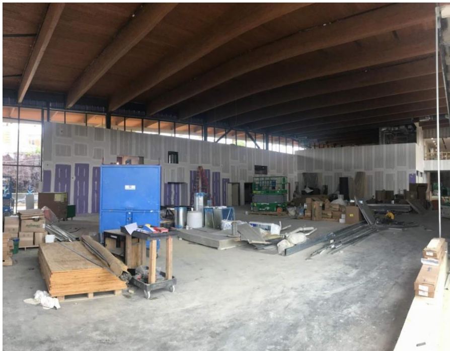
PROGRESS AT GYMNASIUM
