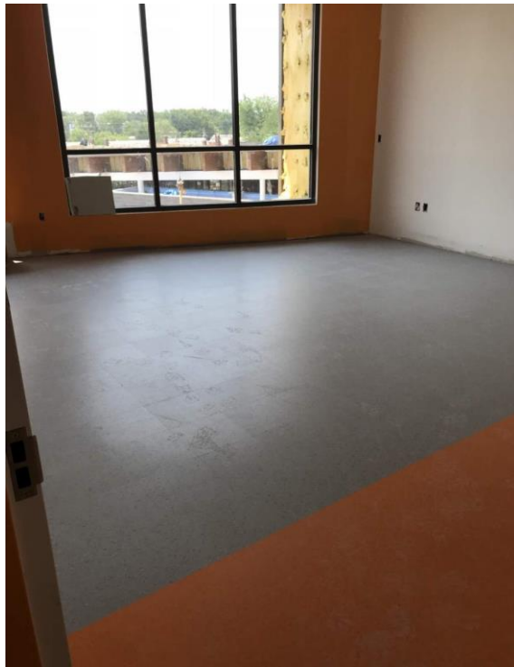
FLOOR TILE COMPLETE AT 3 RD FLOOR CLASSROOMS
