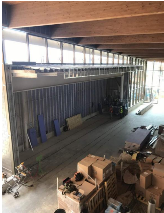
FRAMING OF STAGE WITHIN GYMNASIUM
