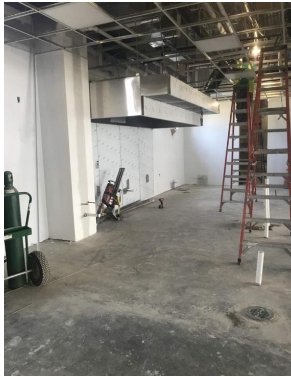
KITCHEN EXHAUST HOOD INSTALLED
