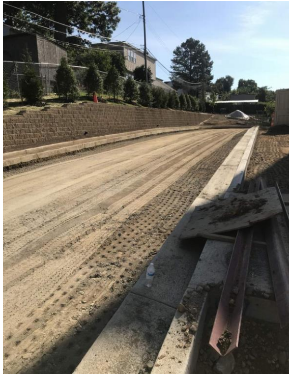
BUS LOOP CURB AND GUTTER IN PLACE
