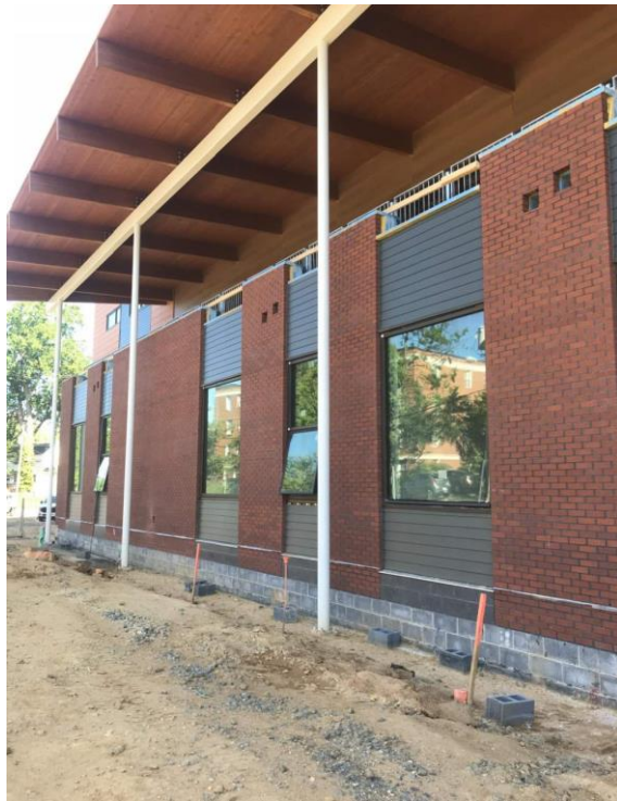
WEST FAÇADE PROGRESS
