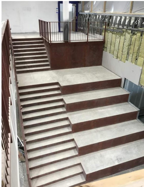
STORY STAIR BETWEEN 3 RD AND 4 TH FLOORS
