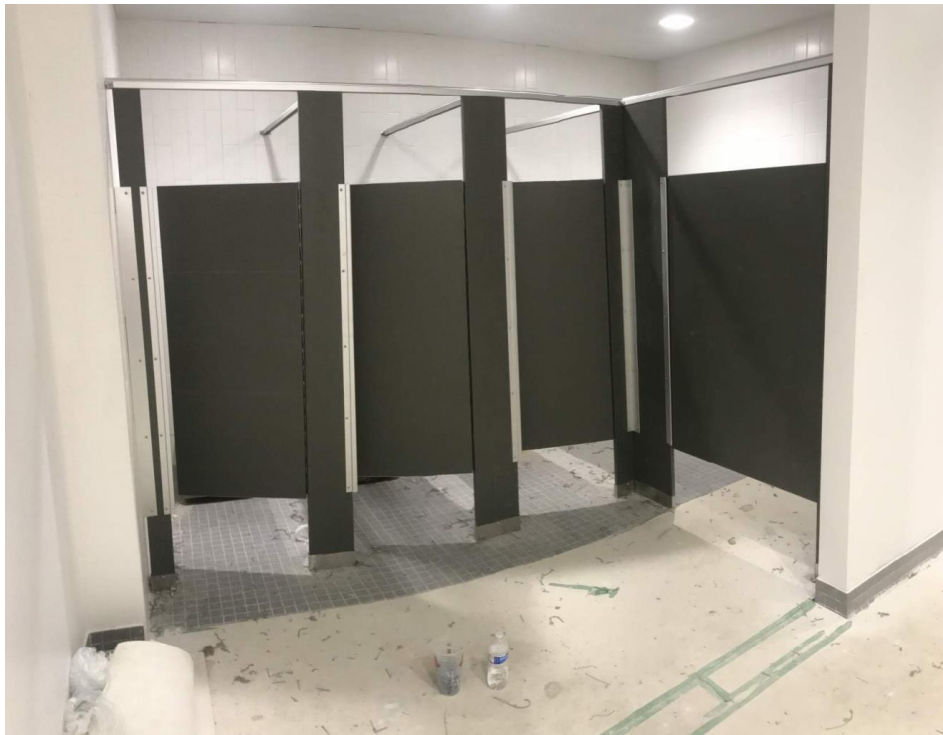
TOILET PARTITIONS SET IN 3 RD FLOOR STUDENT BATHROOM
