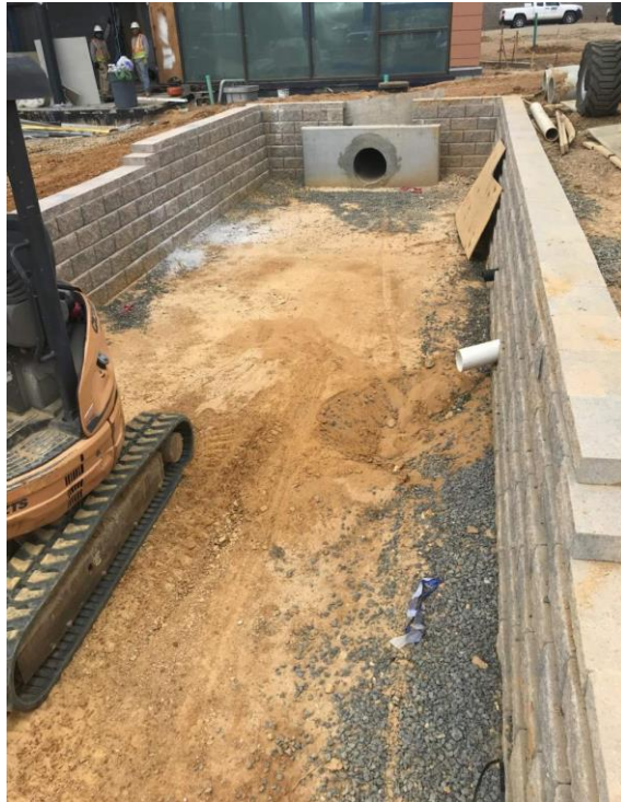
RETAINING WALL AND PIPING FOR BIO-SWALE IN PLACE
