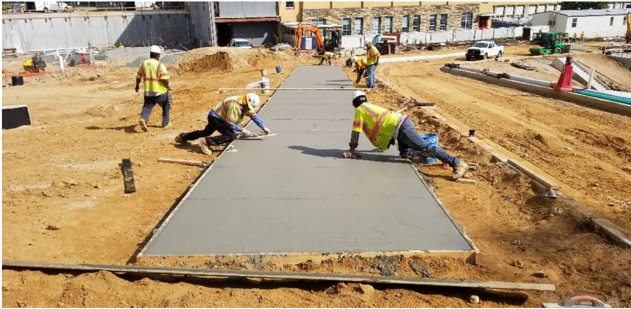
Sidewalk along Drop-Off road
