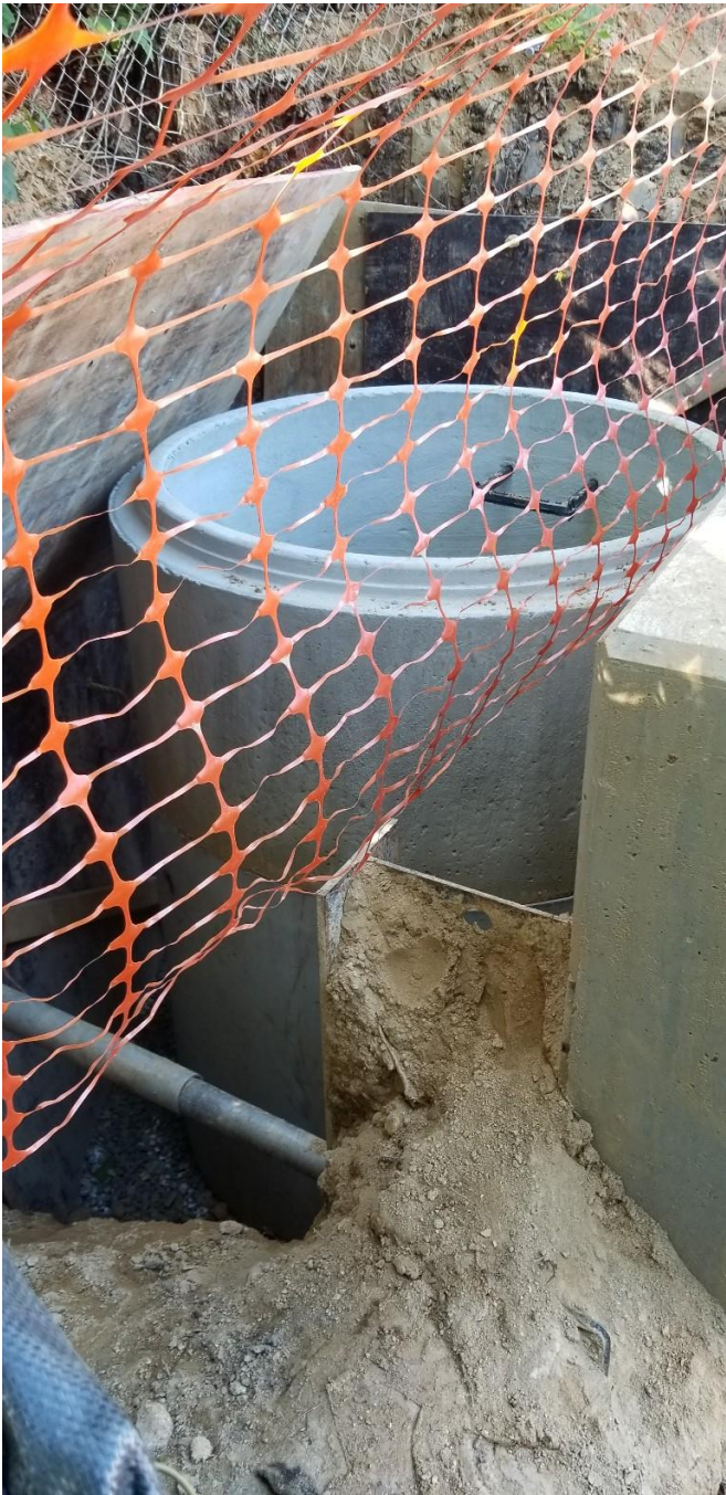
Site drainage near Vacation Lane behind retaining wall
