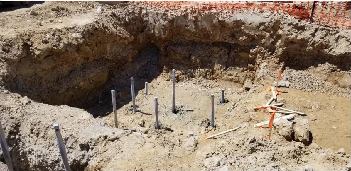
Pile foundation for addition
