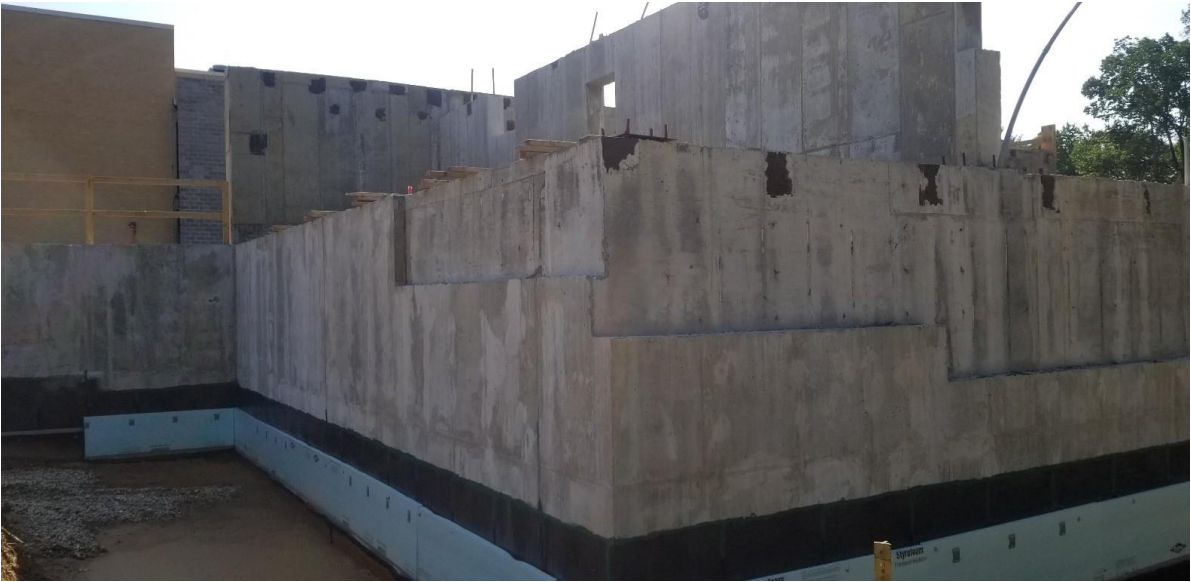
Exterior building waterproofing
