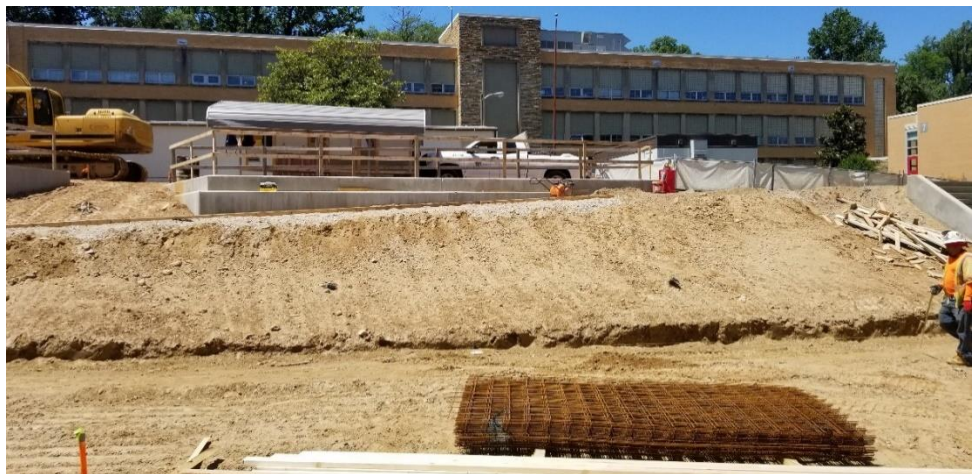
Various Field Hardscape Elements
