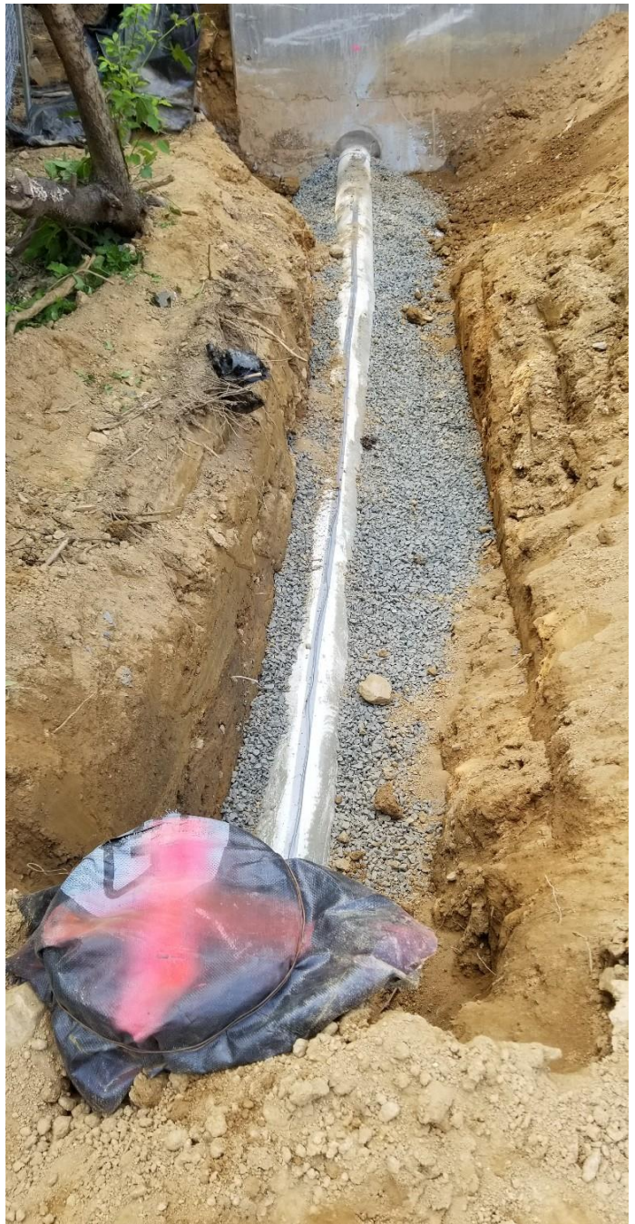
Site drainage near Vacation Lane behind retaining wall
