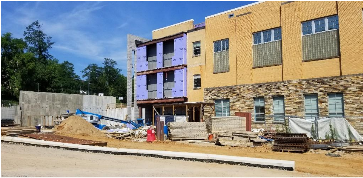
Prep work for new metal exterior fascia
