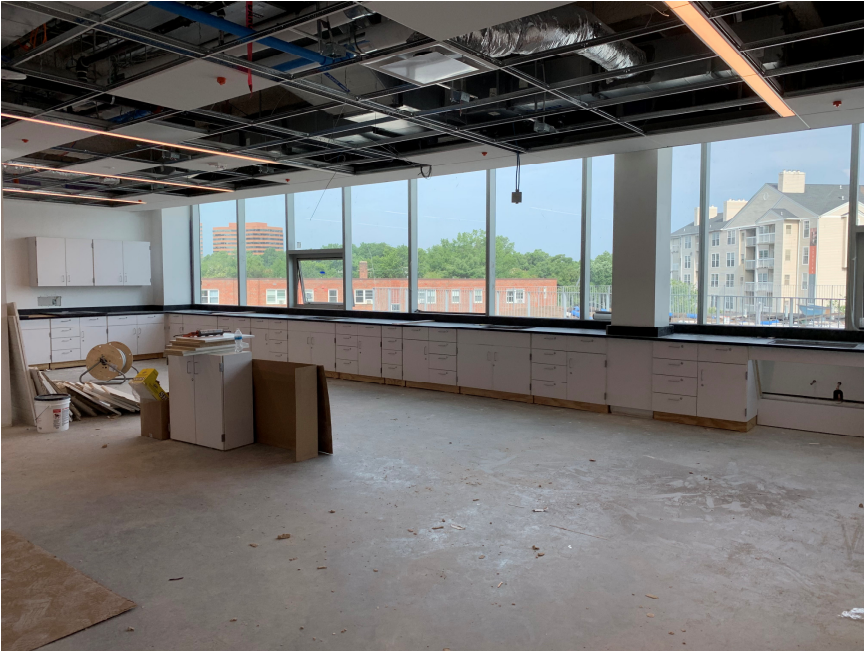
Lab cabinets installed at level 3
