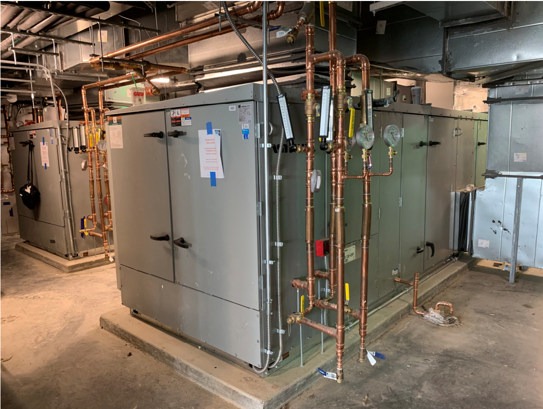
Mechanical systems installed and testing started
