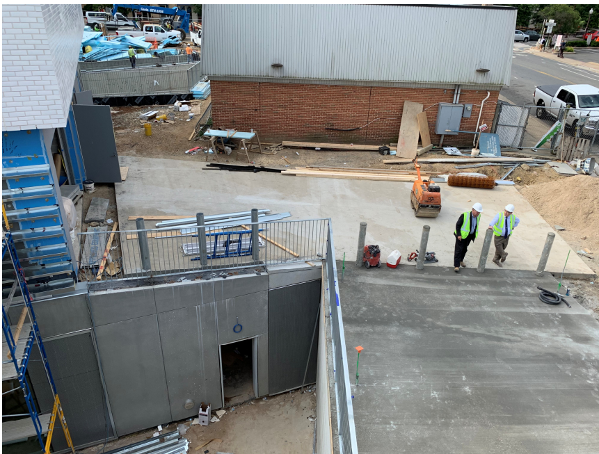
Concrete slab poured at loading dock
