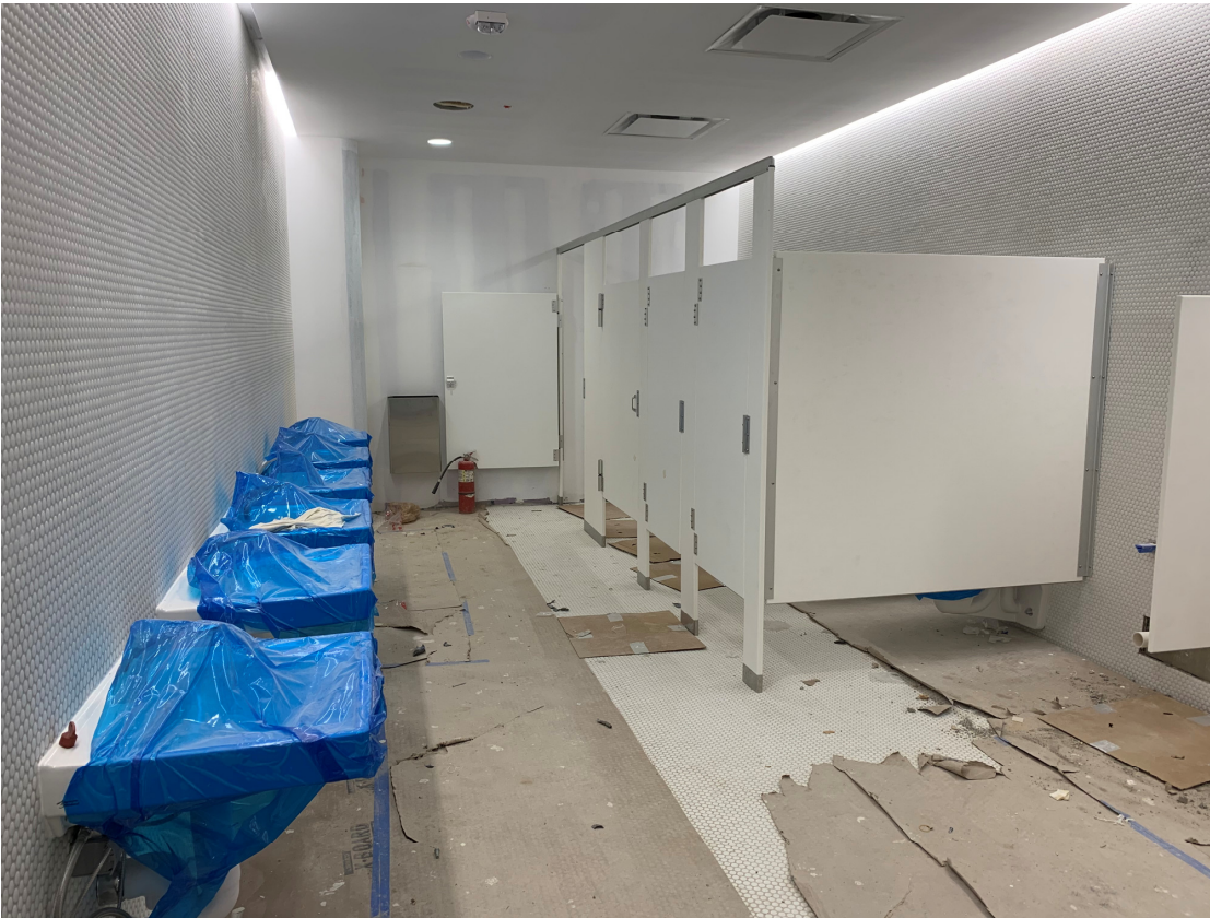
Sinks and partitions installed at gang bathroom
