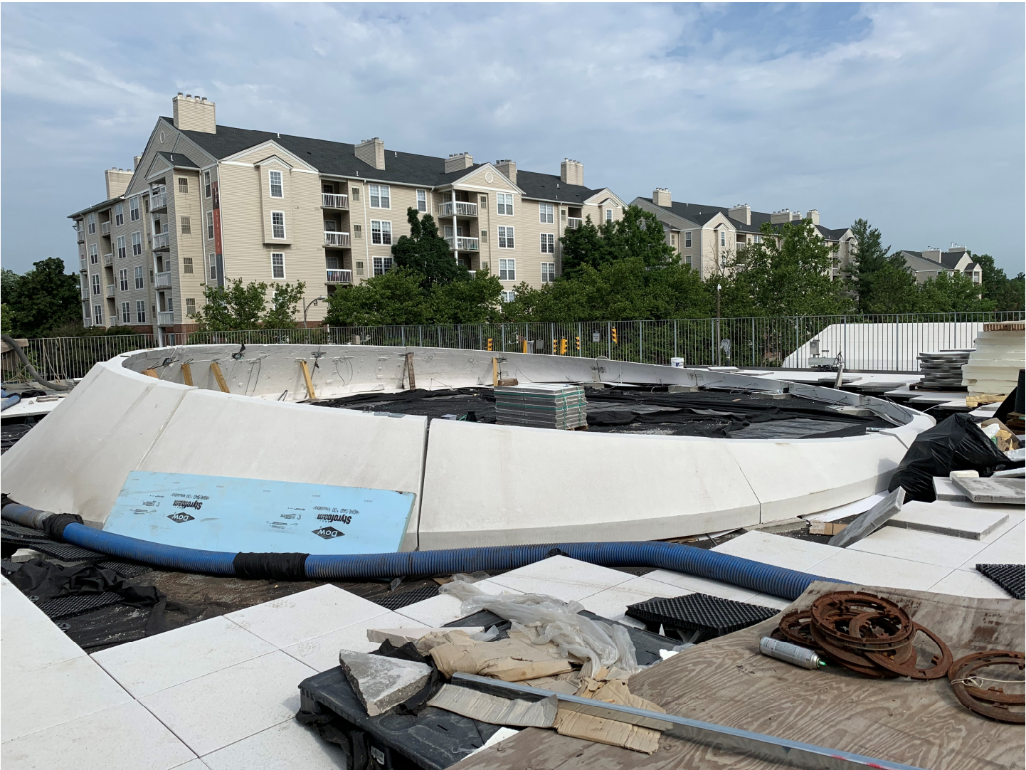
Precast planter box installed on main terrace
