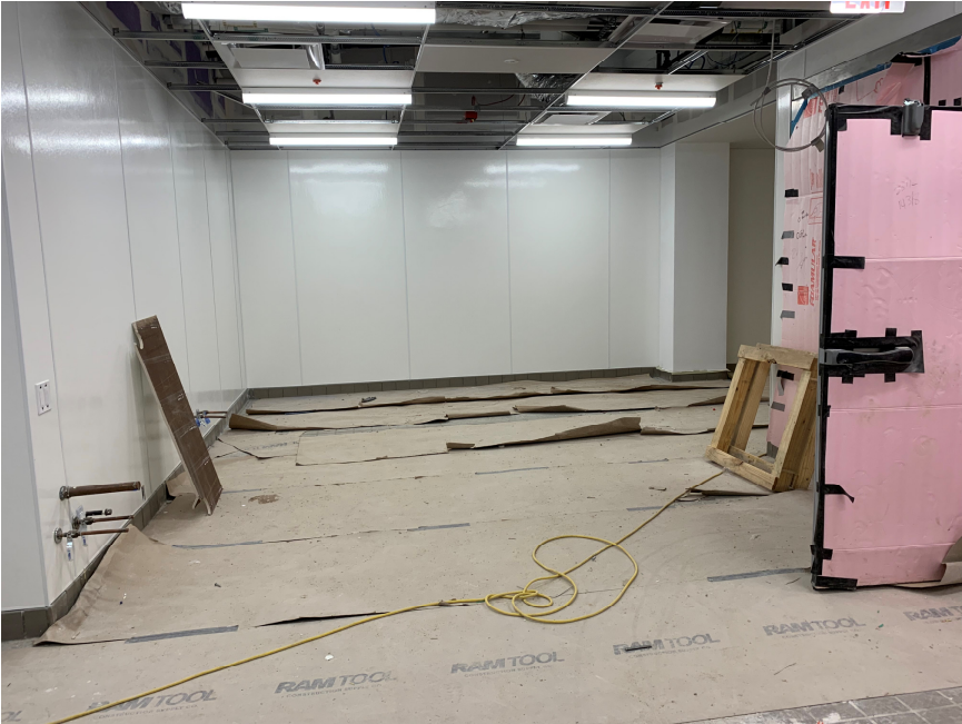
FRP panels installed at kitchen
