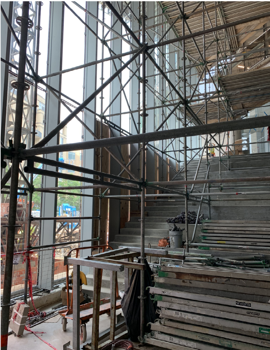
Entrance curtain wall installation started
