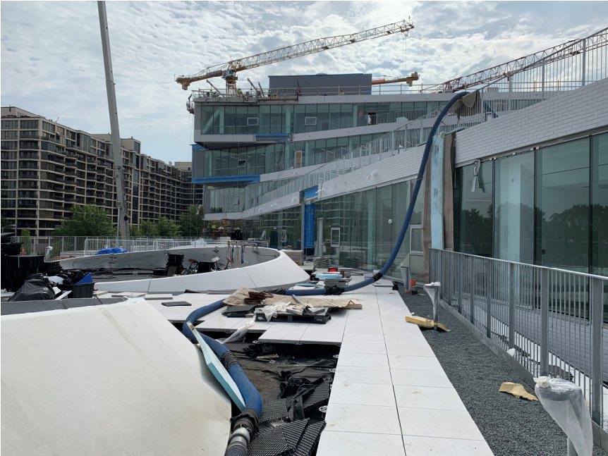
Precast planter box installed on main terrace
