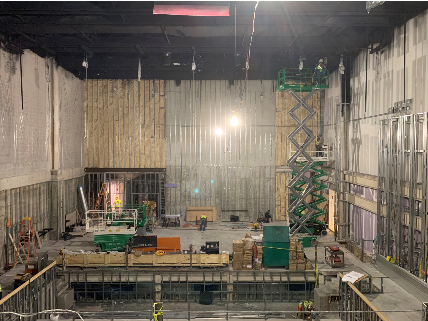
Framing installation at auditorium started
