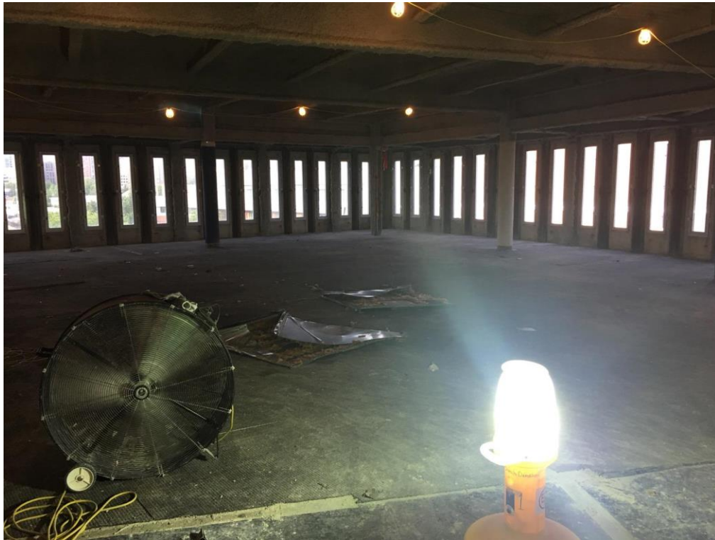
Demolition of 4 th floor Mechanical Room
