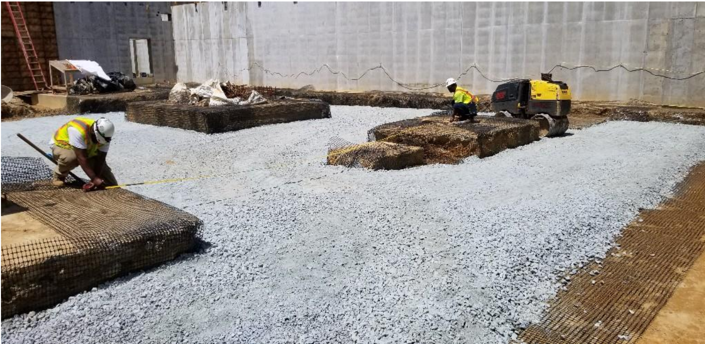
1 st floor slab on grade stabilization
