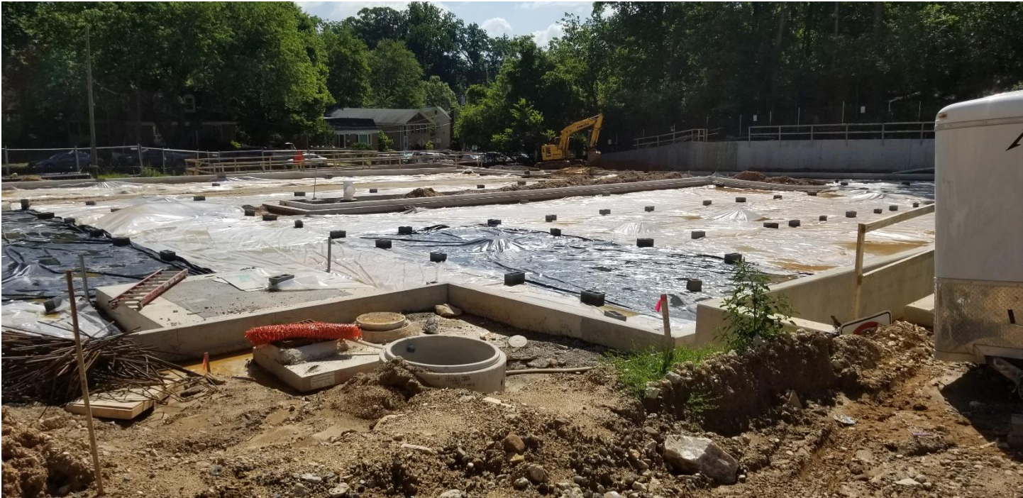
New Employee Parking lot
