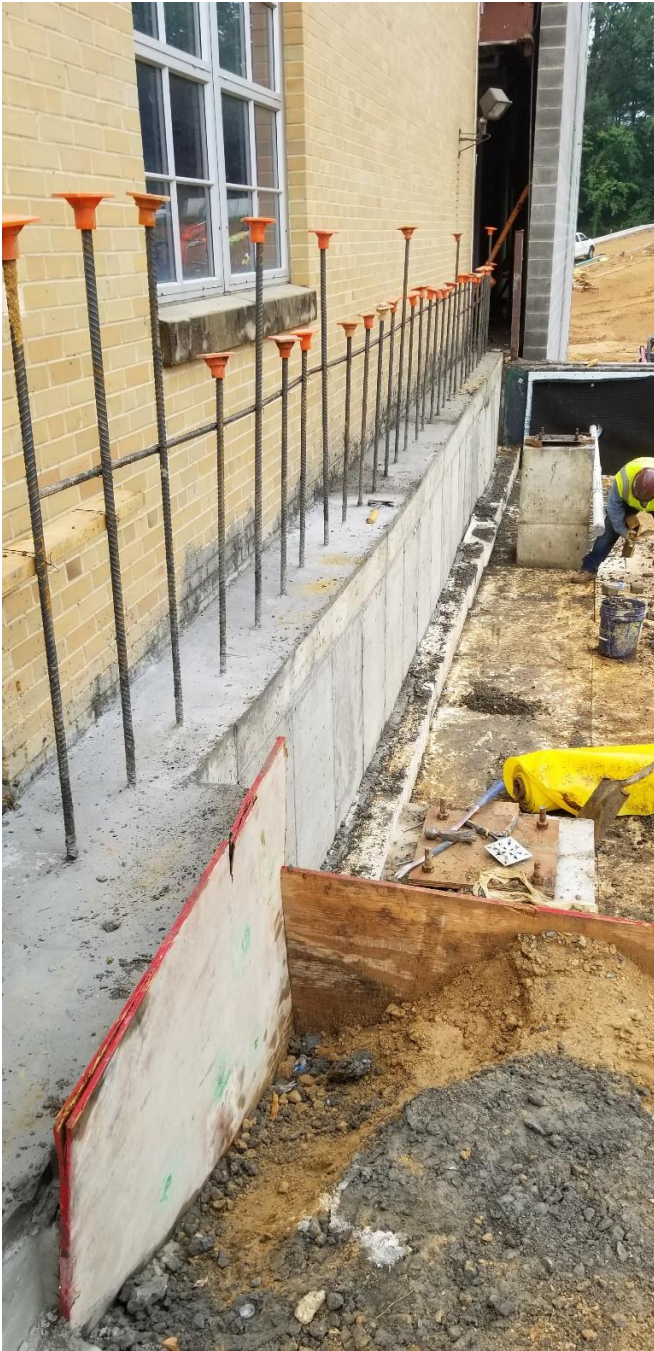
Structural beam to support masonry separation wall
