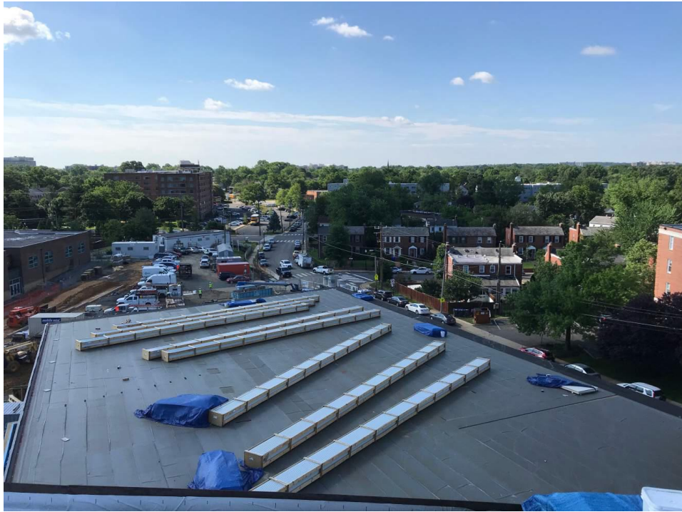
STANDING SEAM METAL PANEL ROOFING STOCKED AT GYM ROOF
