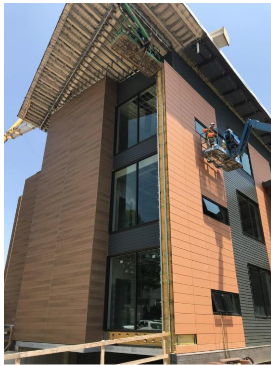
TERRACOTTA CLADDING IN PROGRESS NEXT TO COMPLETED FIBER CEMENT SIDING
