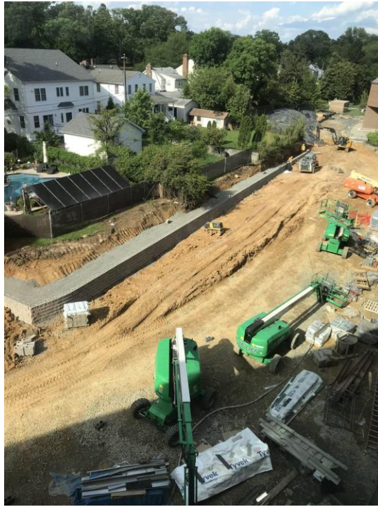
COMPLETED SITE RETAINING WALL AT NORTH SIDE PROPERTY LINE
