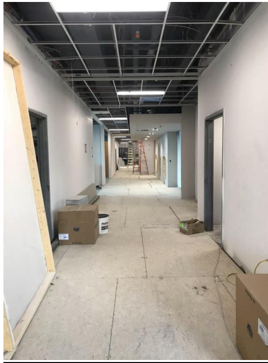
PROGRESS AT 3 RD FLOOR HALLWAY
