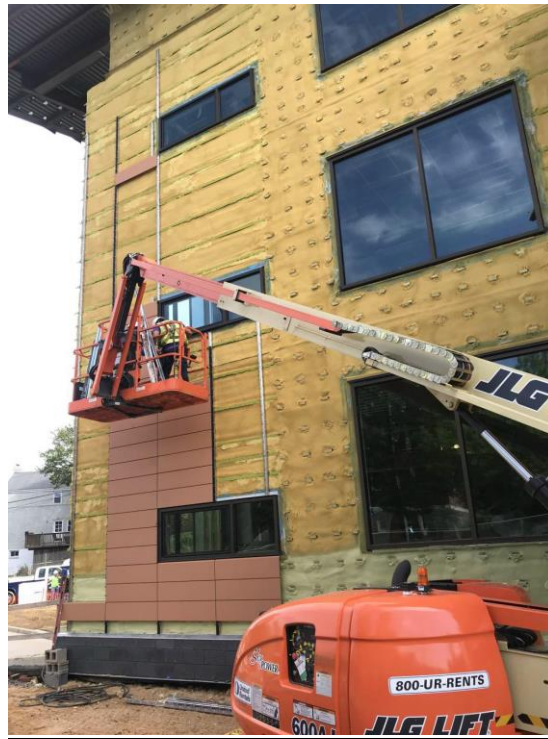
INSTALL OF TERRACOTTA CLADDING PANELS OVER SPRAY FOAM INSULATION
