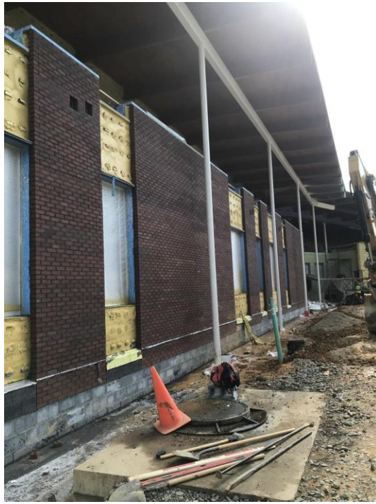
MASONRY VENEER INSTALLED AT WEST FACADE
