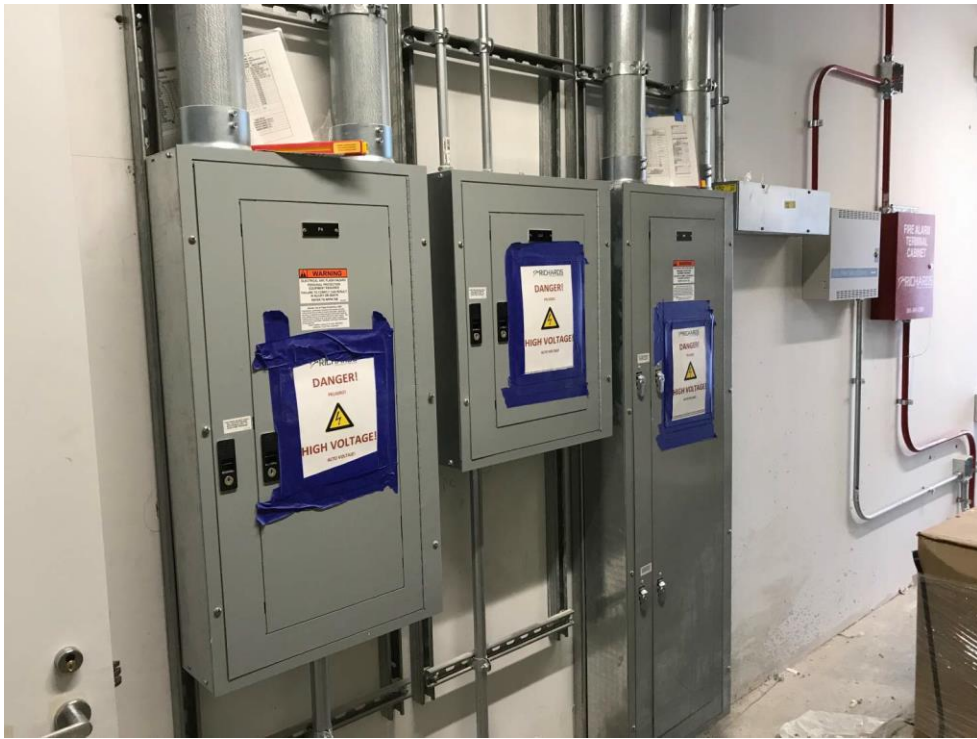
PROGRESS OF TYPICAL ELECTRICAL DISTRIBUTION ROOM
