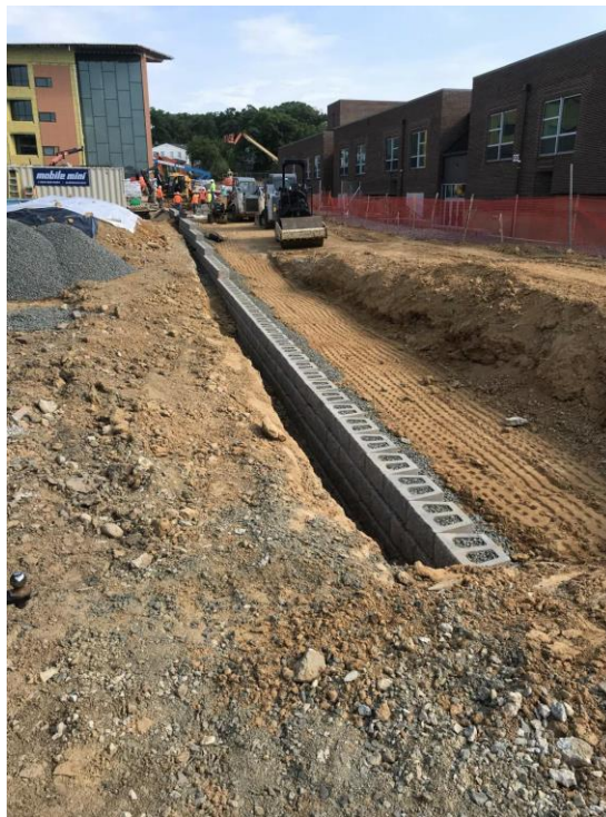
SITE RETAINING WALL ADJACENT TO TJMS IN PROGRESS
