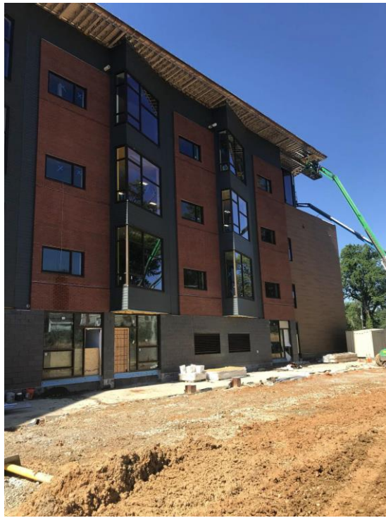
EXTERIOR CLADDING PROGRESS AT NORTH FAÇADE
