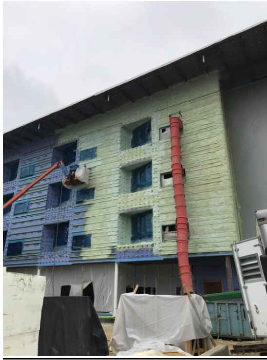
LAST SECTION OF EXTERIOR SPRAY FOAM INSULATION BEING COMPLETED
