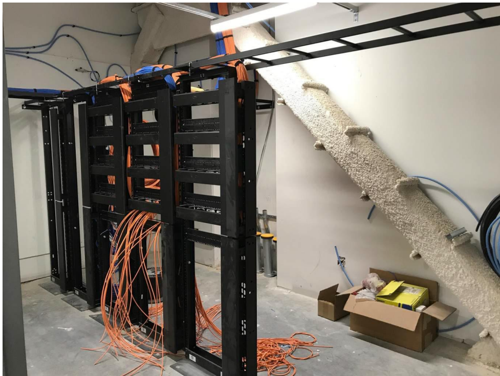
PROGRESS AT MAIN COMMUNICATIONS CLOSET
