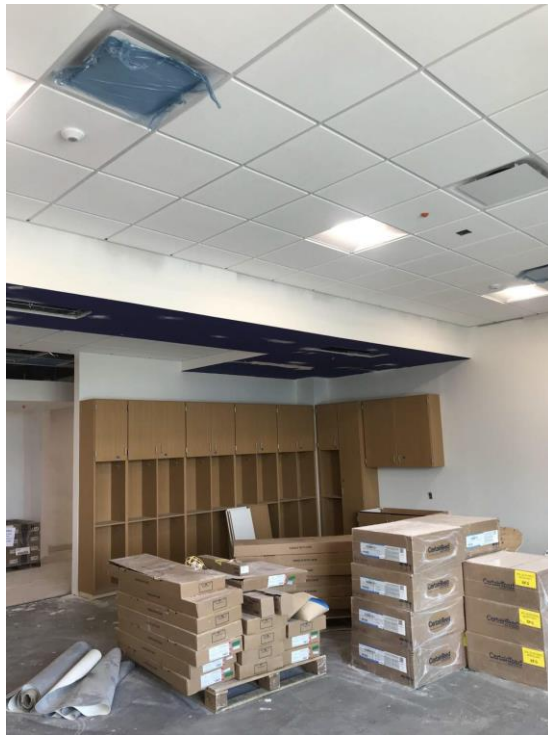
CASEWORK AND FINISHED CEILINGS AT 4 TH FLOOR CLASSROOM
