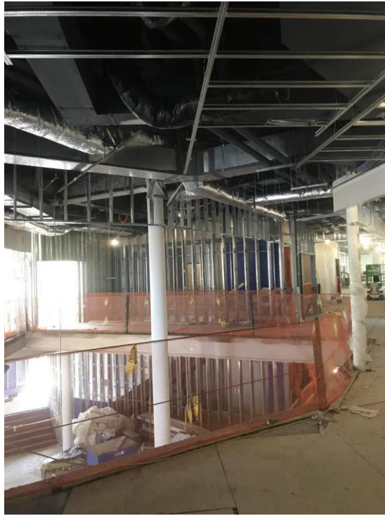
WALL AND CEILING FRAMING AT 2 ND FLOOR HUB
