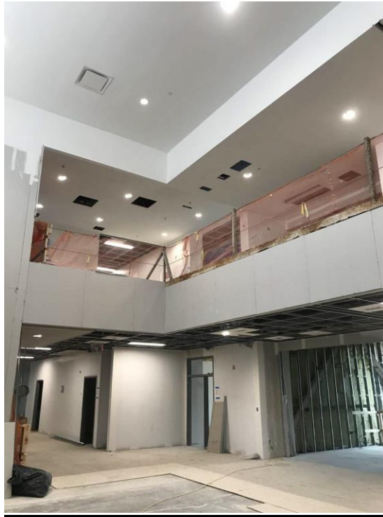
OPEN ATRIUM BETWEEN FLOORS 3 AND 4
