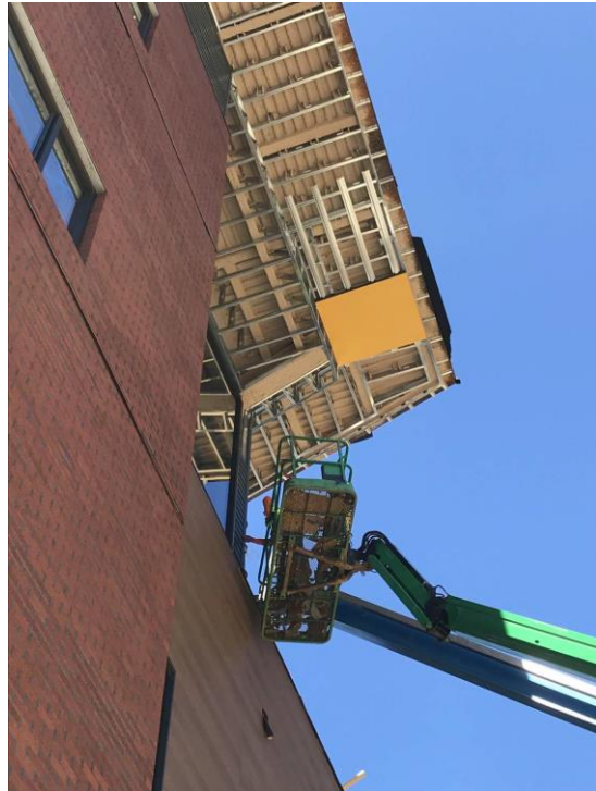
START OF SOFFIT INSTALL AT NORTH SIDE
