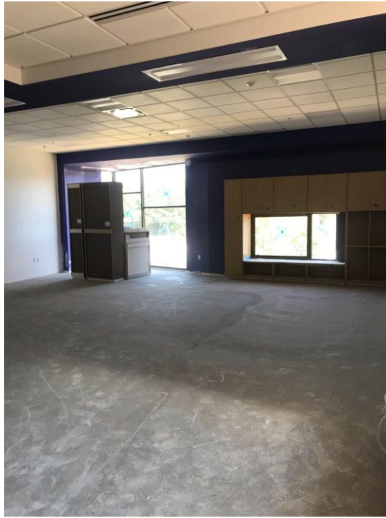
4 TH FLOOR CLASSROOM PREPARED FOR FLOOR TILE
