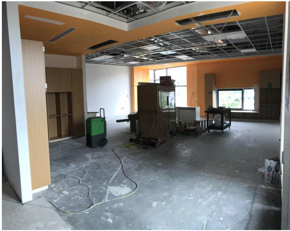
FINISH PAINT, CASEWORK, AND CEILING AT 3 RD FLOOR CLASSROOM
