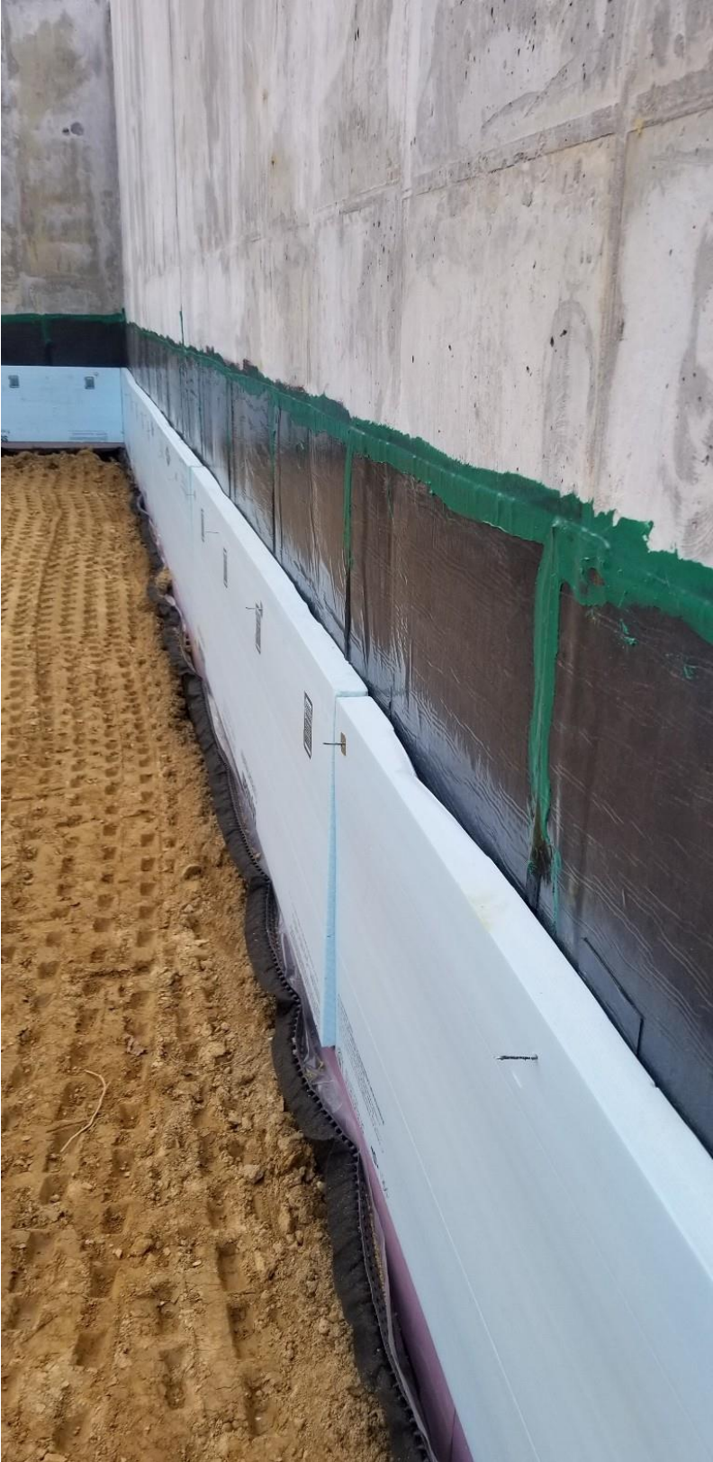
Waterproofing main retaining wall between levels 1 & 2
