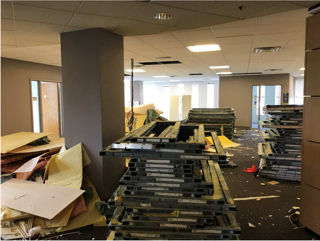
Demolition of systems furniture and separation of materials for recycling.
