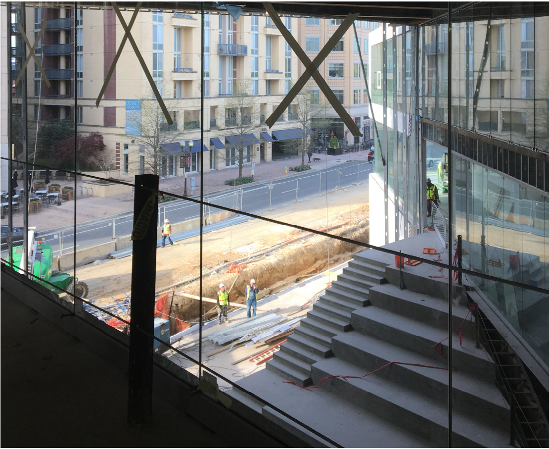
Prep work for three story curtainwall along Wilson Blvd
