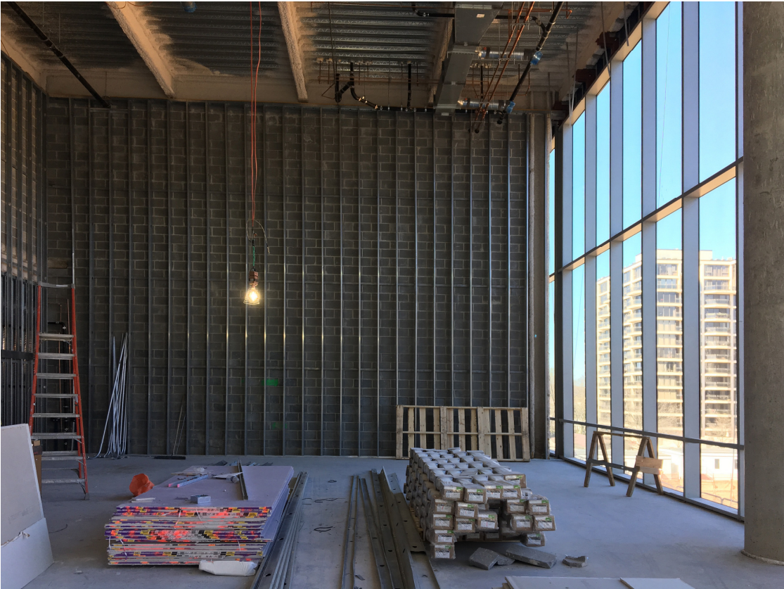
CMU wall installed between music rooms
