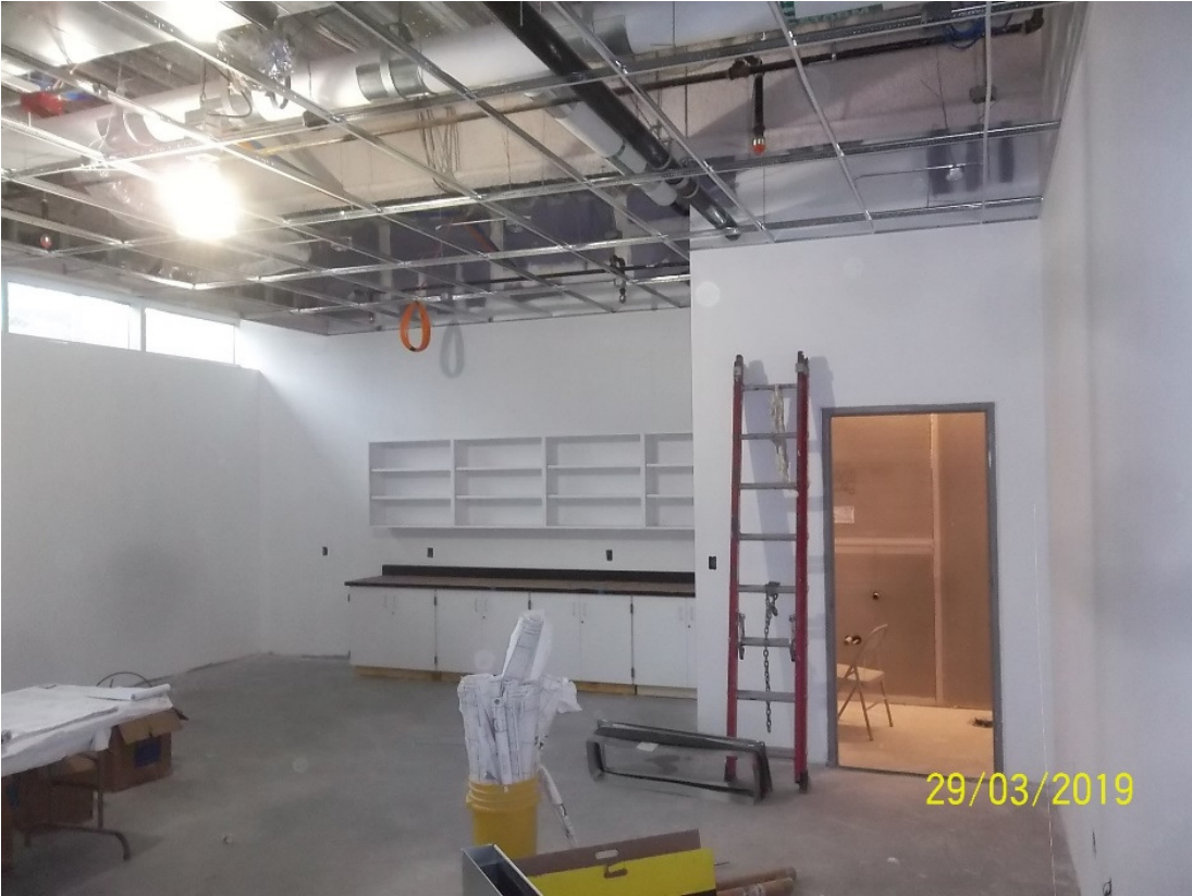
Casework and ceiling grid installation at G1 classrooms
