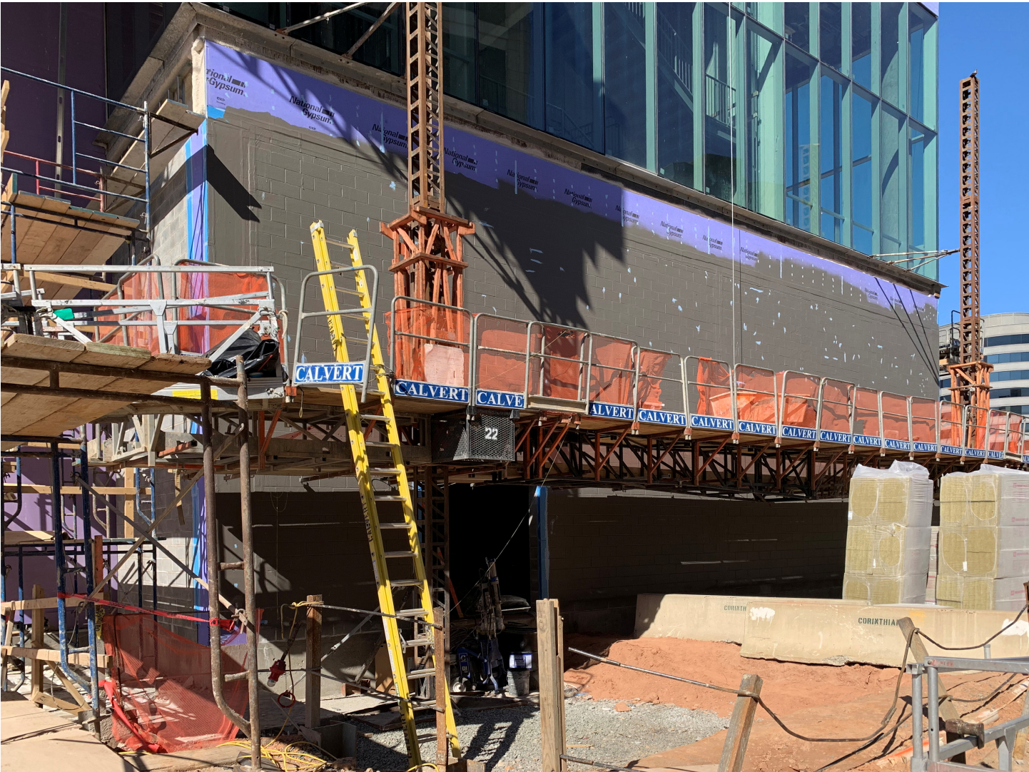
Installation of vapor barrier and brick rainscreen started at south facade
