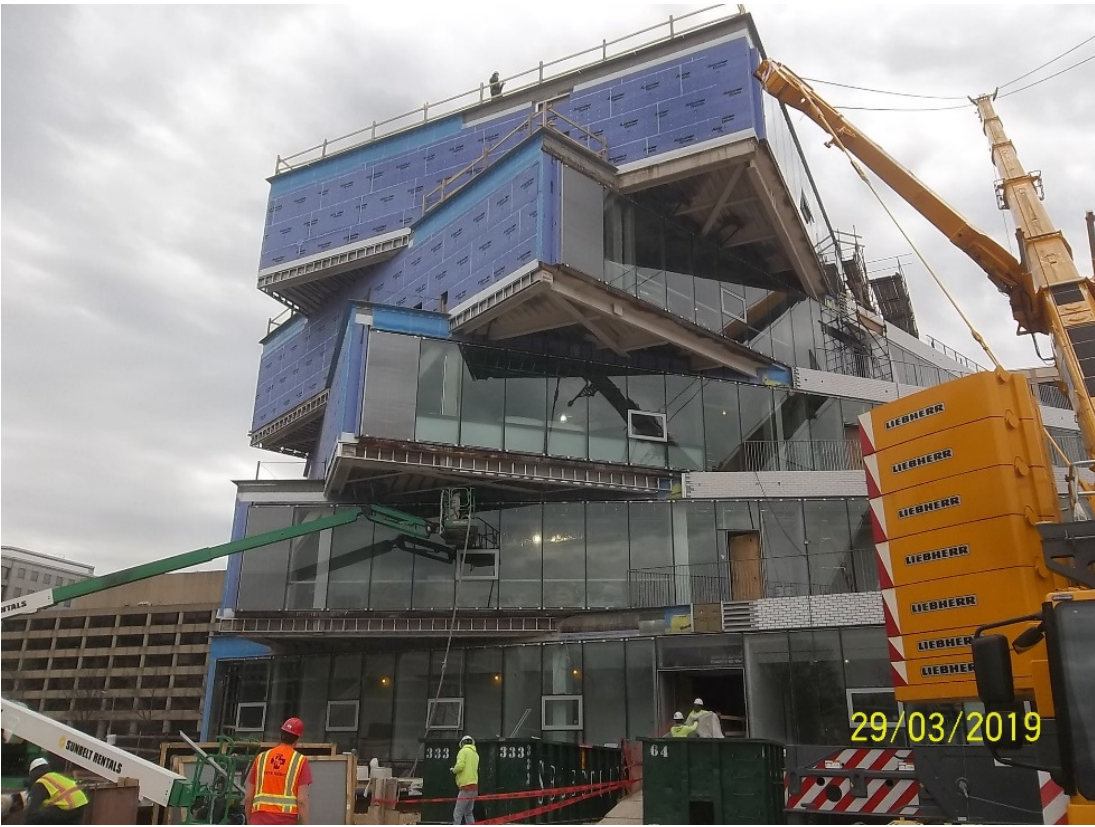
View from 18 th Street
