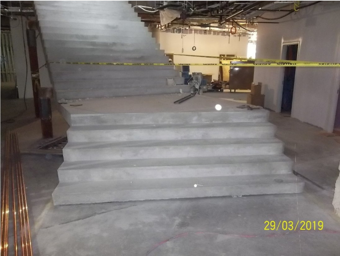
Interior cascading stair at level 3
