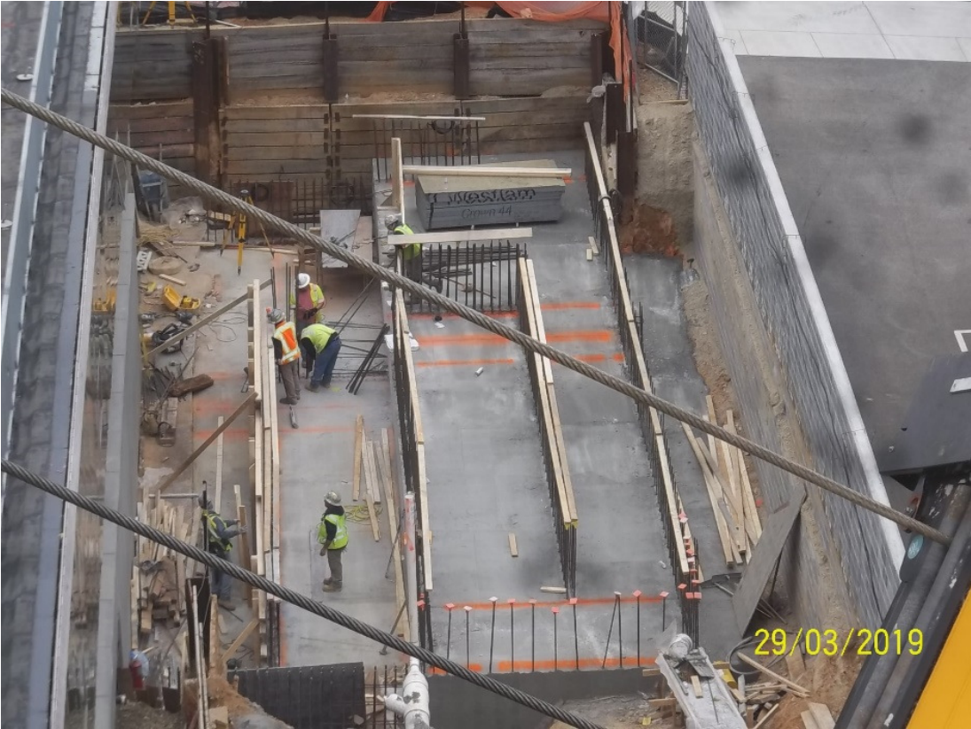
Construction of NW Entrance Stair/Ramp
