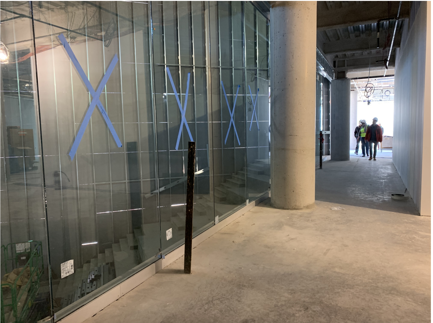
Interior curtain wall installed at level 2
