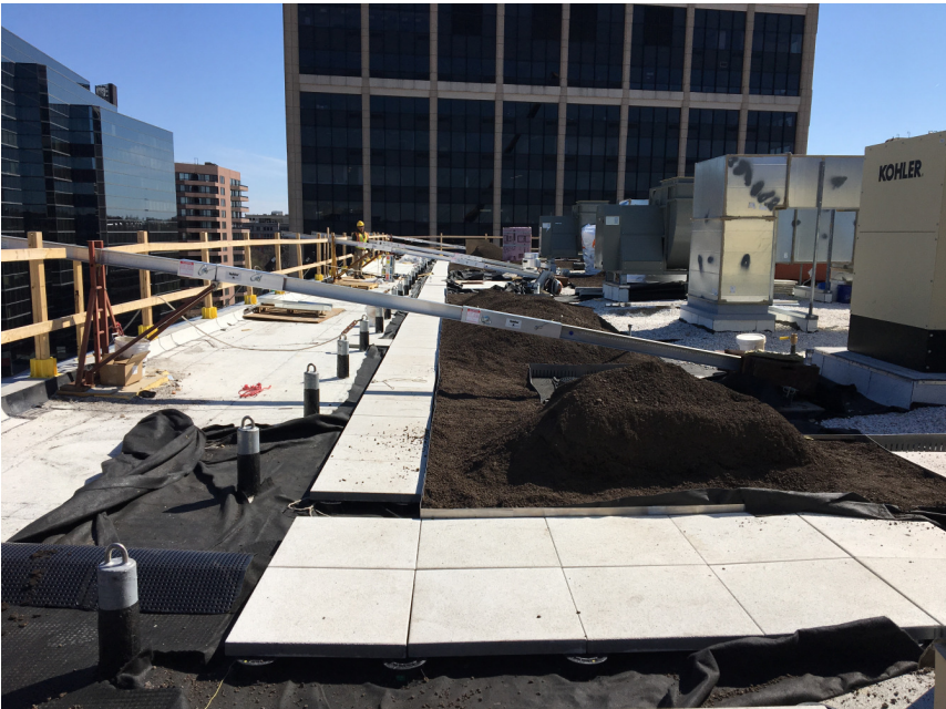
Roof pavers installed at level 5
