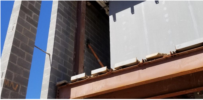
12-hour CMU temporary bracing until Precast units is installed
