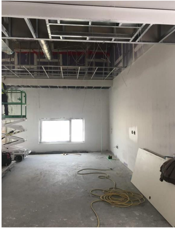
PRIME PAINTING OF CLASSROOM SPACES ON 4 TH FLOOR
