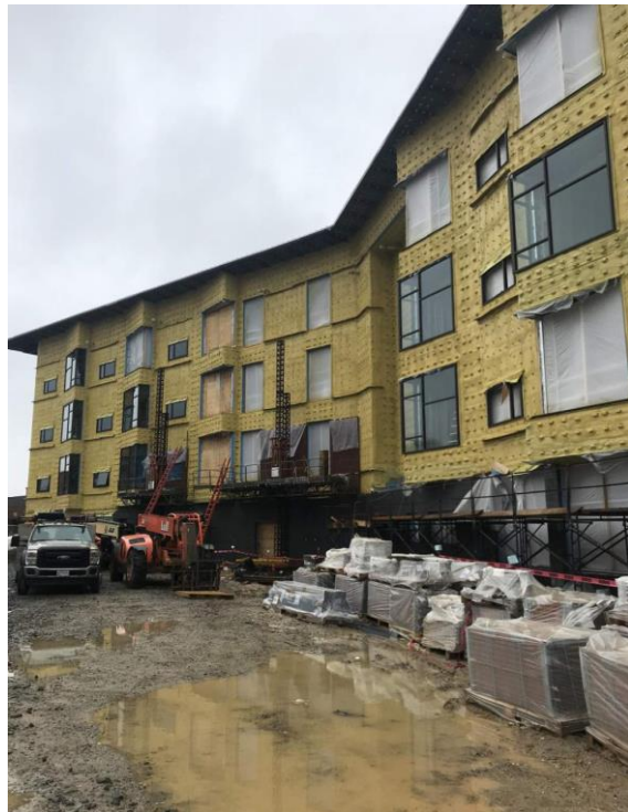
OVERALL PROGRESS OF NORTH SIDE FAÇADE
