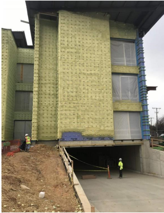
INSTALLED SPRAY FOAM/AIR BARRIER ON FAÇADE ABOVE GARAGE ENTRY
