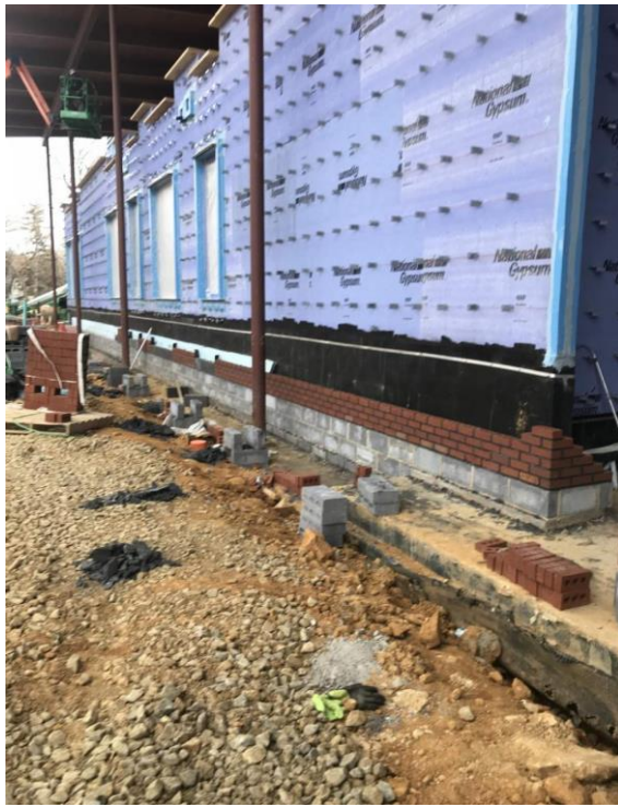
COMMENCEMENT OF MASONRY VENEER INSTALLATION AT WEST SIDE FACADE
