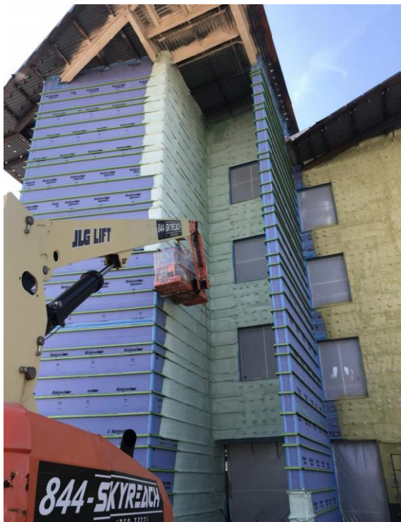
INSTALLATION OF SPRAY FOAM/AIR BARRIER ON EAST SIDE OF BUILDING
