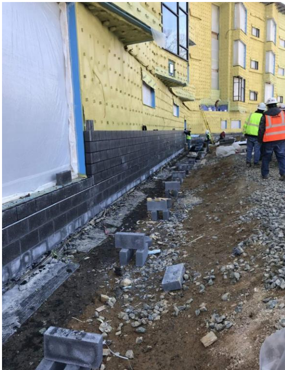
INSTALLATION OF MASONRY VENEER AT NORTH SIDE FACADE
