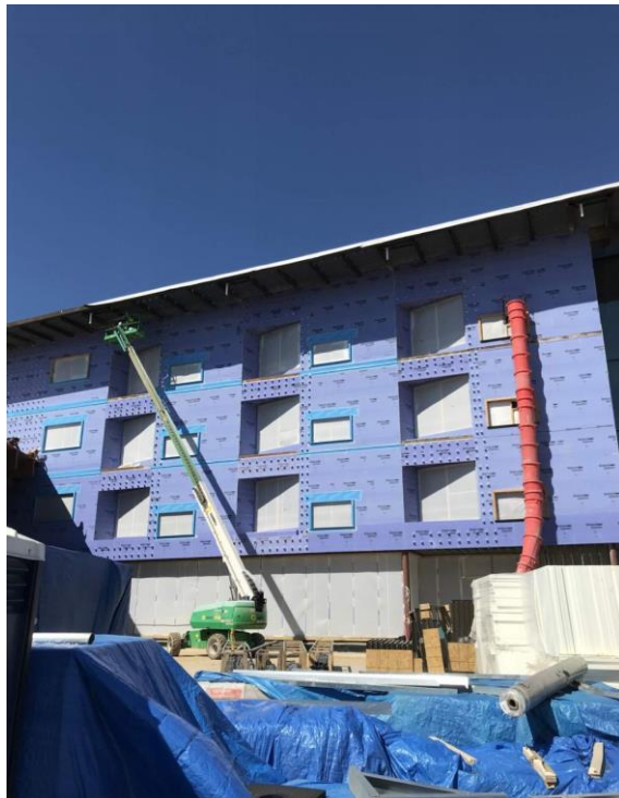
PROGRESS AT EXTERIOR FAÇADE ON SOUTH SIDE OF BUILDING
