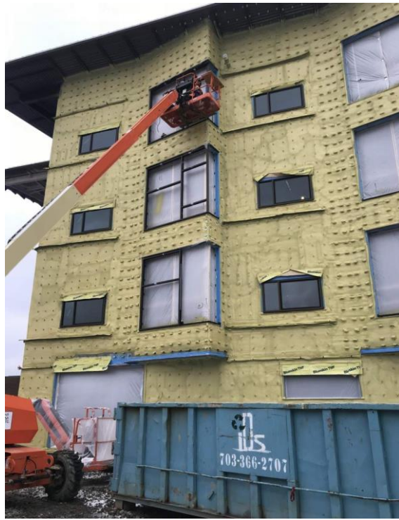
INSTALLATION OF WINDOWS AT NORTH SIDE FAÇADE
