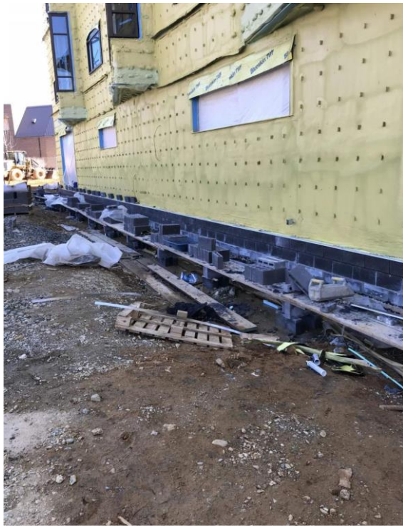
COMMENCEMENT OF MASONRY VENEER INSTALLATION AT NORTH SIDE FACADE
