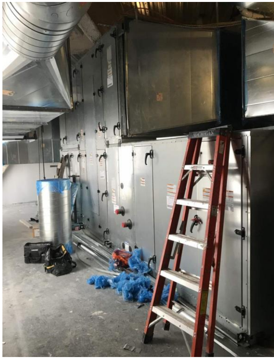
CENTRAL BUILDING OUTSIDE AIR UNIT SET
