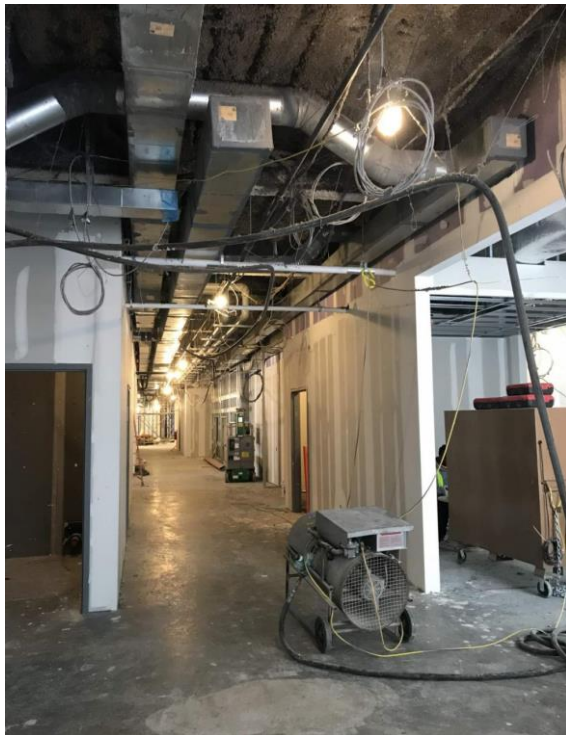
PROGRESS OF WALL CLOSE-INS ON 2 ND FLOOR
