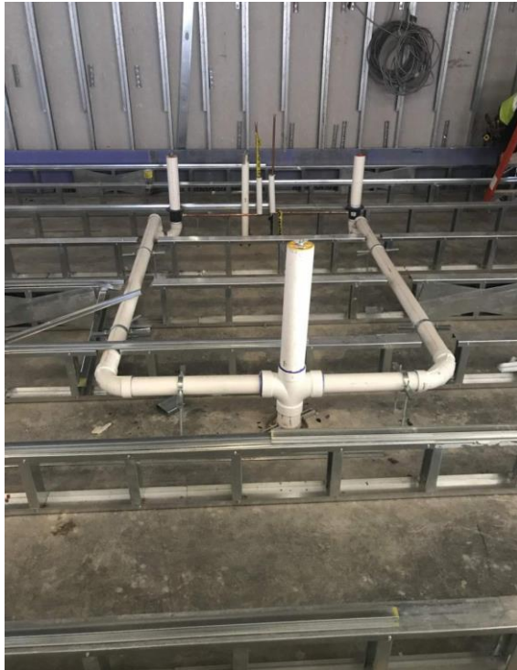
PLUMBING ROUGH-INS AT STUDENT BATHROOM ON 1 ST FLOOR
