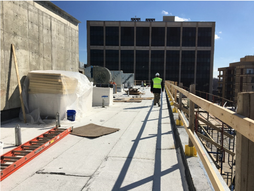
Final roofing installed at level 5
