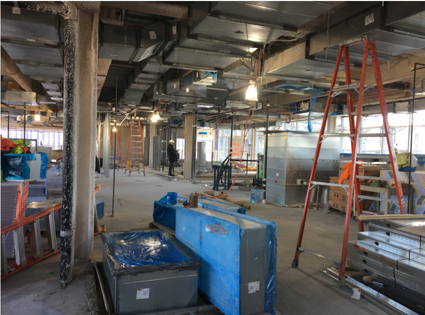
Mechanical duct work installed at L5
