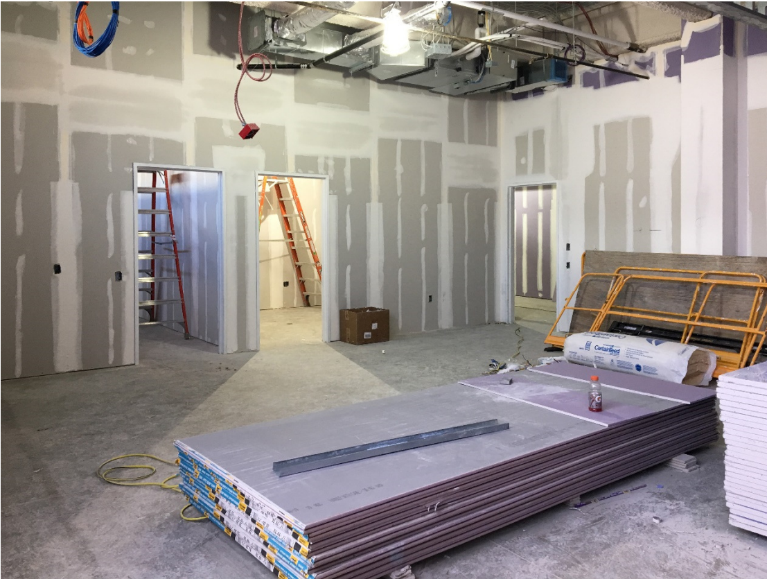
Front office at N. Quinn St entrance
