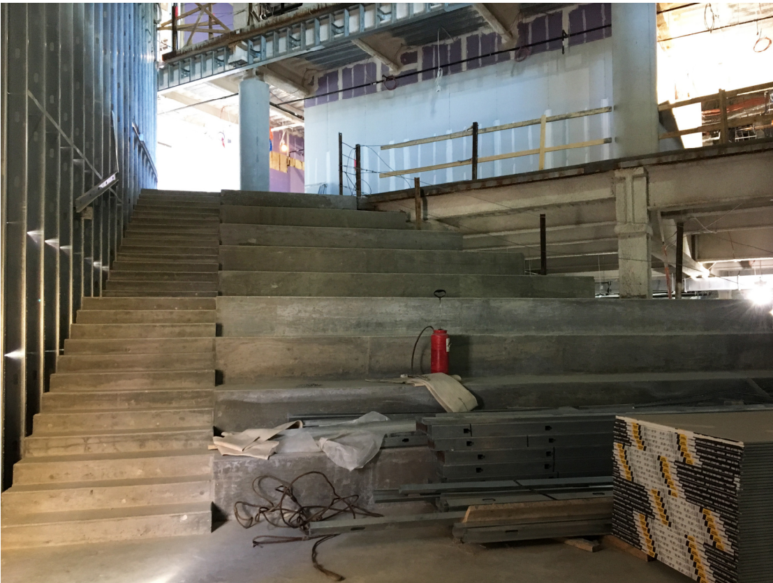
Concrete stair at Wilson Blvd. lobby up to library
