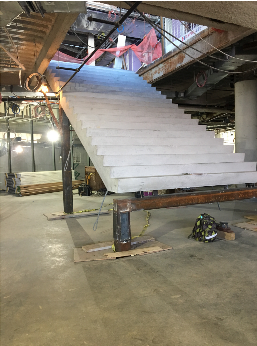
Interior cascading stair installed
