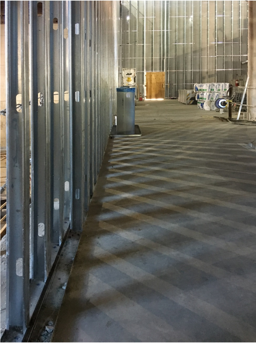
Framing for theater at Wilson Blvd. lobby
