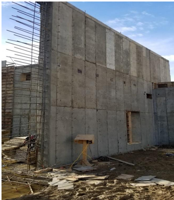
Auxiliary Gym foundation (after)
