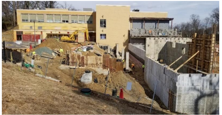
L1/L2 Foundation wall (after)
