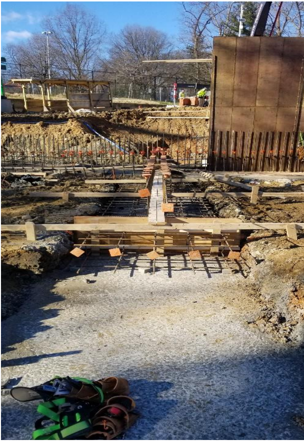
Auxiliary Gym foundation (before)
