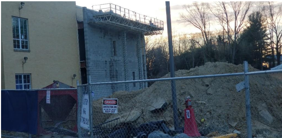
New 12-inch Firewall between existing and addition, (after)
