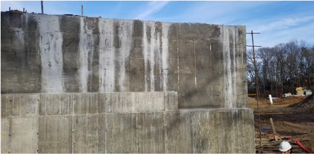
Exterior of Aux Gym Walls to receive brick fascia
