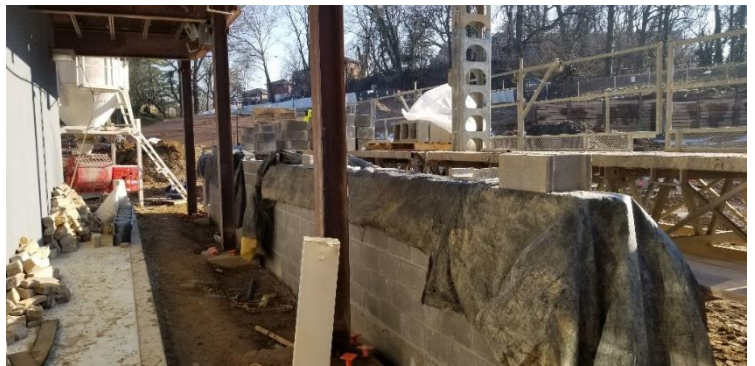
New 12-inch Firewall between existing and addition, (during)
