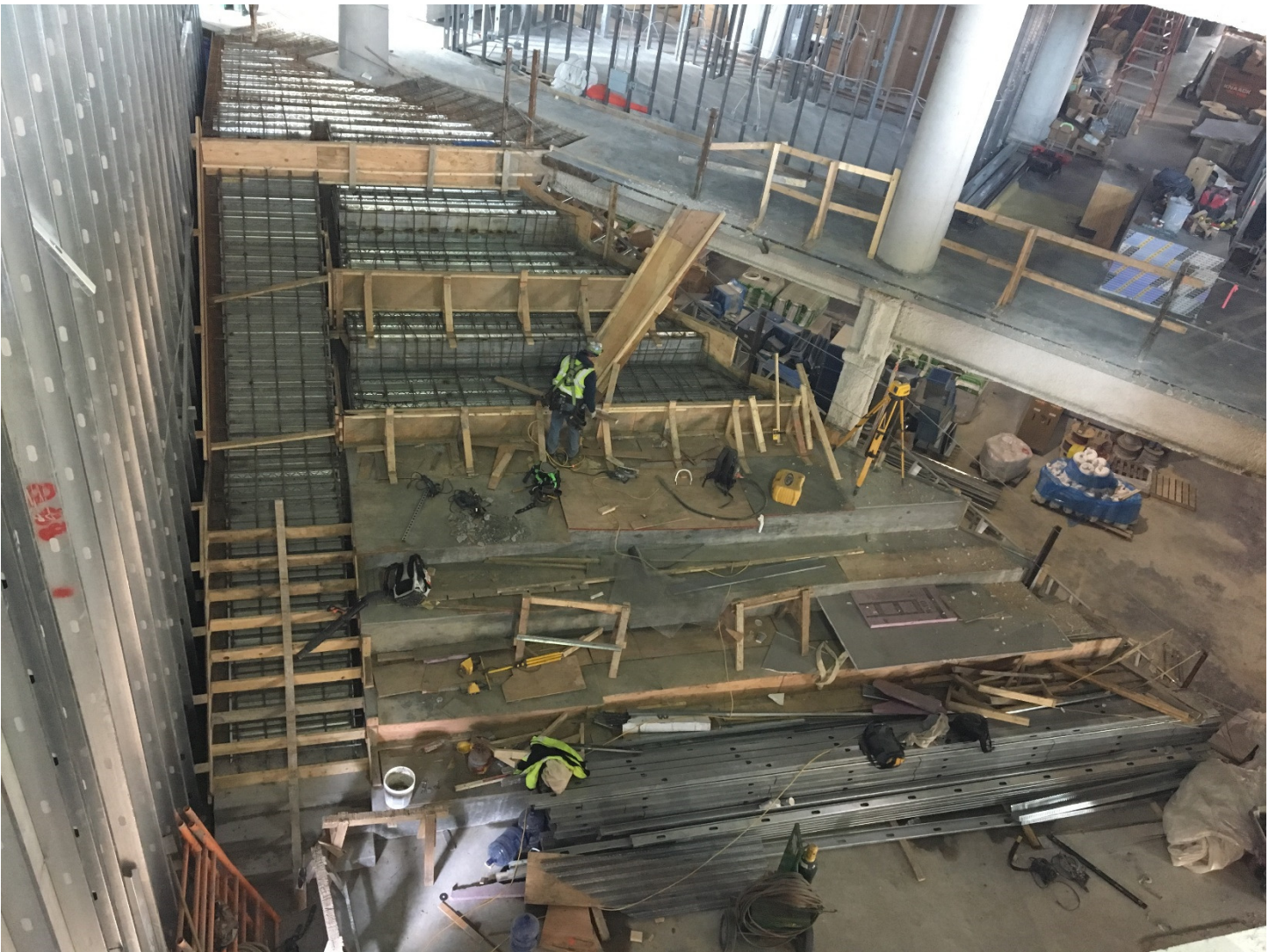
Formwork for stair at Wilson Blvd entrance for concrete pour
