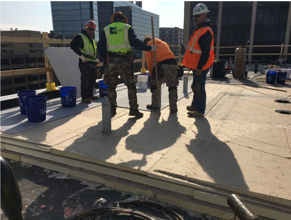
Roof and insulation installed at L5
