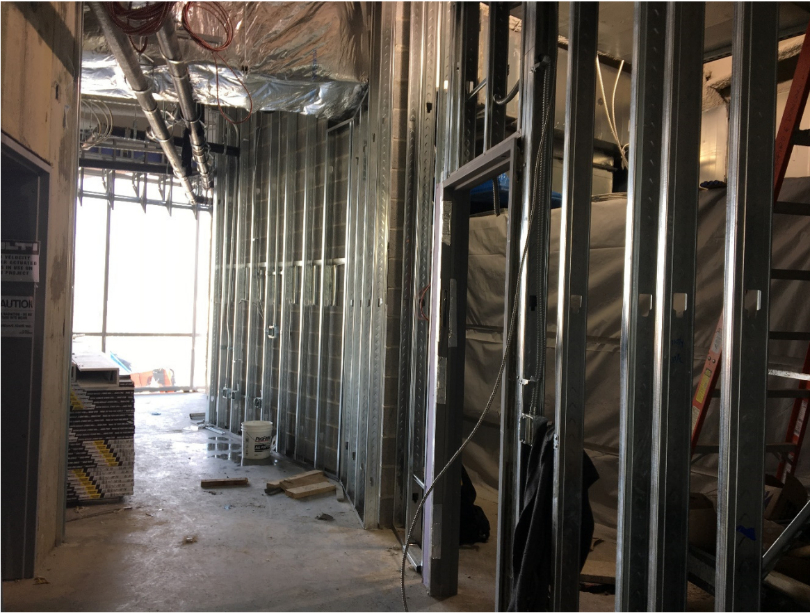
CMU wall at L2 mechanical room
