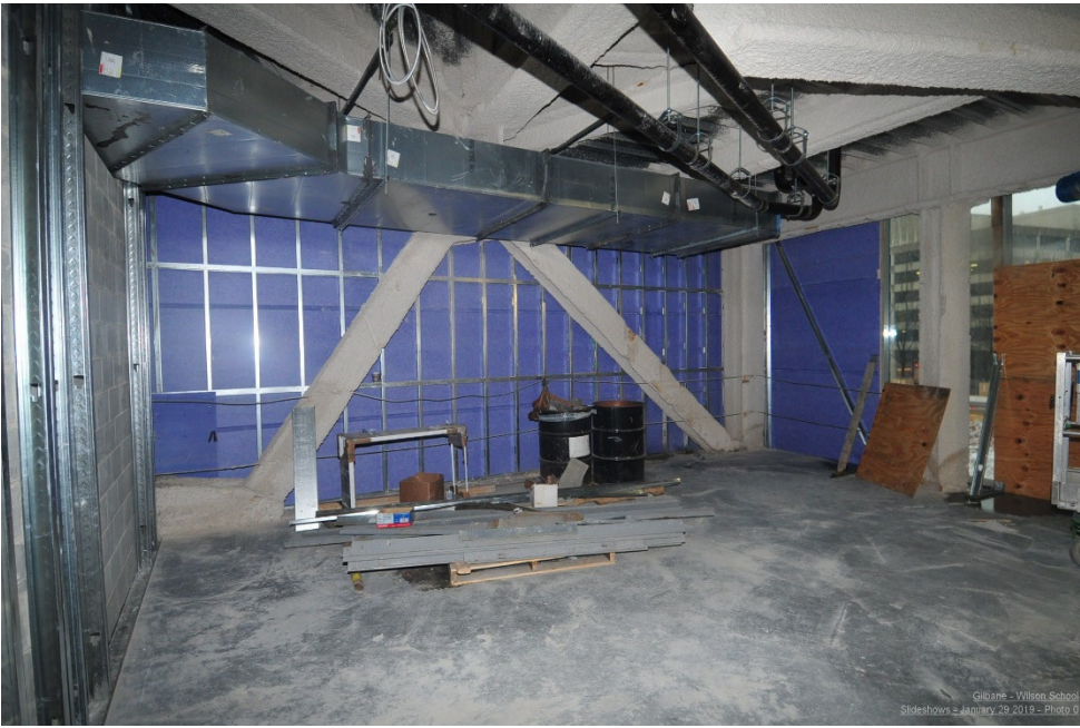
Framing at L2 exterior wall
