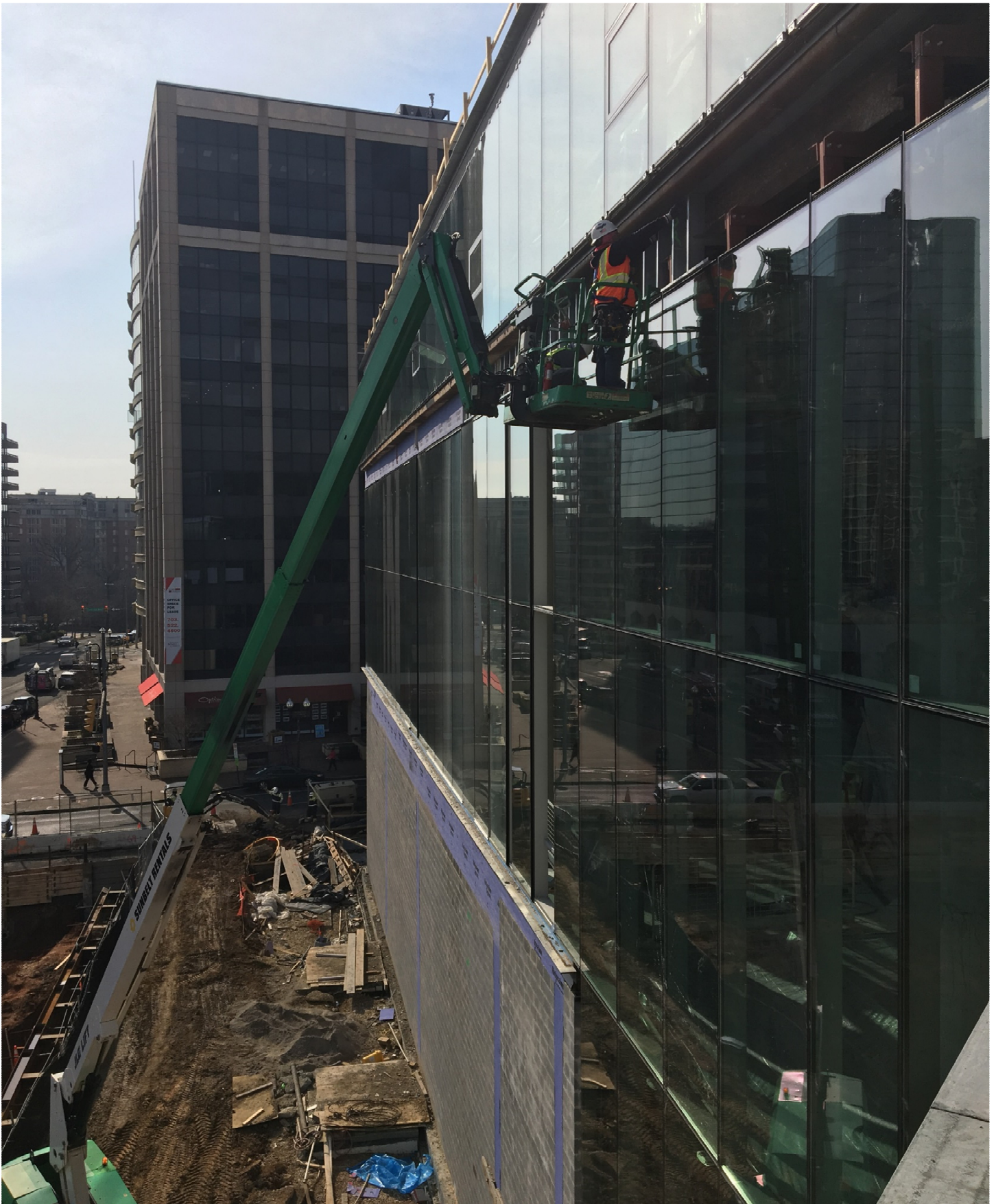
Install exterior framing
