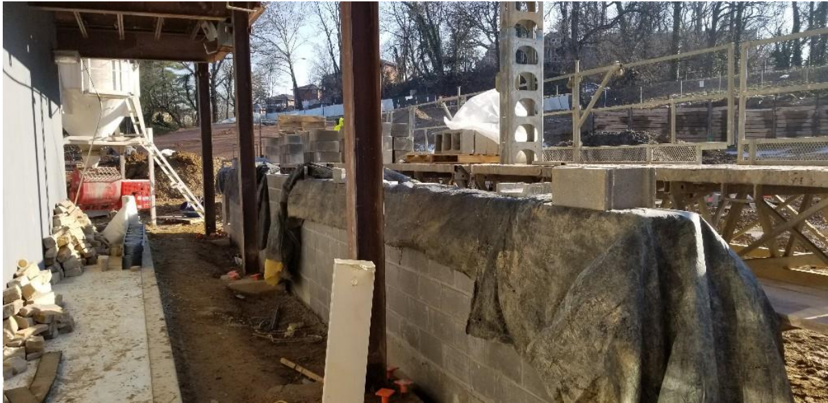
New 12-inch Firewall between existing and addition
