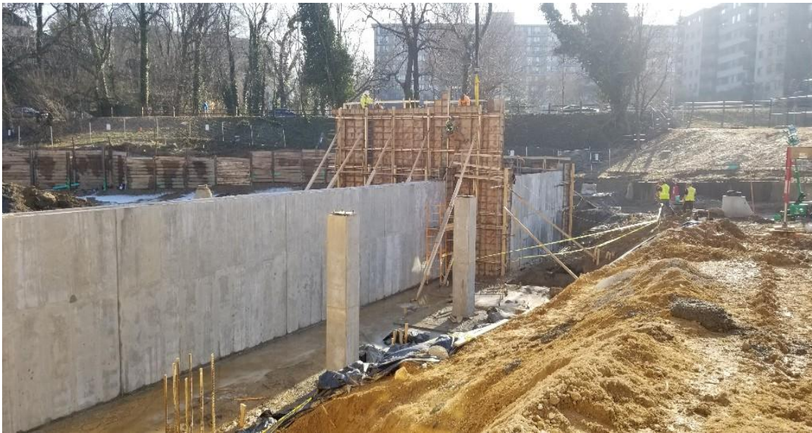
Level 1 / Level 2 Retaining Wall
