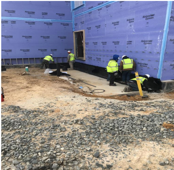
FINAL STAGES OF FOUNDATION WATERPROOFING
