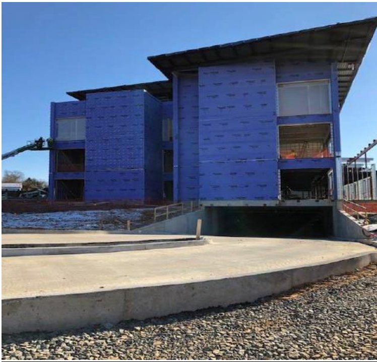
FAÇADE AT NORTH SIDE AND GARAGE ENTRY RAMP
