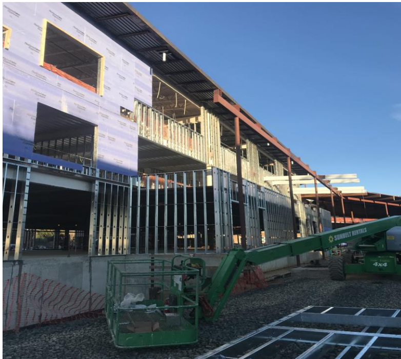
EXTERIOR FRAMING AND SHEATHING AT WEST FACADE
