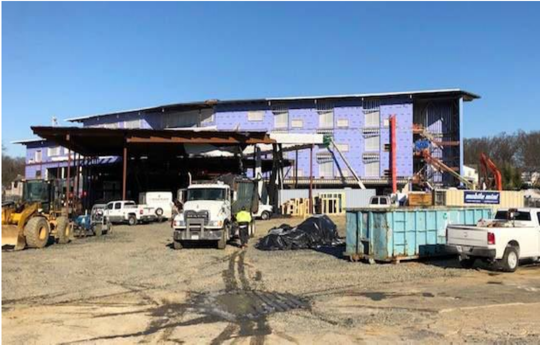
SOUTH FAÇADE PROGRESS
