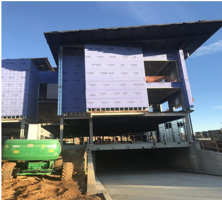
GARAGE ENTRY AND RAMP
