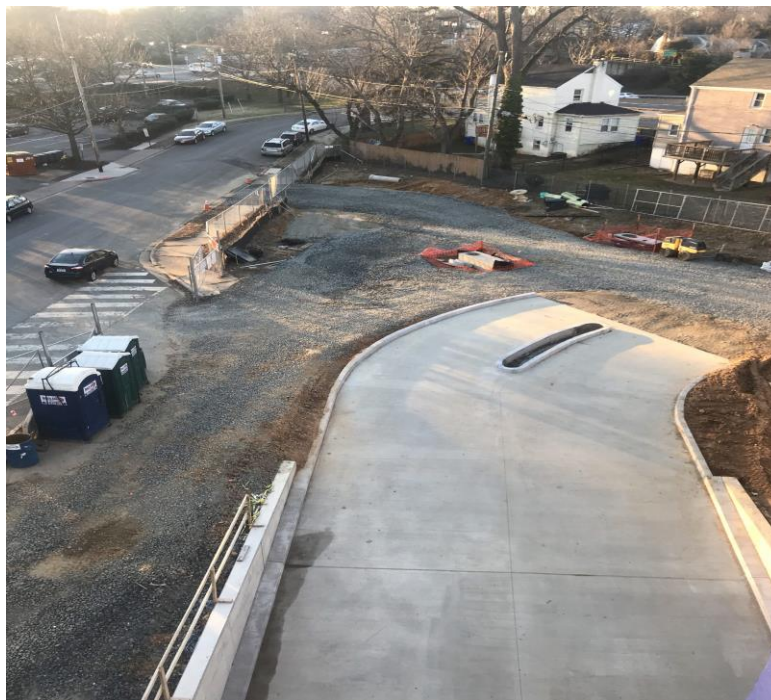
GARAGE CONCRETE RAMP TIED INTO BUS LOOP STONE SUB-BASE
