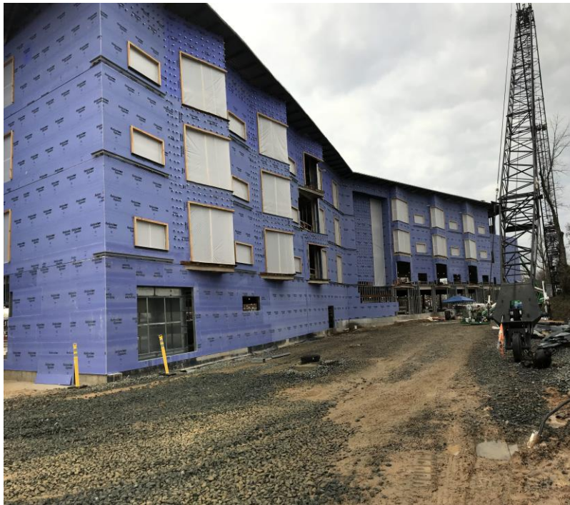
NORTH SIDE FAÇADE EXTERIOR FRAMING AND SHEATHING
