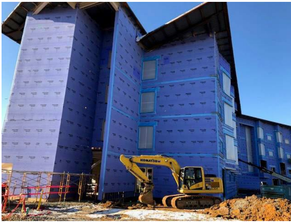
EAST SIDE FAÇADE EXTERIOR SHEATHING COMPLETE
