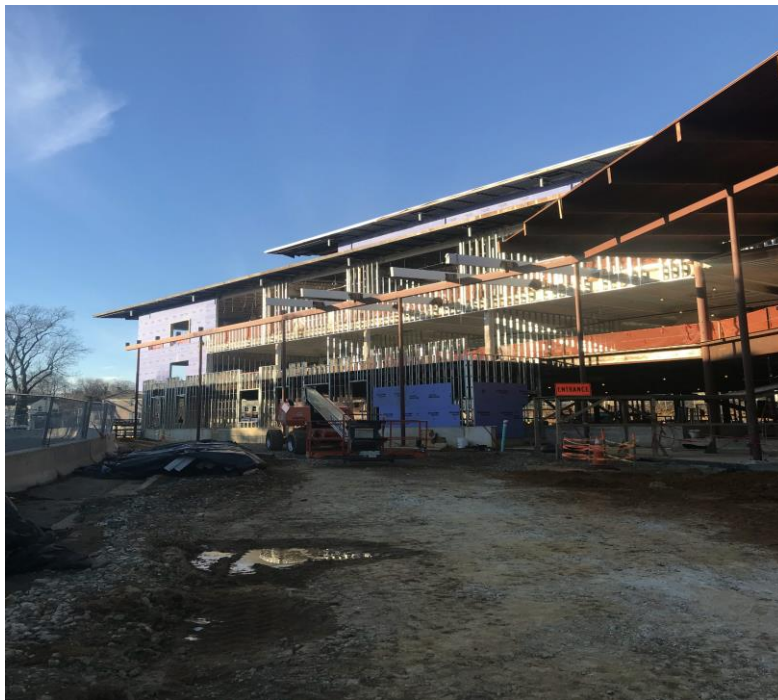
EXTERIOR FRAMING AT WEST FAÇADE
