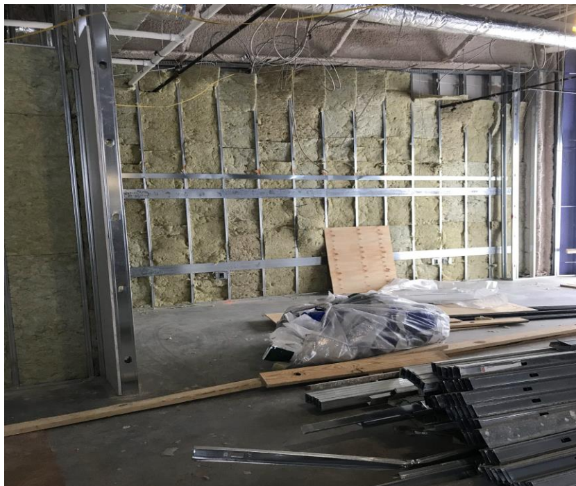
INTERIOR PARTITION WALL SOUND INSULATION
