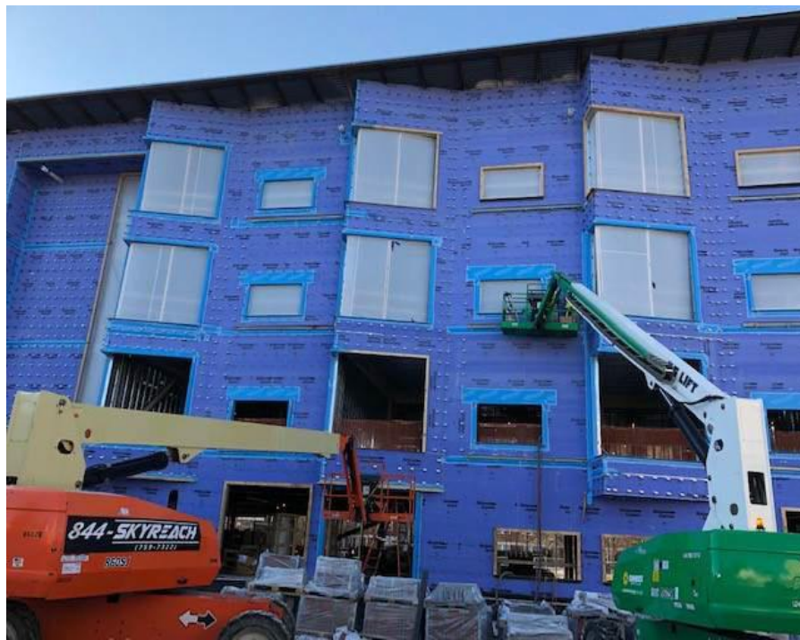
INSTALLATION OF BLUESKIN AIR/VAPOR BARRIER TRANSITION STRIPS AT WINDOWS
