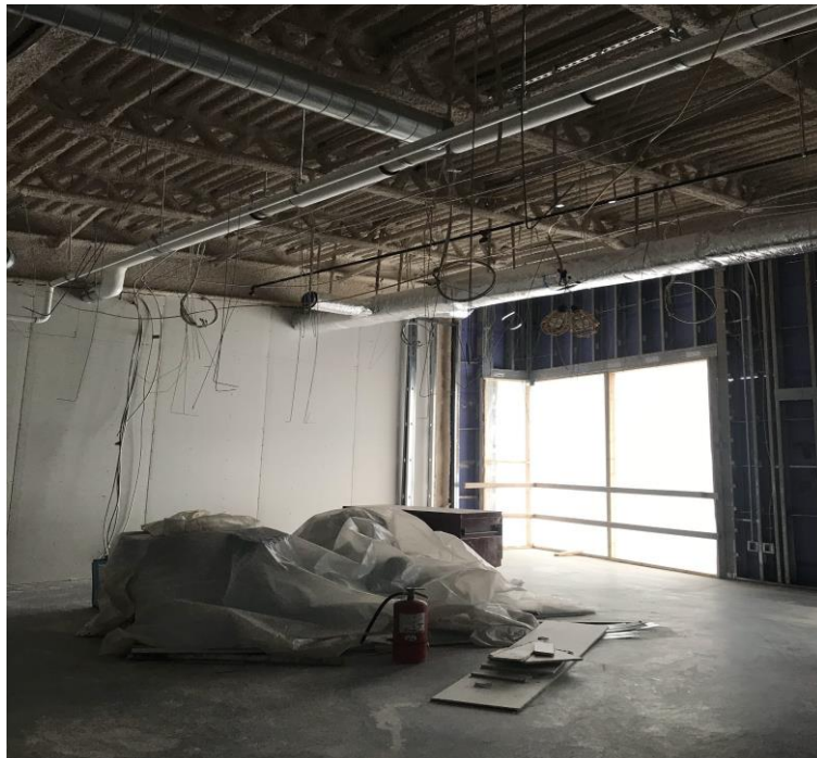
ONGOING MEP ROUGH-IN WORK
