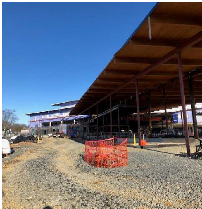
WEST SIDE FAÇADE IN FRONT OF GYM
