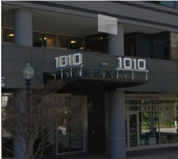
VIEW OF CANOPY
